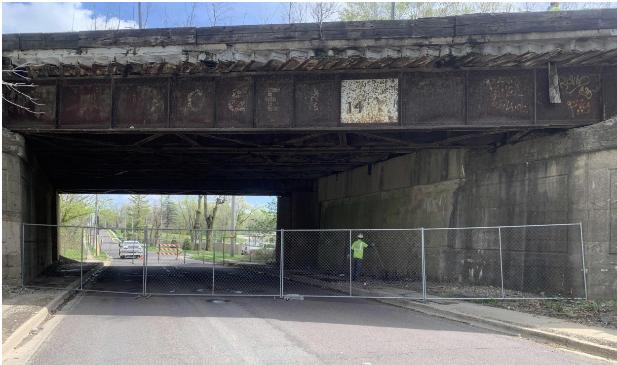
FIGURE 4-8: CLOSED ROADWAY UNDERPASS WHILE RAIL BRIDGE REPAIRS ARE COMPLETED
