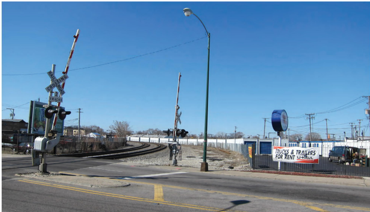
FIGURE 4-7: CENTRAL AVENUE/BELT RAILWAY COMPANY OF CHICAGO CROSSING
