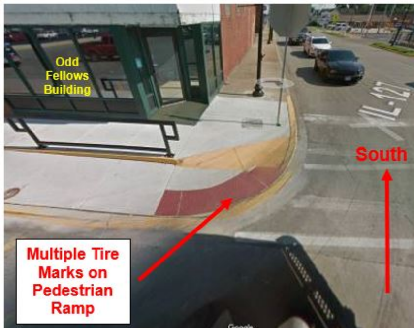
Figure 4 – Tire Tracks on Pedestrian Ramp
