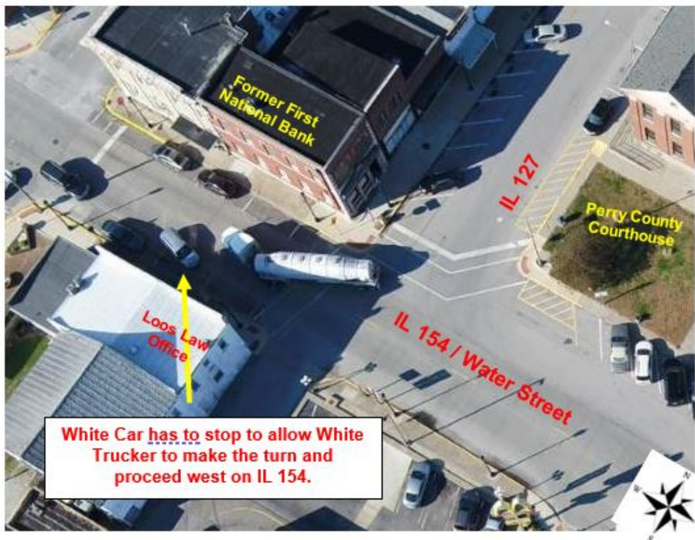
Figure 14 – Tanker Truck – Eastbound Lane Encroachment – IL 154
