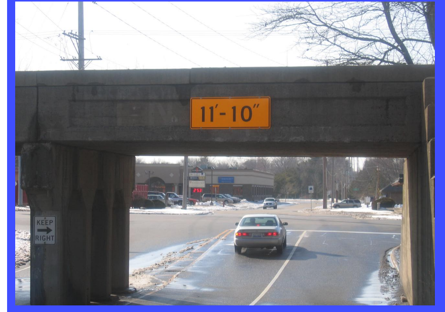
Figure 24: Clearance Constraint
