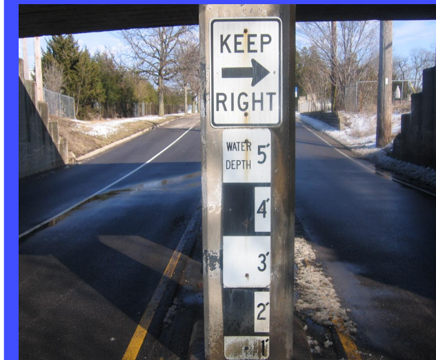
Figure 26: Water Depth Chart Under Viaduct
