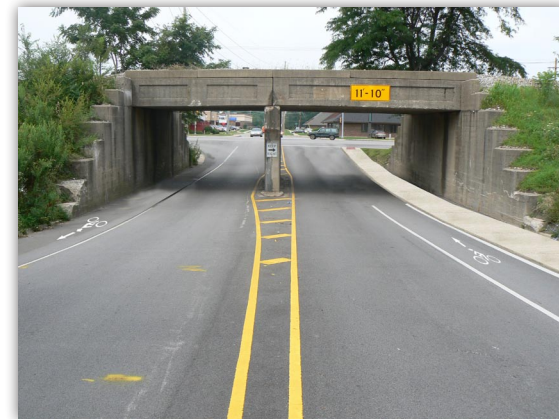
Looking west along St. Mary’s Road under viaduct: Horizon Year 2015
