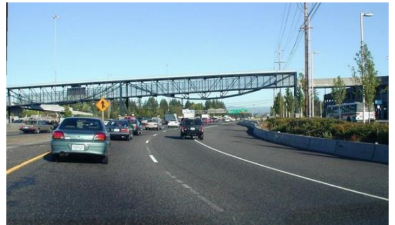
Light rail stations
