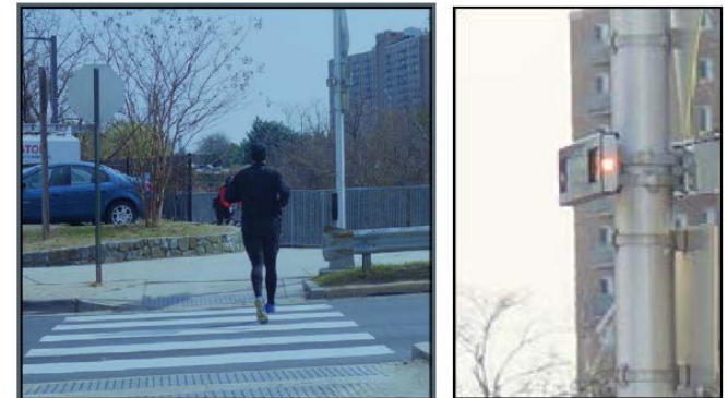
Figure 2. View of pilot light to pedestrian at shared-use path crossing with median refuge. Enlargement of pilot light at right.
