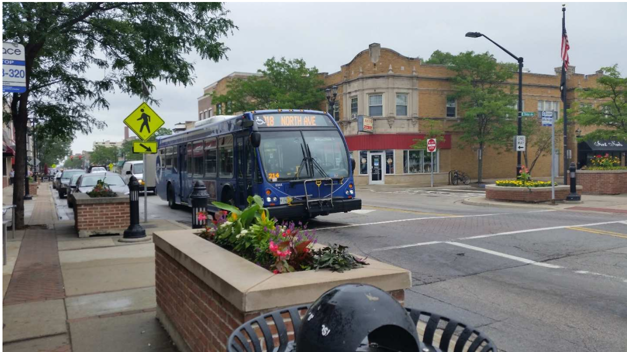
Figure 19 - Raised crosswalk on Madison Street in Forest Park, Illinois
