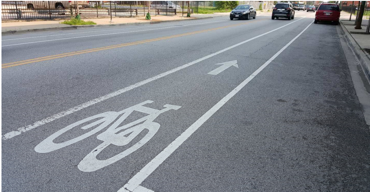
Figure 1 - Conventional bicycle lane on Damen Avenue in Chicago
