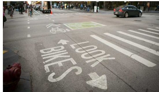
Figure 39 - Two-stage turn box between the SBL and the travel lanes on the two-way SBL on Dearborn Street in Chicago
