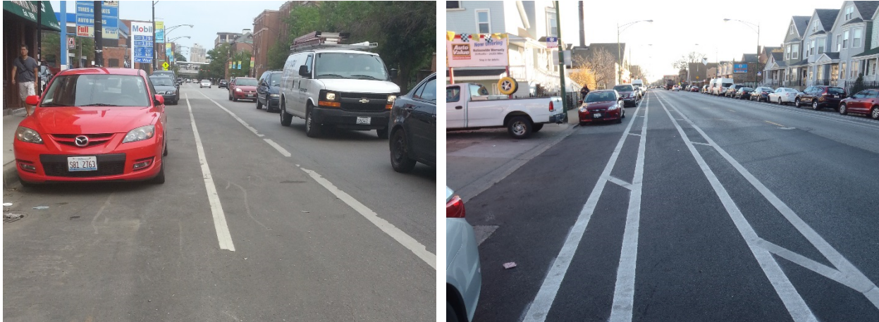
Figure 6 - Left: Fullerton Avenue conventional bicycle lane survey approach. Right: Kedzie Avenue buffered bicycle lane survey approach.
