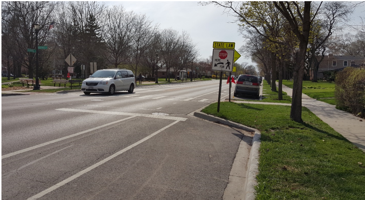
Figure 1 - Curb bump out extending into a parking lane on Central Street in Evanston, Illinois
