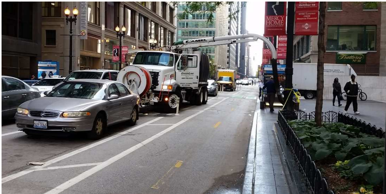
Figure 14 - CTA contractor cleaning out a subway station with hose boom extending over the Dearborn Street two-way separated bicycle lane in Chicago
