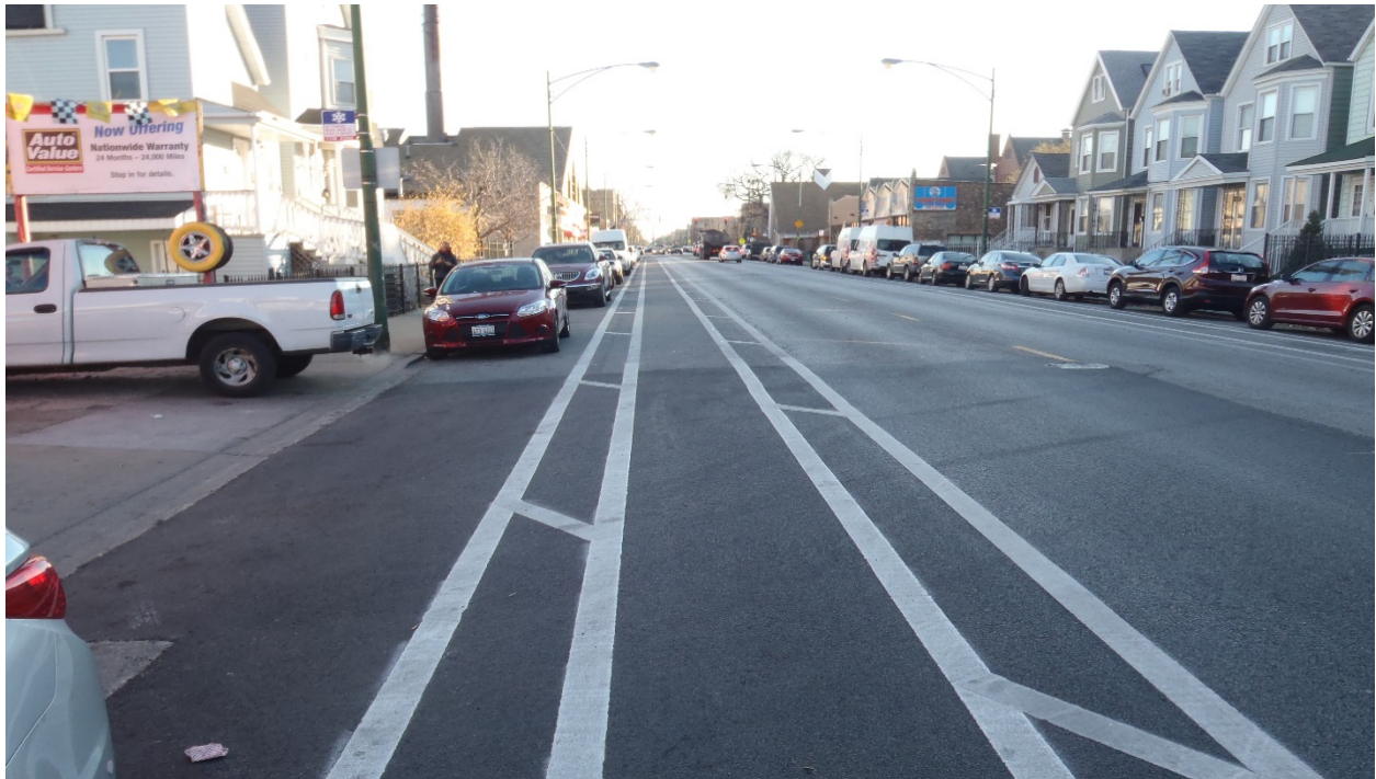
Figure 1 – Buffered bicycle lanes on Kedzie Avenue in Chicago
