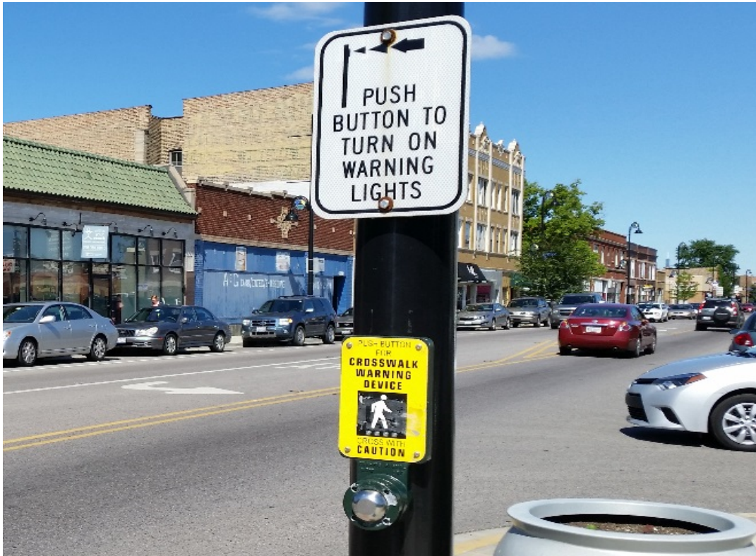
Figure 6 - Pedestrian activated button on Roosevelt Road (IDOT) at Lombard Avenue in Oak Park, Illinois. View is from south side of Roosevelt Road looking easterly.
