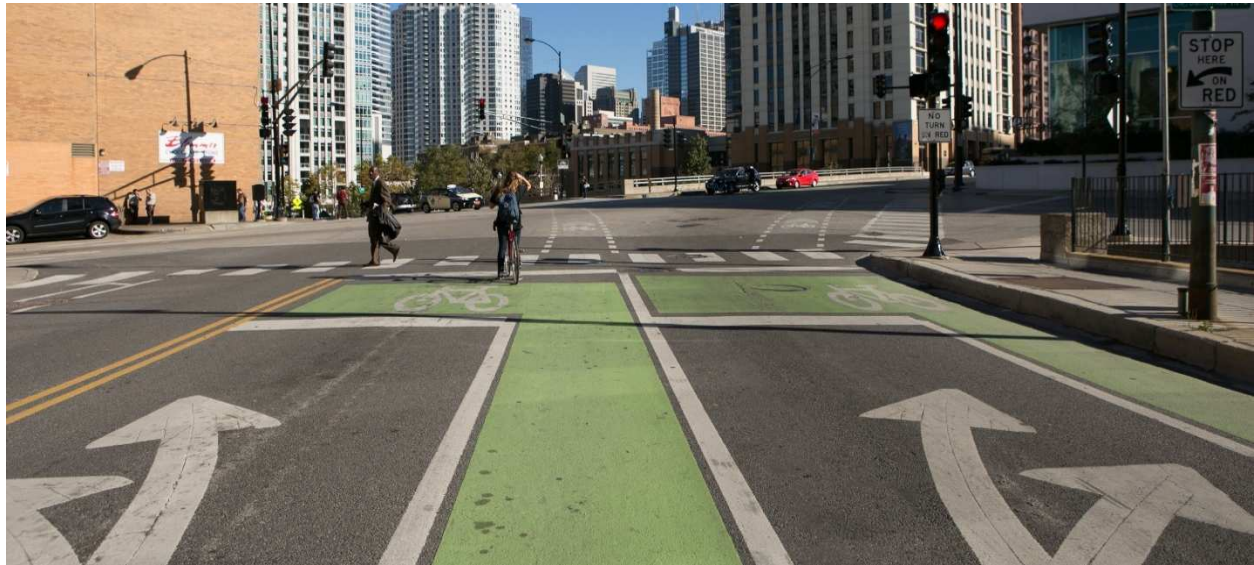
Figure 1 – Bicycle boxes at the head of both southbound traffic lanes along Milwaukee Avenue at the intersection with Desplaines Street and Kinzie Street in Chicago
