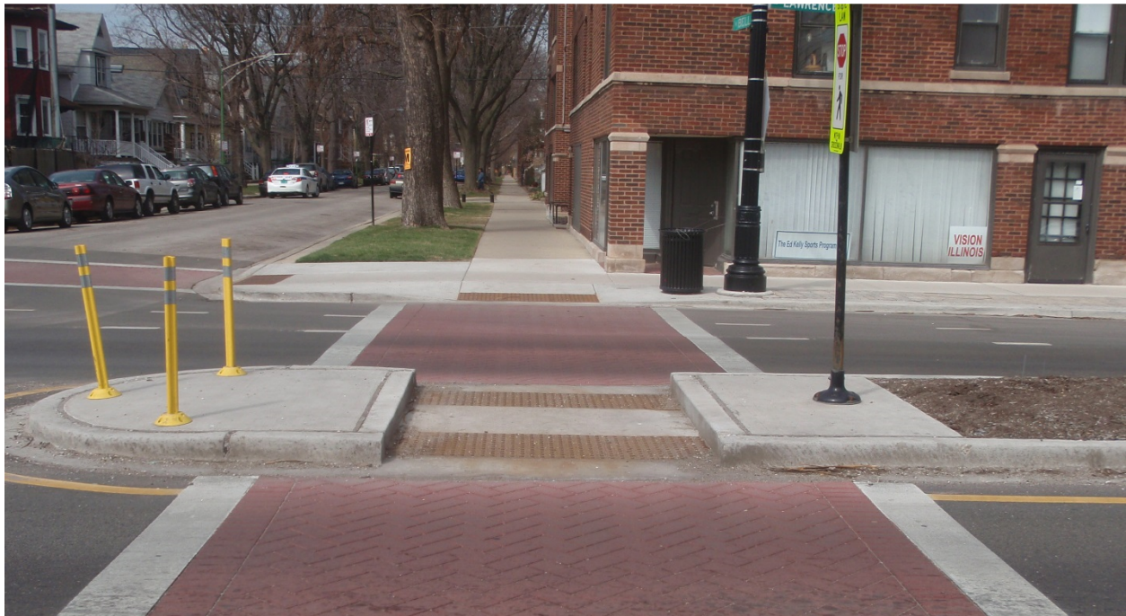
Figure 1 - Crosswalk enhancements utilizing alternative color and texture between crosswalk lines and supplemental unsignalized pedestrian crosswalk signs, on Lawrence Avenue in Chicago
