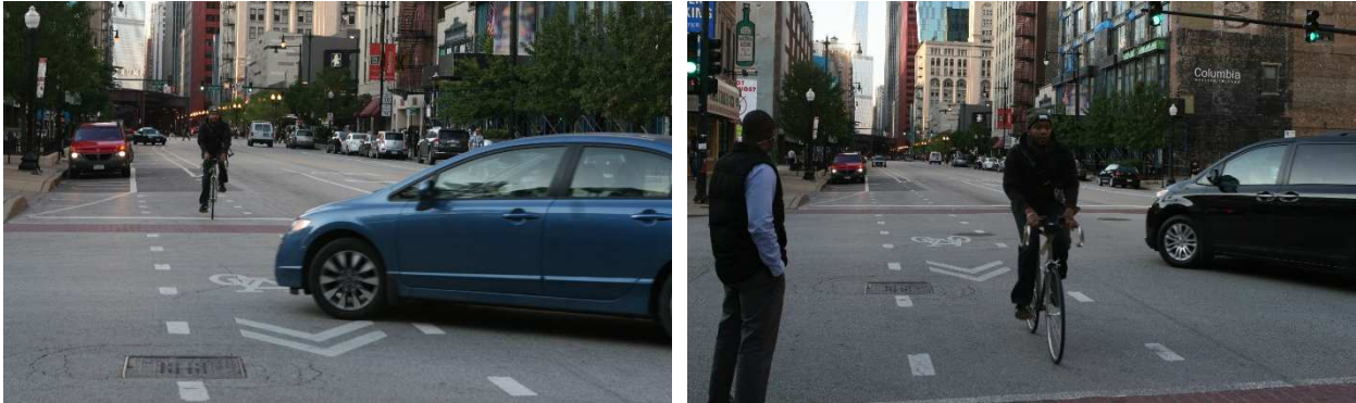
Figure 41 - Dotted stripe intersection marking with shared lane marking on the Wabash Street buffered bicycle lane in Chicago
