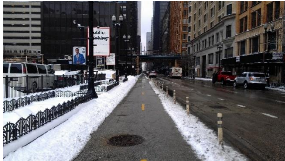
Figure 15 - Plowed and salted two-way separated bicycle lane in Chicago
