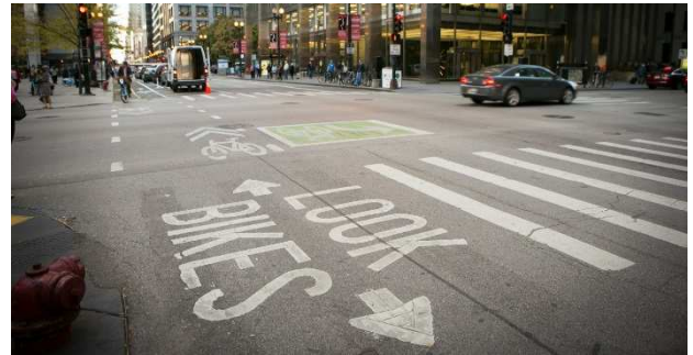
Figure 15 - Intersection crossing marking with dotted striping, shared lane markings, and pedestrian warnings inside the crosswalk on the Dearborn Street two-way separated bicycle lane in Chicago.
