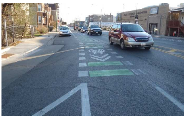
Figure 26 - Lateral shift with thick dotted striping, dotted colored pavement, and shared lane markings during the transition to an expressway onramp on Kedzie Avenue, Chicago
