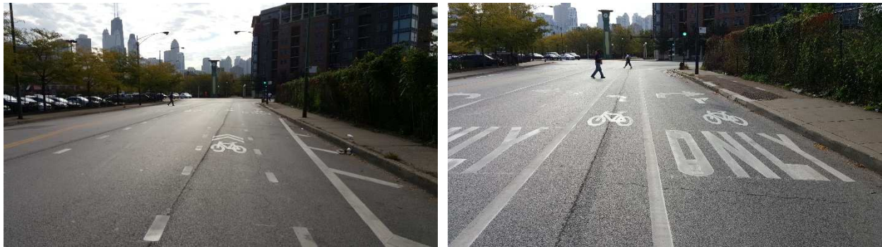
Figure 45 - Lateral shift on Clybourn Avenue at Division Street in Chicago.
