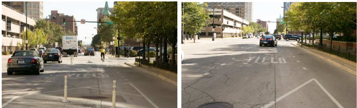
Figure 42 - Mixing zone with shared lane markings and yield markings on the Desplaines Street separated bicycle lane in Chicago
