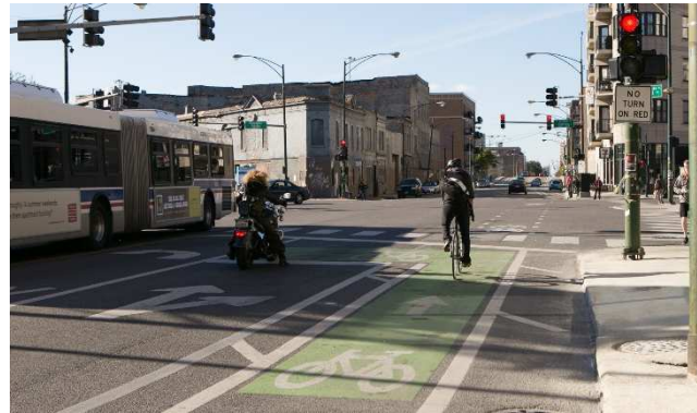
Figure 33 - Bicycle box on Milwaukee Avenue in Chicago
