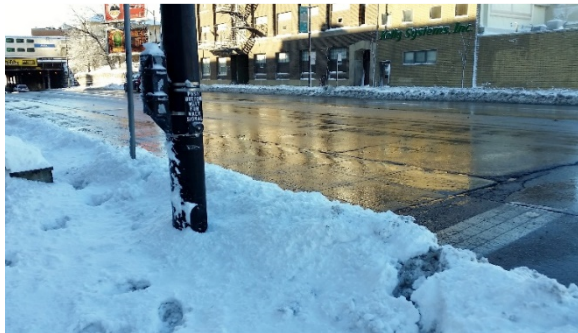
Figure 29 - Top: broken curb, brick, and road debris inside a median refuge island. Bottom: pedestrian push button and crosswalk ramp blocked by plowed snow.
