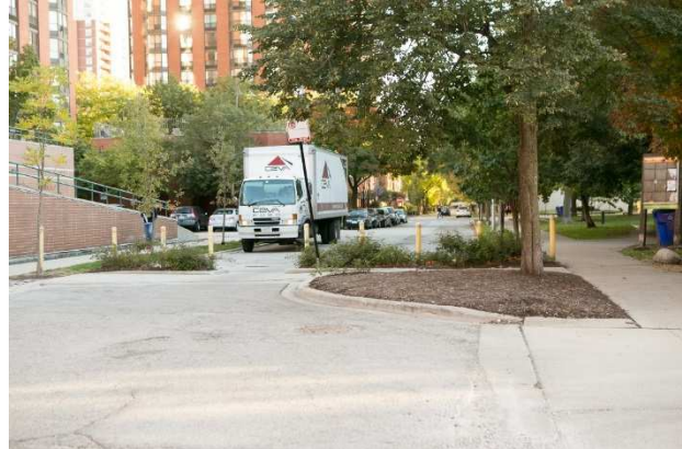
Figure 12 - Traffic diverter with landscaping in Chicago
