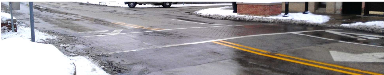
Figure 6 - Plowed and salted raised crosswalk on Madison Street in Forest Park. Note the shoveled sidewalk approaches.
