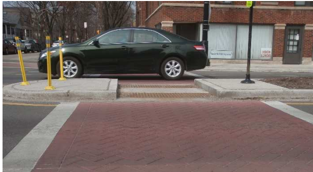
Figure 7 - Median refuge island with stamped pavement and an at-grade cut through for pedestrians on Lawrence Avenue in Chicago.
