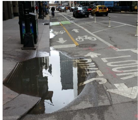
Figure 17 - Ponding on the Dearborn Street two-way separated bicycle lane in Chicago
