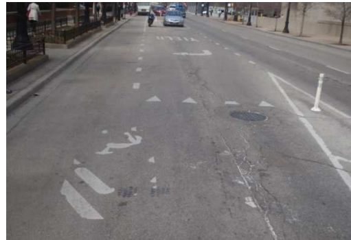
Figure 49 - Faded shared lane symbol and "sharks teeth" yield markings on a mixing zone on Desplaines Street in Chicago
