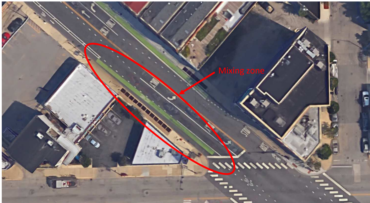
Figure 61 - Aerial view of Milwaukee Avenue and Chicago Avenue. Image: Google.
