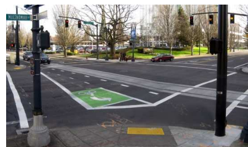
Figure 40 - Two stage turn box adjacent to a street-car route. Image from Urban Bikeway Design Guide, by NACTO. Copyright © 2014 National Association of City Transportation Officials. Reproduced by permission of Island Press, Washington, D.C.
