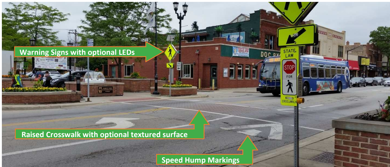
Figure 1 - Raised crosswalk on Madison Street in Forest Park, Illinois
