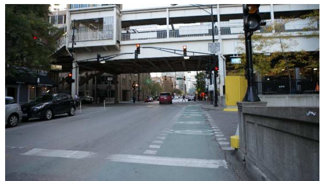
Figure 10 - Dotted and colored intersection marking with bicycle symbols orientated toward the cross traffic direction on Kinzie Street in Chicago.
