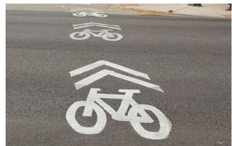
Figure 30 - Shared lane markings calling attention to a popular intersection crossing from the Lake Front Trail on Ardmore Avenue in Chicago
