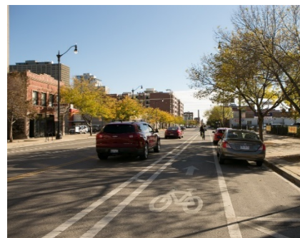
Figure 16 - Buffered bicycle lanes on Wabash Street in Chicago
