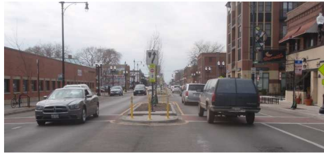
Figure 11 - Median refuge island on West Lawrence Avenue in Chicago
