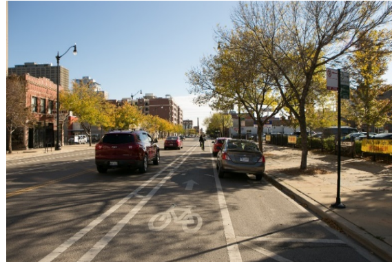
Figure 3 – Buffered bicycle lanes on Wabash Street in Chicago
