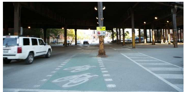
Figure 11 - Intersection crossing marking with dotted striping, colored pavement, and bicycle symbols orientated in the direction of approaching traffic. The crossing includes associated signage and is located on a separated bicycle lane on Kinzie Street in Chicago.
