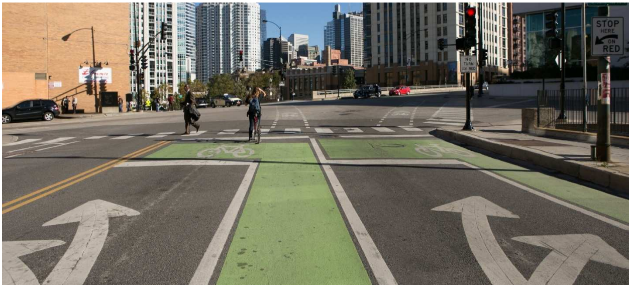
Figure 46 - Bicycle boxes at the head of both southbound traffic lanes along Milwaukee Avenue at the intersection with Desplaines Street and Kinzie Street in Chicago
