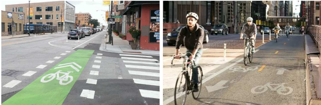
Figure 1 – Left: one-way SBL along Milwaukee Avenue in Chicago, utilizing flexible bollards and parking lane for separation from motorists. Right: two-way SBL along Dearborn Street in Chicago, separated by flexible bollards over the Chicago River.
