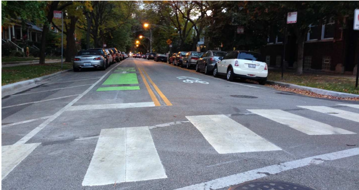
Figure 1 - Bicycle boulevard that includes a contra-flow bicycle lane in one direction and a marked shared lane in the other, on Berteau Avenue in Chicago
