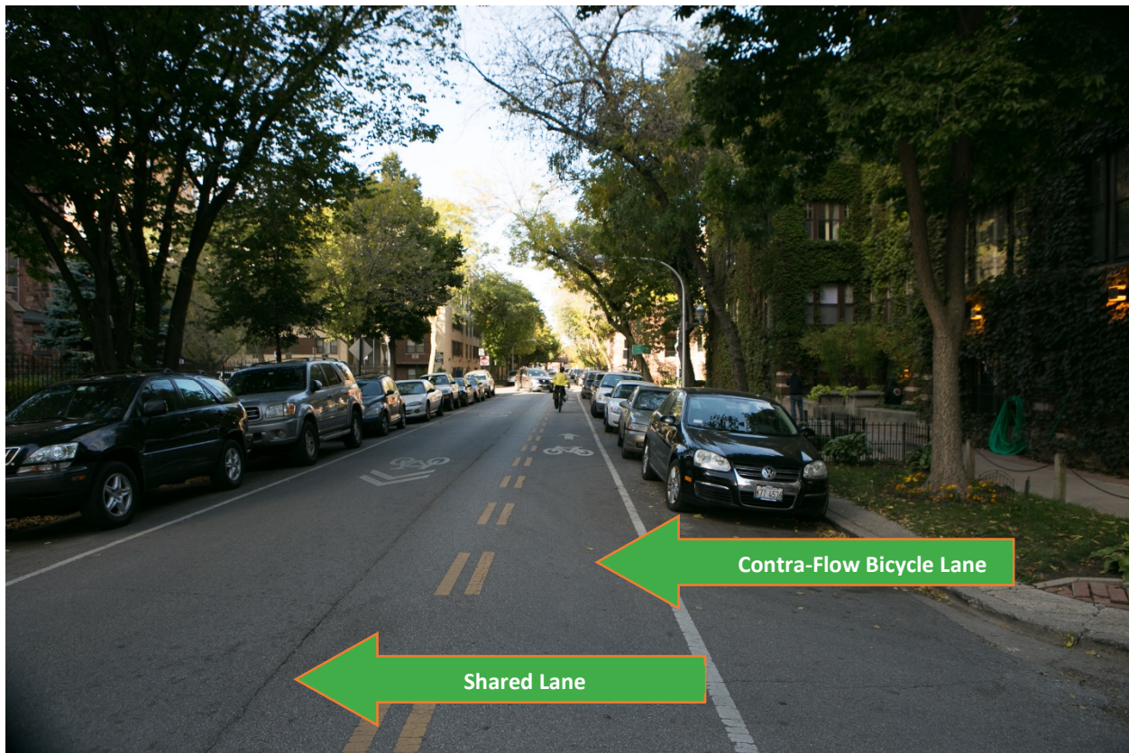
Figure 1 - Contra-flow bicycle lane along West Ardmore Avenue from Kenmore Avenue to Sheridan Road in Chicago. The bicycle lane is in the contra-flow direction separated from the opposing marked shared lane with a dashed double yellow line.
