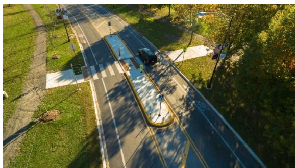
Figure 20 - Midblock crossing with median refuge island. Copyright Skyity.com. Reprinted with permission.
