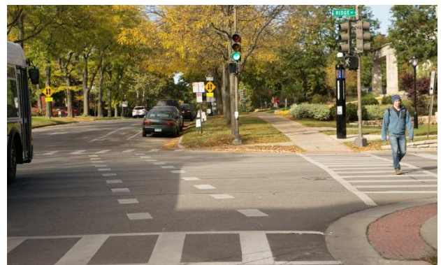
Figure 16 - Intersection crossing marking with "elephant feet" striping along the Church Street separated bicycle lane in Evanston. The markings help guide bicyclists at an offset intersection. See the section on Lateral Shifts below for more information on various striping options.
