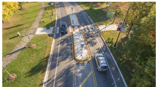
Figure 4 – Median refuge islands on two separate road diet conversions in Chicago. Bottom image reprinted with permission by Skyity.com.
