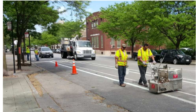
Figure 7 - Striping crew on Washington Street in Chicago
