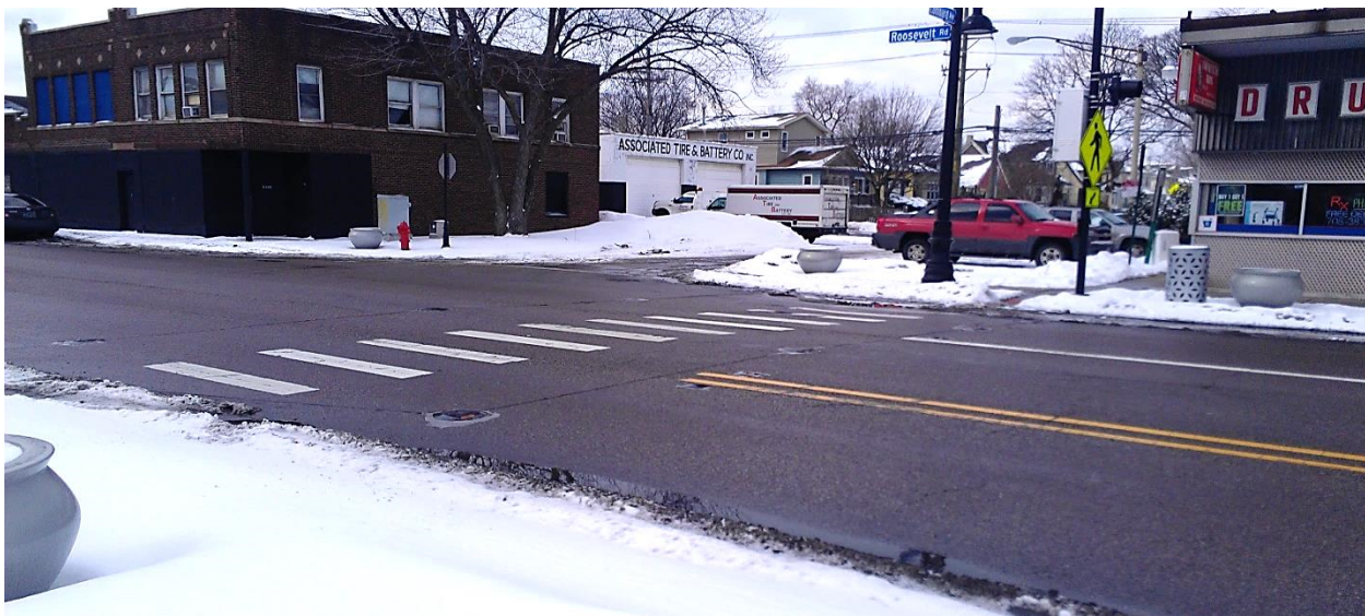
Figure 3 - A lighted crosswalk in the winter on Roosevelt Road (IDOT) at Lombard Avenue in Oak Park, Illinois. View is from the south side of Roosevelt Road looking northwesterly.
