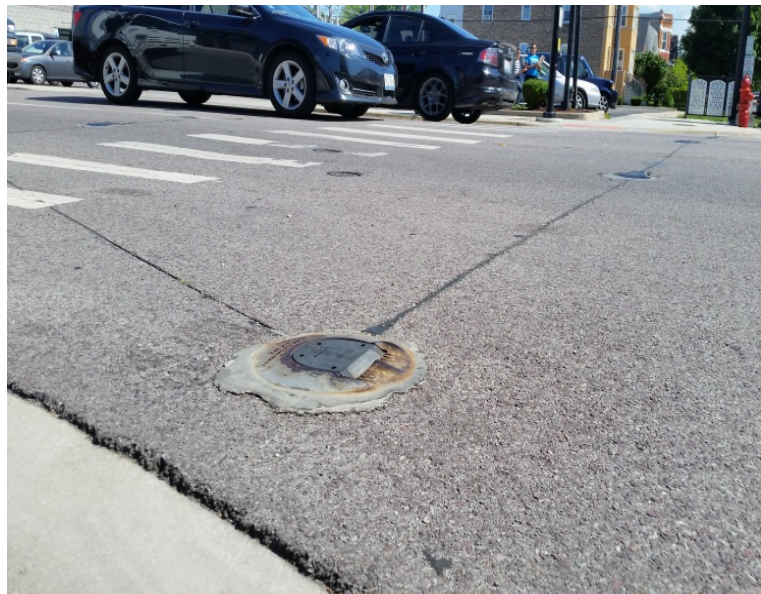
Figure 32- In-roadway warning lights on Roosevelt Road at Lombard Avenue intersection in Oak Park, Illinois
