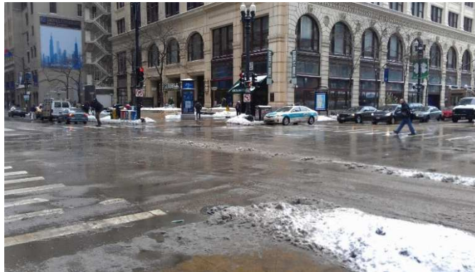
Figure 15 - Partially snow-covered crosswalks at the Barnes Dance at State Street and Jackson Boulevard in Chicago. The diagonal crosswalk markings have worn out and are not noticeable in the photo.
