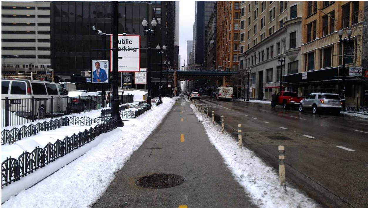
Figure 11 - Plowed and salted two-way separated bicycle lane along Dearborn Street in Chicago
