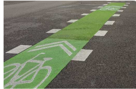
Figure 31 - Green colored pavement, with shared lane markings and dotted white lines, delineating an SBL intersection crossing marking on Davis Street in Evanston, IL
