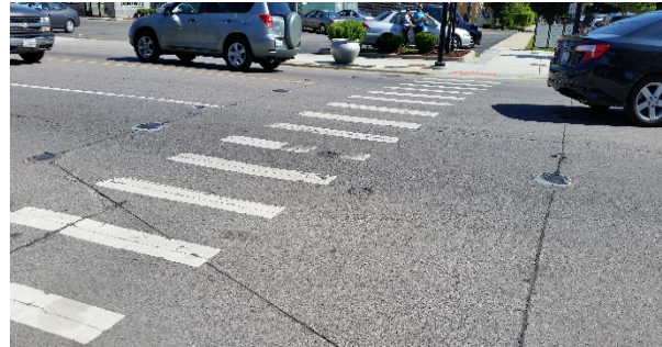
Figure 10 - IRWLs and cable routing on Roosevelt Road (IDOT) at Lombard Avenue in Oak Park, Illinois
