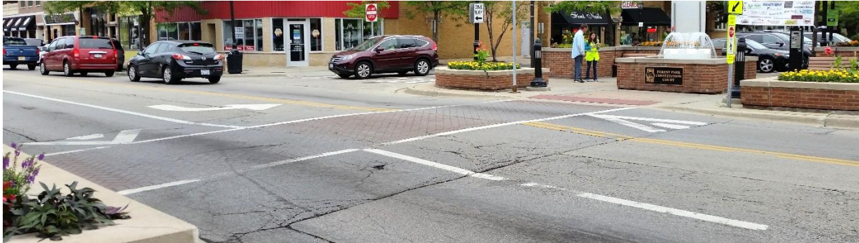
Figure 5 - Raised crosswalk on Madison Street in Forest Park, Illinois
