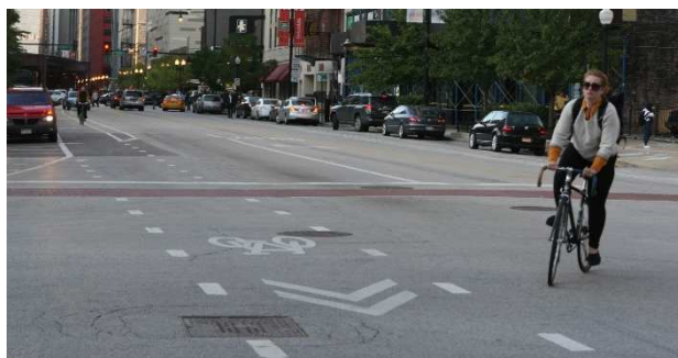
Figure 9 - Intersection marking with shared lane marking on the Wabash Street buffered bicycle lane in Chicago.
