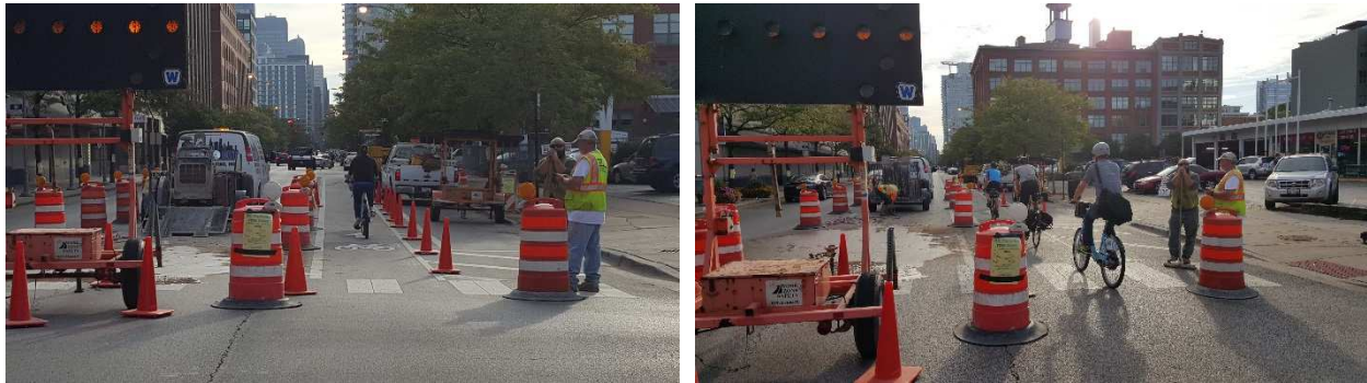
Figure 15 – Example of maintenance of traffic that leaves an adjacent buffered bicycle lane open in Chicago
