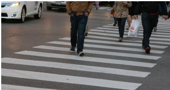
Figure 19 - International style crosswalk markings
