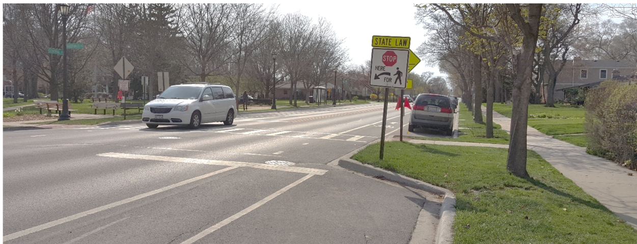
Figure 15 - Bump out at Central Street and Hastings Avenue in Evanston, Illinois
