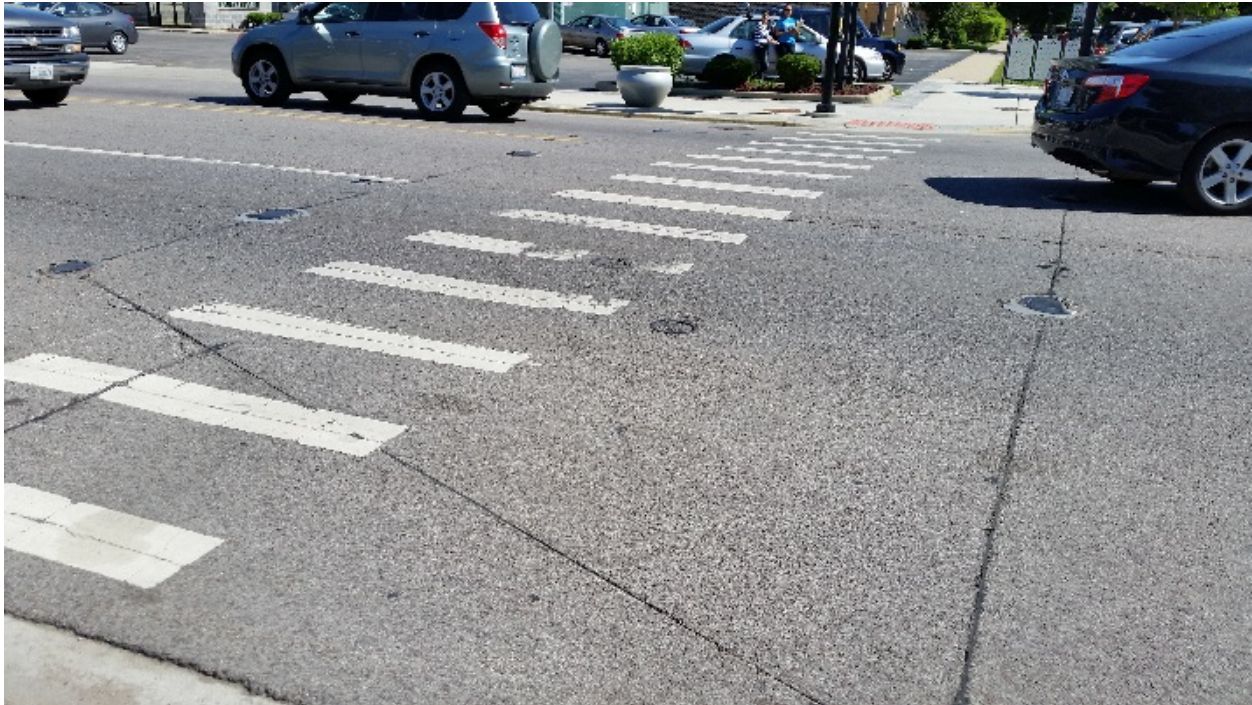
Figure 9 – Crosswalk with in-roadway warning lights on Roosevelt Road (IDOT) at Lombard Avenue in Oak Park, Illinois. View is from the south side of Roosevelt Road looking northerly.
