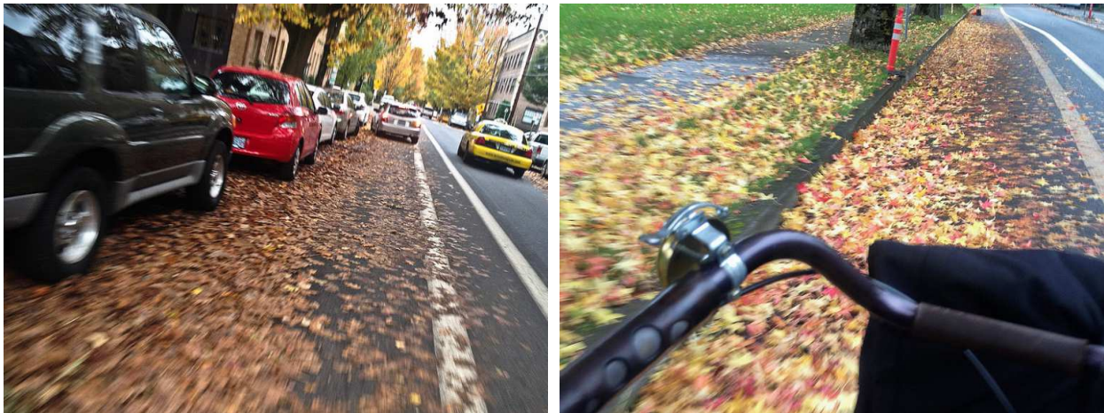
Figure 7 – Debris in left-side bicycle lanes on NW Everett Street in Portland, Oregon (Images: Jonathon Maus - Publisher/Editor, Bike Portland)
