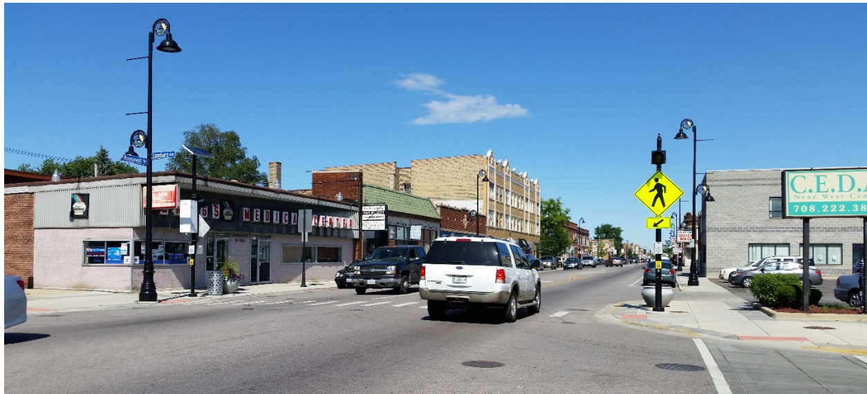
Figure 1— Lighted crosswalk with pedestrian warning beacon on Roosevelt Road (IDOT) at Lombard Avenue in Oak Park, Illinois. View is from south side of Roosevelt Road looking easterly.
