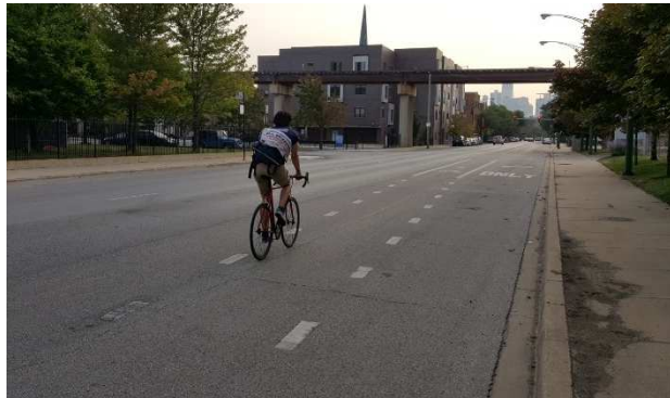
Figure 23 - Skip-dash striping lateral shift in Chicago. The bicycle lane is tapered out into the street to allow room for a turn lane and parking up ahead.
