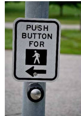
Figure 7 - Pushbutton detector at a HAWK signal in Pekin, Illinois
