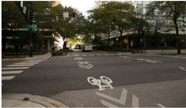
Figure 12 - Shared lane marking intersection crossings along Ardmore Avenue in Chicago
