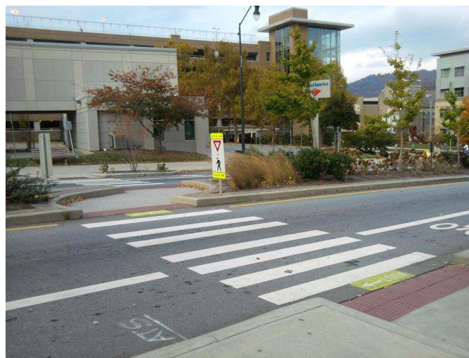
Figure 9 - Midblock median refuge island with an offset median cut through and accessible detector pads perpendicular to the roadway. Image: www.pedbikeimages.com / Lyubov Zuyeva
