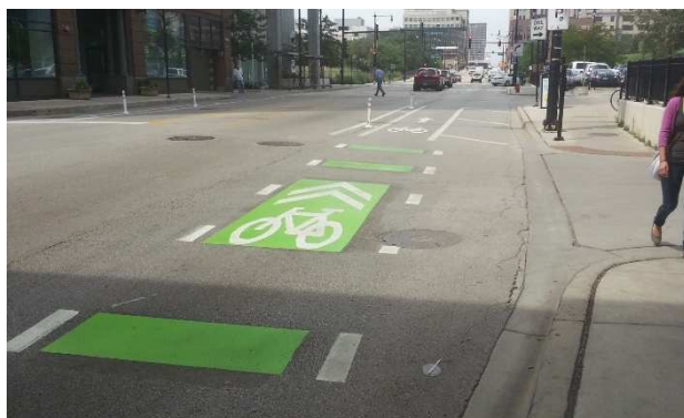
Figure 8 – Driveway/alley intersection marking with shared lane marking and green pavement on Harrison Street in Chicago.
