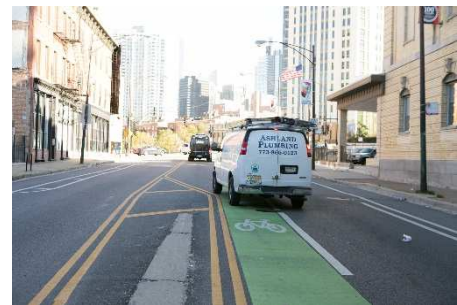
Figure 32 - Green pavement on the approach to a bicycle box at Desplaines Street and Milwaukee Avenue in Chicago
