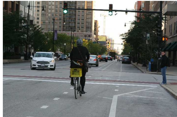
Figure 5 - Bicycle lanes and dedicated left turn lanes at an intersection on the Wabash Street road diet in Chicago
