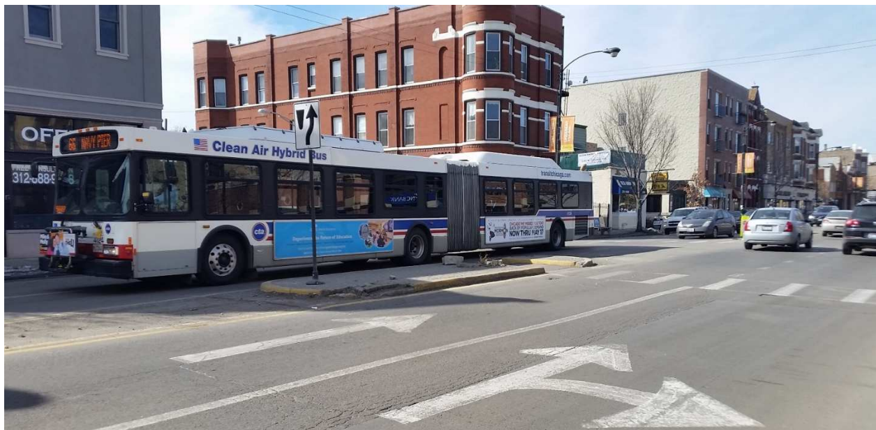
Figure 15 - Damaged median refuge island on Chicago Avenue and Hoyne Avenue in Chicago. All flexible delineators have been knocked down.
