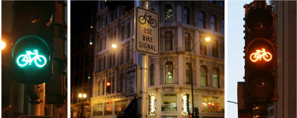
Figure 4 - Bicycle signal heads and signage for bicyclists and crossing pedestrians
