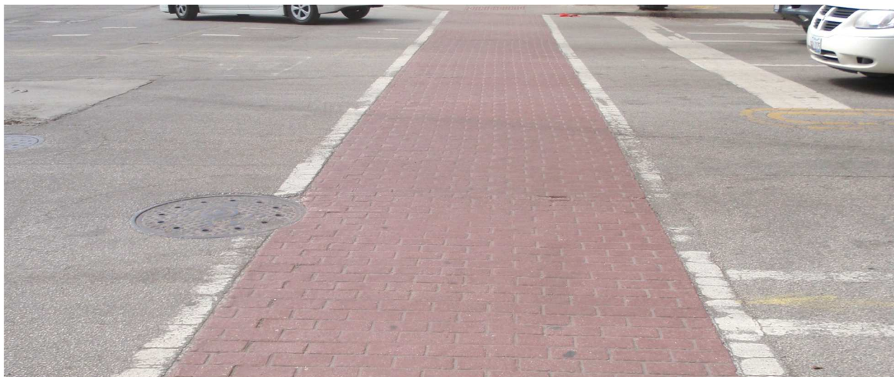
Figure 1 – Crosswalk enhancements utilizing alternative color and texture between crosswalk lines, at the intersection of Wabash and Roosevelt in Chicago, Illinois.
