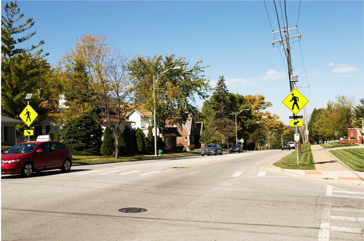
Figure 9 - RRFB at crossing in Lemont, Illinois
