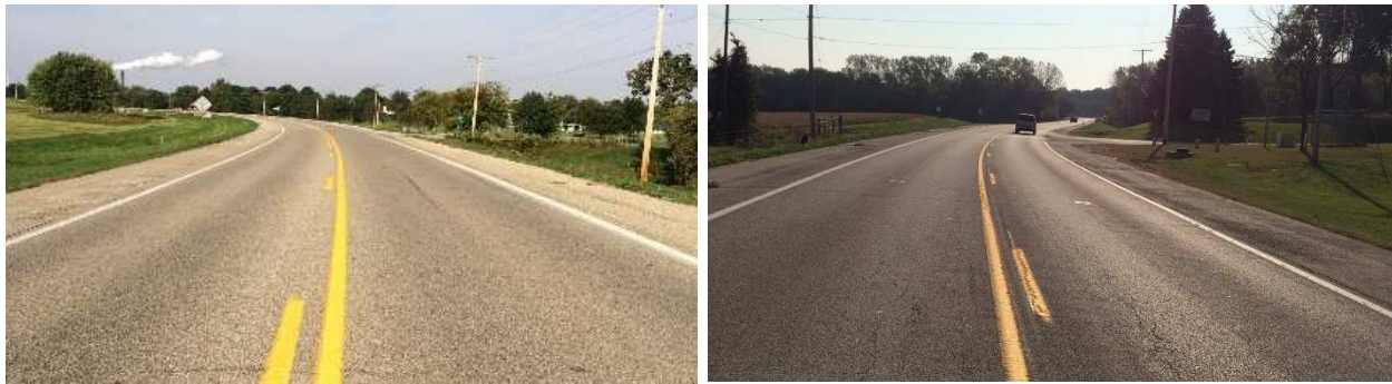
Figure 1 – Widened shoulders along County Highway 56 (Rochester Road) in Springfield, Illinois
