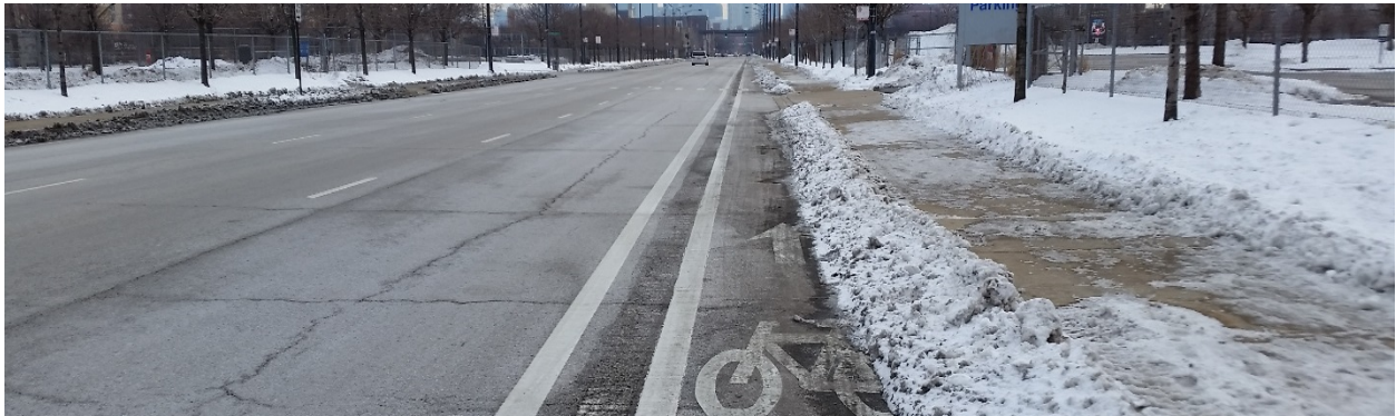
Figure 5 – Partially plowed and salted buffered bicycle lane on Warren Boulevard in Chicago.
