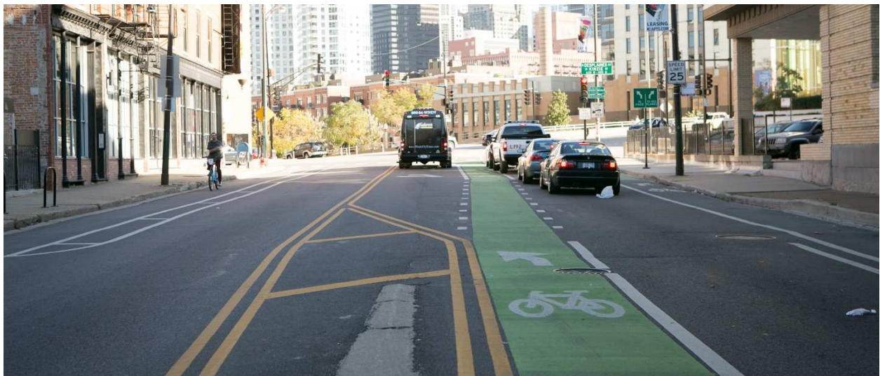
Figure 25 - A lateral shift adjacent to a left turn lane with skip-dash striping with colored pavement and turn lane symbol on Milwaukee Avenue in Chicago
