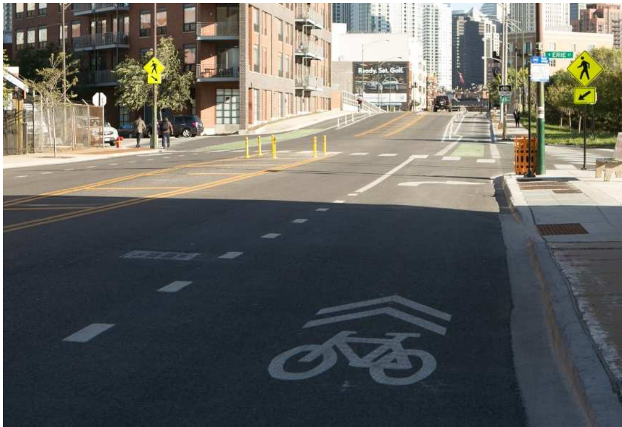
Figure 19 - Mixing zone on Milwaukee Avenue in Chicago
