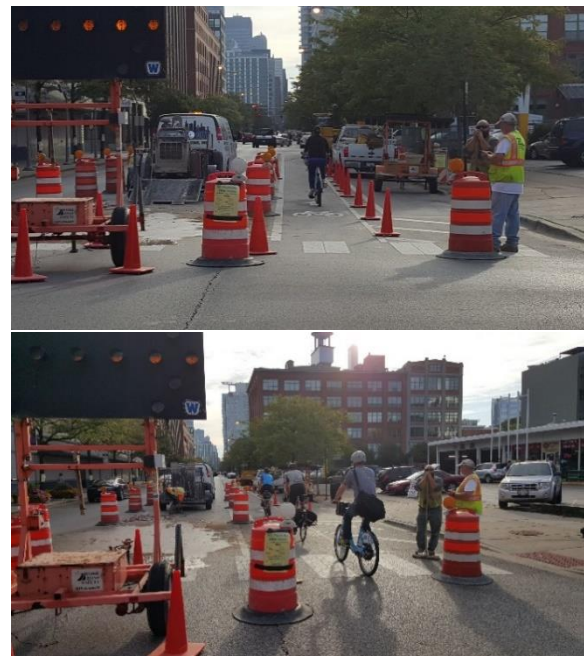
Figure 12 – Example maintenance of traffic that leaves an adjacent buffered bicycle lane open in Chicago
