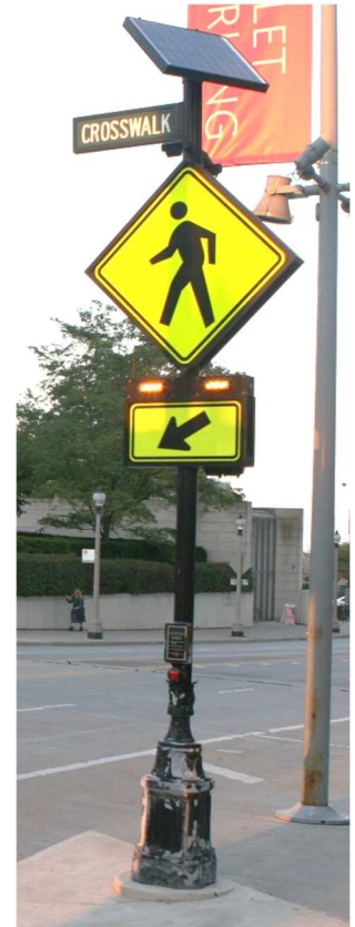
Figure 7 - RRFB on Monroe Street in Chicago, between Millennium Park and the Art Institute of Chicago.
