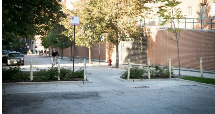
Figure 2 - A bicycle cut through, a bicycle boulevard feature, at Plymouth Court and Polk Street in Chicago
