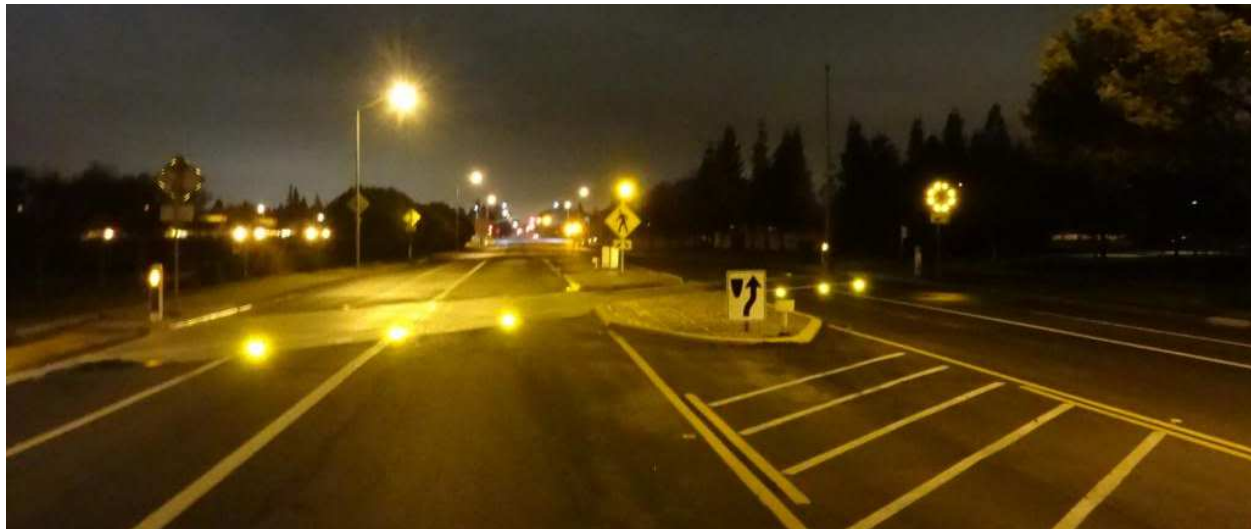
Figure 1 – A lighted crosswalk at night in Clovis, California. Image by James Sinclair , reprinted with permission.
