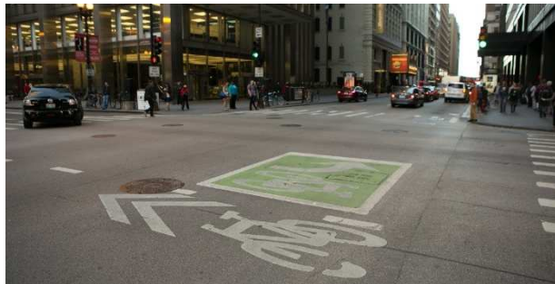
Figure 6 - A two-stage turn box in Chicago
