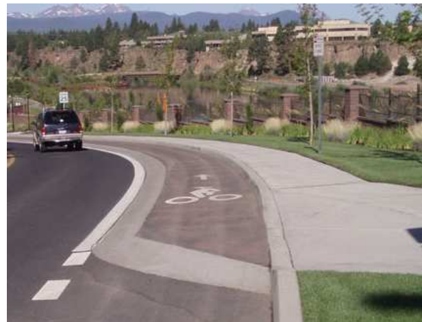
Figure 4 - Raised SBL (intermediate level between roadway and sidewalk) in Bend, Oregon. Image from Urban Bikeway Design Guide, by NACTO. Copyright © 2014 National Association of City Transportation Officials. Reproduced by permission of Island Press, Washington, D.C.
