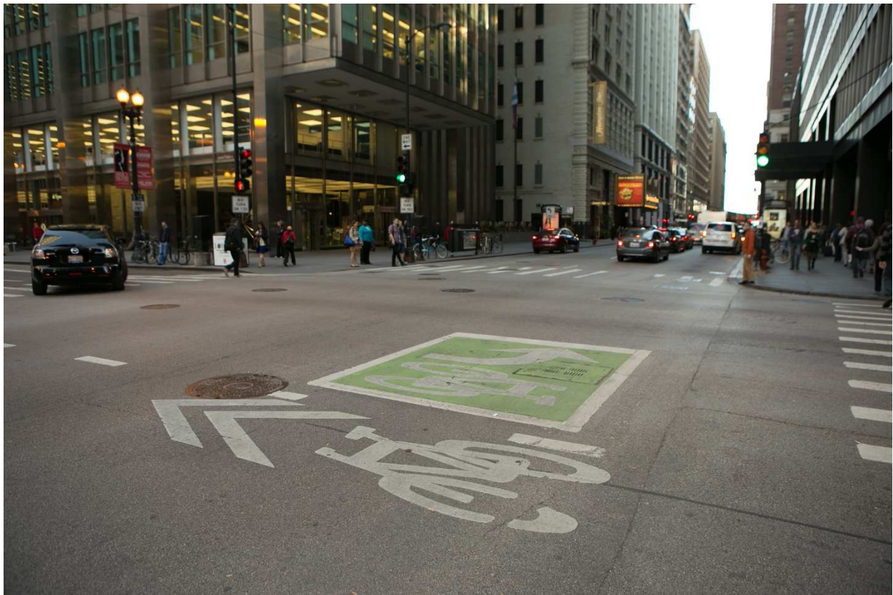
Figure 58 - Two-stage turn box at intersection of Dearborn Street and Monroe Street in Chicago
