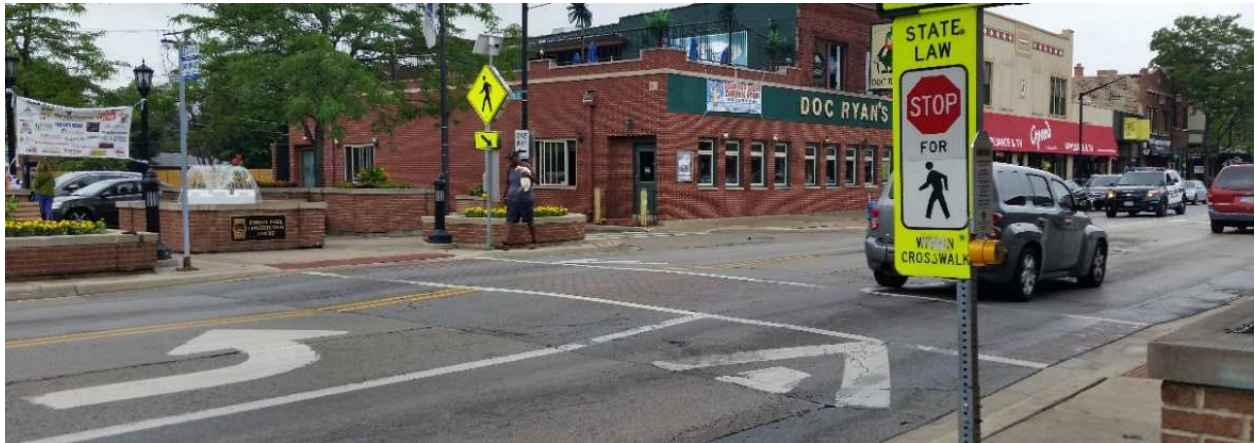
Figure 26 - Raised crosswalk location on Madison Street between Burkhardt Court and Thomas Avenue. Tube Set A is not yet installed.
