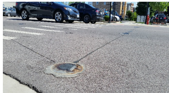
Figure 2 - Unidirectional in-roadway warning lights on Roosevelt Road (IDOT) at Lombard Avenue in Oak Park, Illinois
