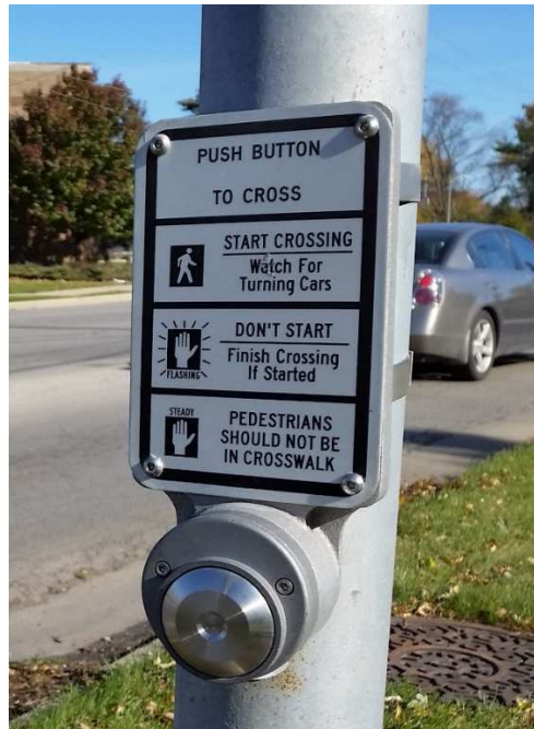
Figure 4 - Pushbutton detectors with mandatory instructional signing mounted directly above the pushbutton (Image: MUTCD, Sec. 4E.08)
