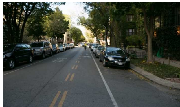
Figure 10 - Contraflow bicycle lane in Chicago
