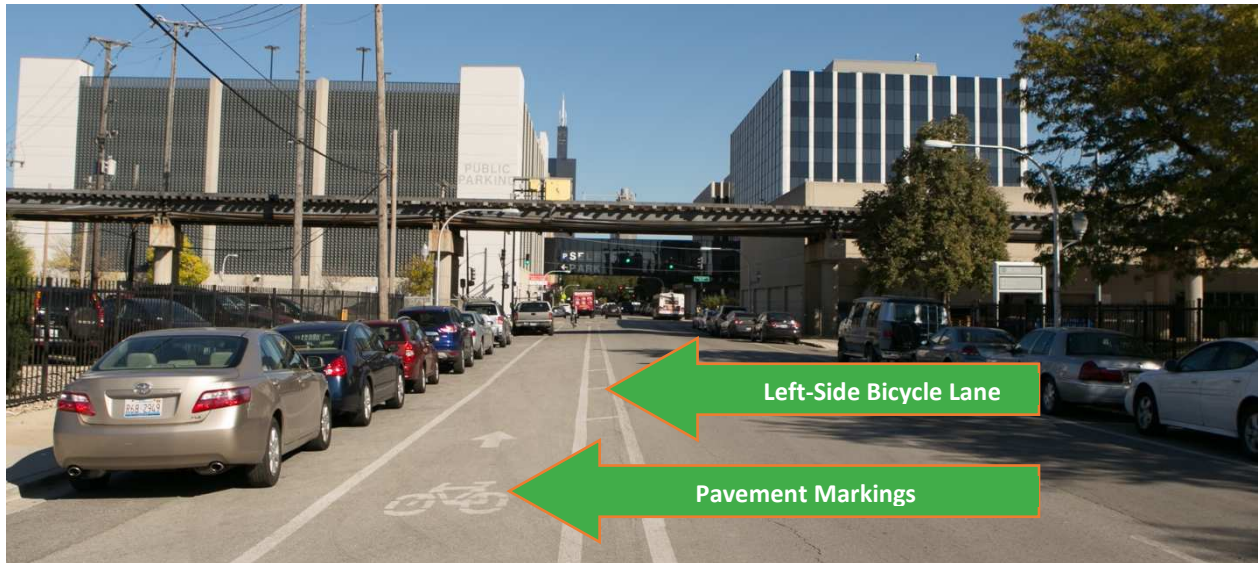
Figure 1 – Left-side bicycle lane on Jackson Boulevard in Chicago
