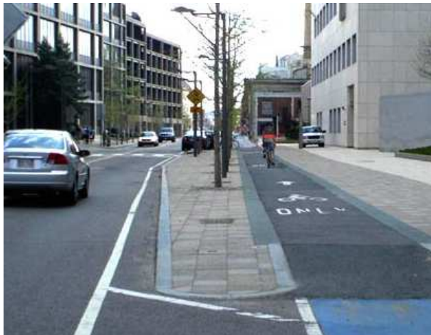
Figure 3 - Raised SBL (level with sidewalk) in Cambridge, Massachusetts. Image from Urban Bikeway Design Guide, by NACTO. Copyright © 2014 National Association of City Transportation Officials. Reproduced by permission of Island Press, Washington, D.C.
