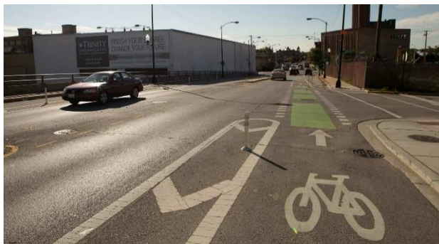
Figure 13 - Dotted striping and colored pavement intersection marking along the 18th Street separated bicycle lane in Chicago.
