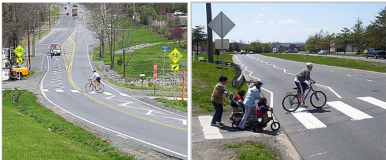
Figure 11 - Zig-zag markings on the approach to various shared use path crossings in Virginia. Reprinted with permission, by Lance E. Dougald. Source: http://www.virginiadot.org/vtrc/main/online_reports/pdf/11-r9.pdf
