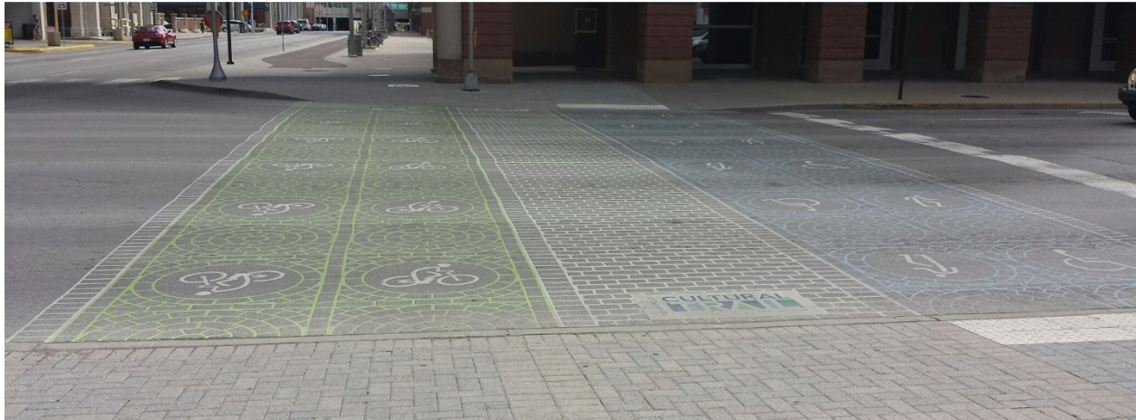
Figure 8 - Alternative pavement markings at a bicycle trail and pedestrian crossing in downtown Indianapolis, Indiana
