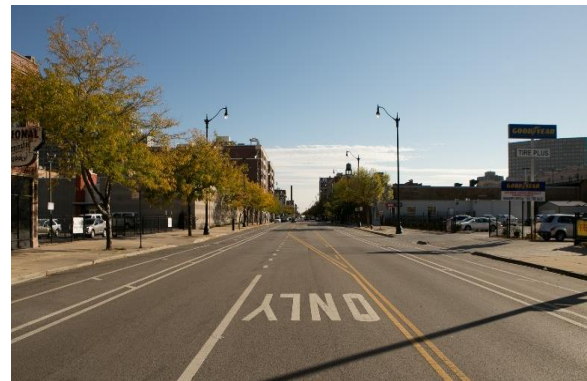
Figure 10 - Road diet on Wabash Avenue in Chicago- photo of the after design.
