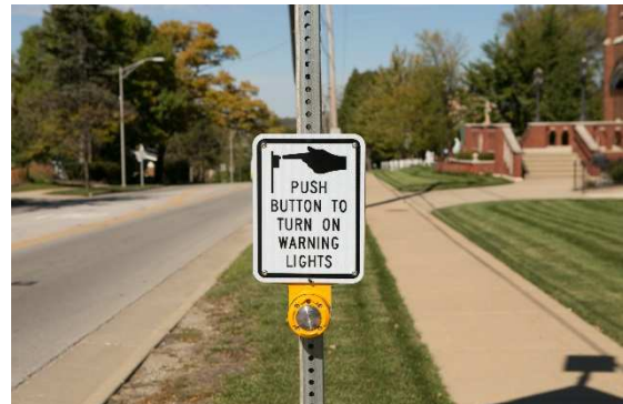
Figure 8 - Pedestrian push button for activation of RRFB in Lemont, Illinois.
