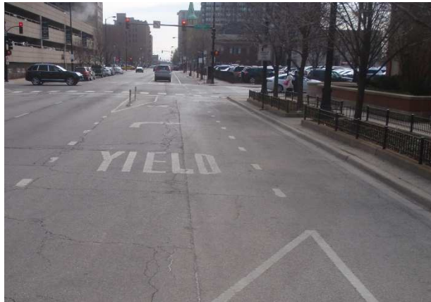
Figure 20 – A mixing zone with yield markings and a right-side dotted bicycle lane on Madison Street in Chicago.
