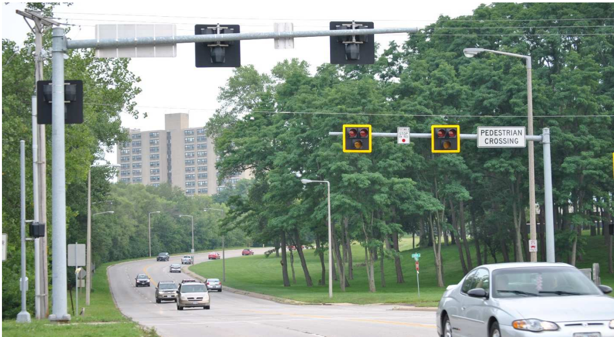
Figure 1 – PHB at a shared use path crossing in Pekin, Illinois
