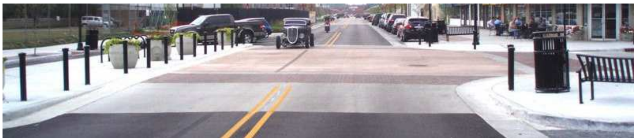
Figure 2 – Raised intersection. Image from Urban Bikeway Design Guide , by NACTO. Copyright © 2014 National Association of City Transportation Officials. Reproduced by permission of Island Press, Washington, D.C.
