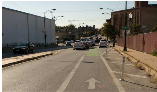
Figure 24 - Approach to a skip-dash striping, colored pavement, and shared lane lateral shift on 18th Street in Chicago
