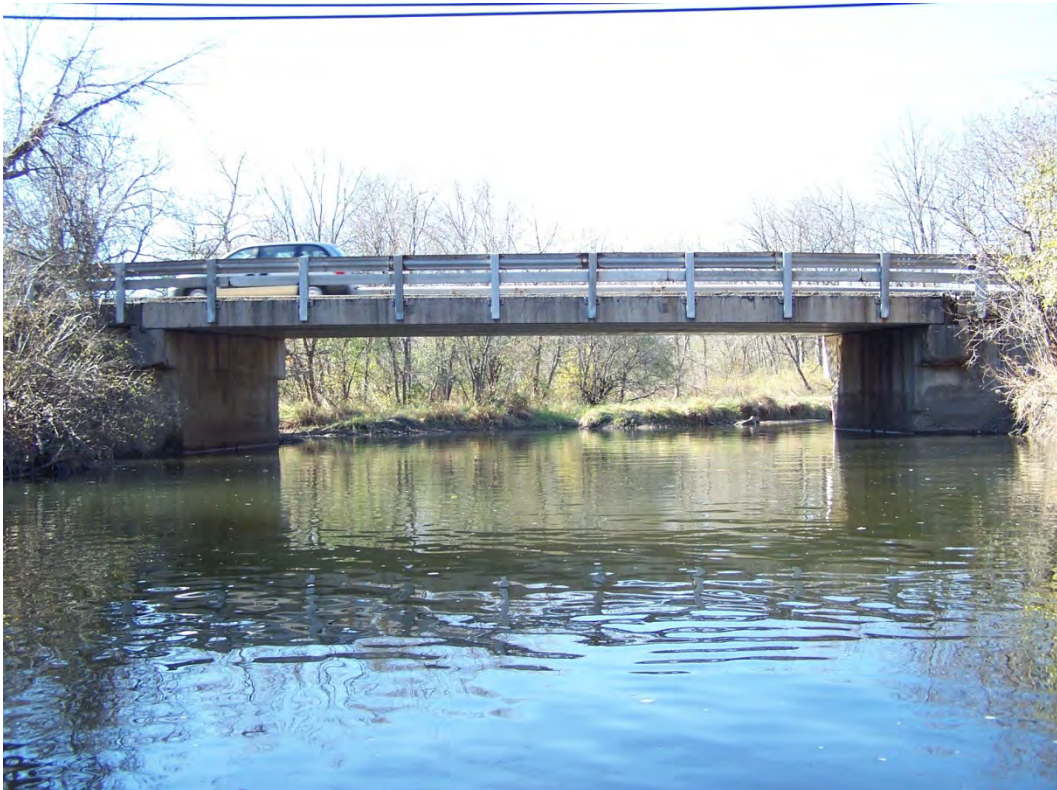
Location: Looking west (upstream) at east face of bridge.
