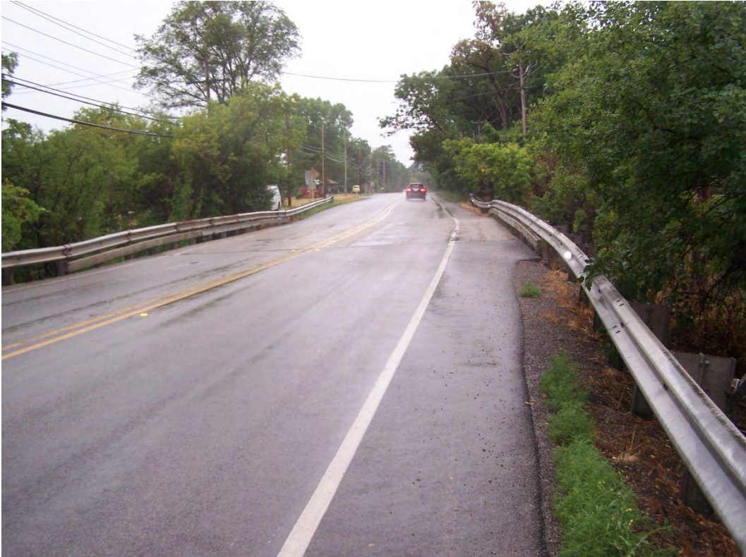
Location: Illinois Route 31 looking south at bridge over Ferson Creek.
