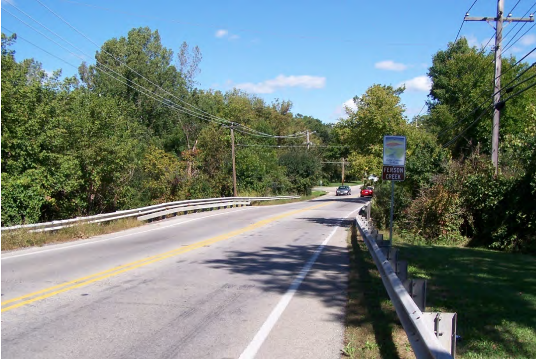
Location: Illinois Route 31 looking north at bridge over Ferson Creek.
