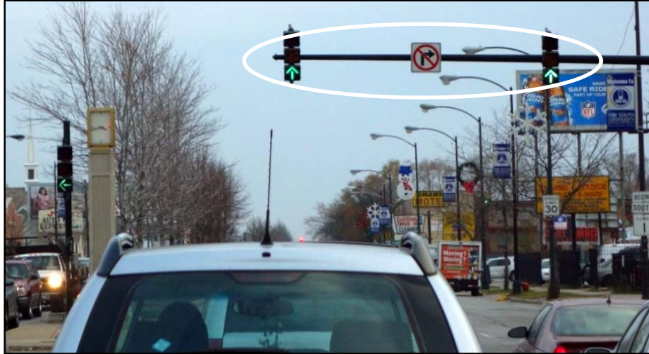
Figure 2-10. No Right Turn sign mounted on mast arm to increase visibility (Image: Huaguo Zhou).
