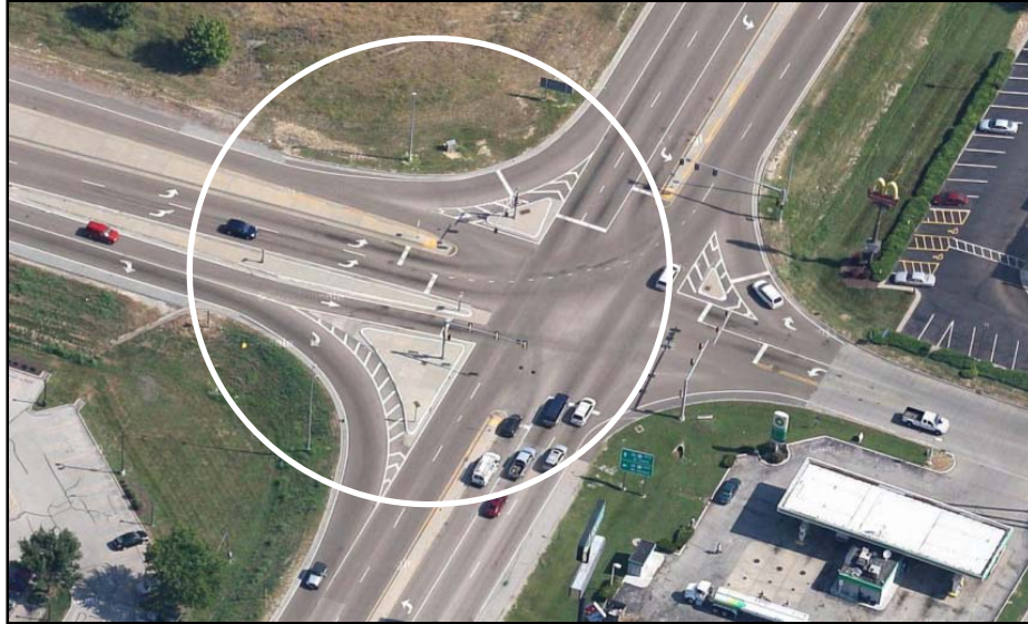
Figure 3-15. Raised median for separating same direction of traffic on an exit ramp (Image: Google Maps).
