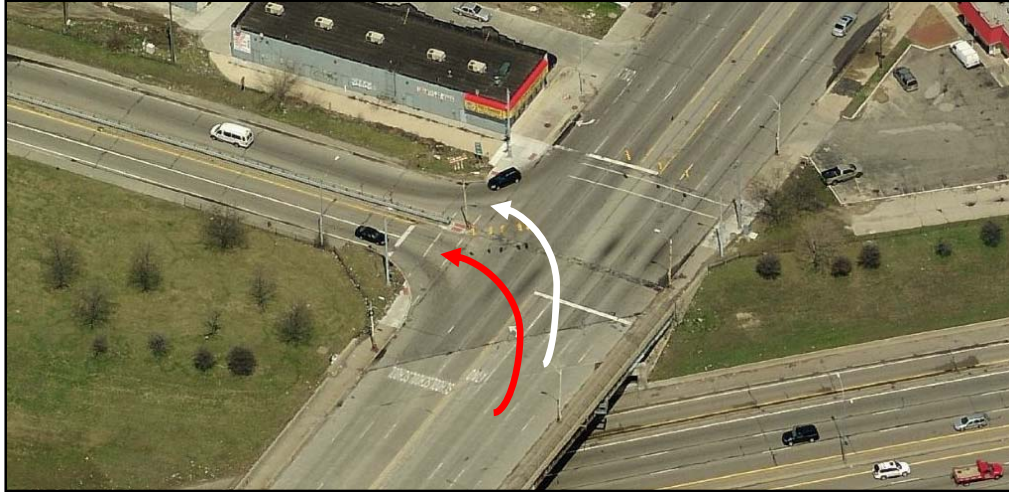
Figure 3-11. Plan view of a treated intersection before treatment with proper (white) and wrong (red) movements (Image: Bing).
