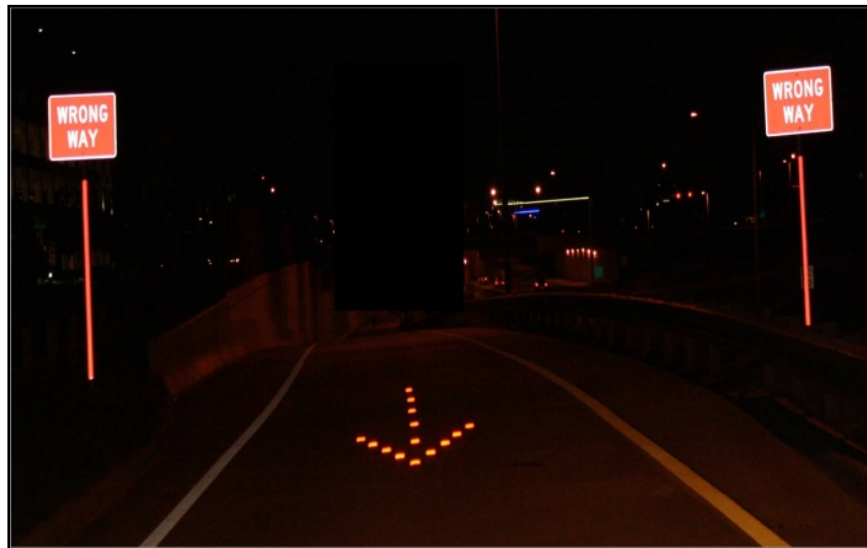
Figure 2-13. Supplemental WW signs and a WW arrow with RPMs (Image: Yang Ouyang).
