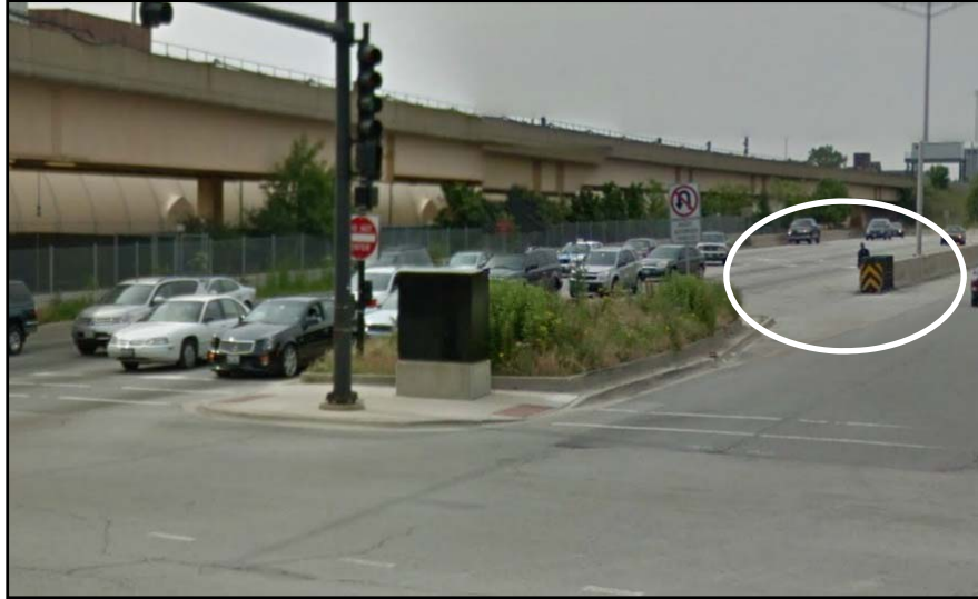
Figure 3-22. Short concrete barrier for a better view of throat of entrance ramp (Image: Google Maps).
