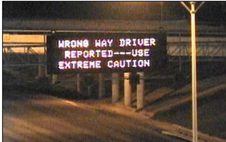
Figure 4-9. Changeable message sign (CMS) to alert right-way drivers (TxDOT 2011).
