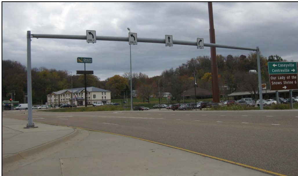
Figure 2-27. Overhead lane-use signs at exit ramps (Image: Huaguo Zhou).
