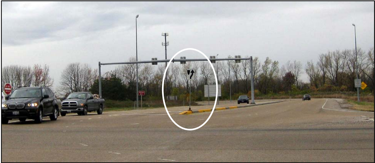
Figure 2-9. Keep Right sign at the median of parclo interchange (Image: Huaguo Zhou).
