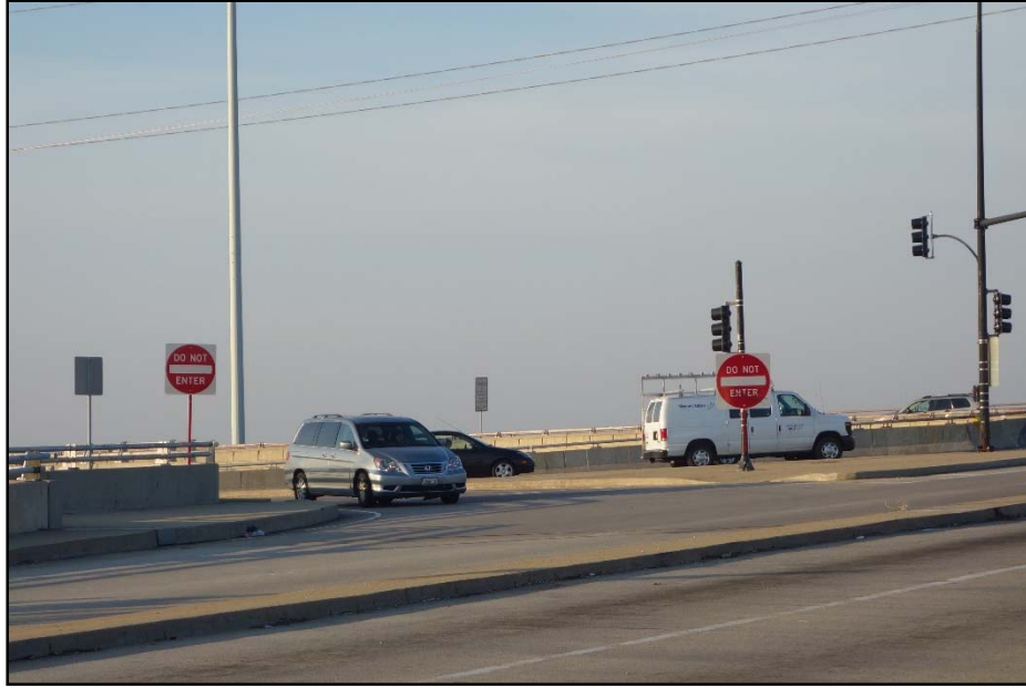
Figure 2-1. Signs facing potential wrong-way drivers at a SPDI.
