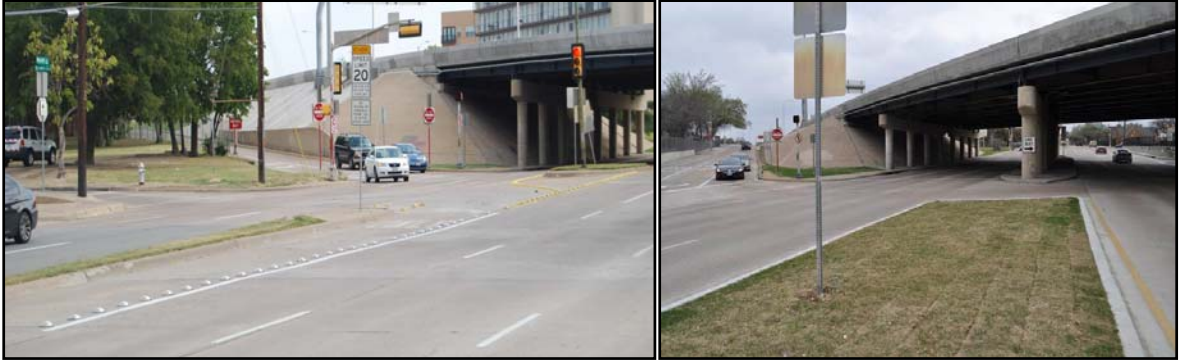
Figure 3-13. Before (left) and after (right) application of raised median to prevent wrong-way maneuvers (Ouyang 2013; Zhou et al. 2012).
