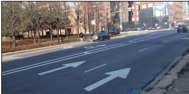
Figure 2-12. Directional pavement arrows at intersection (Image: Huaguo Zhou).
