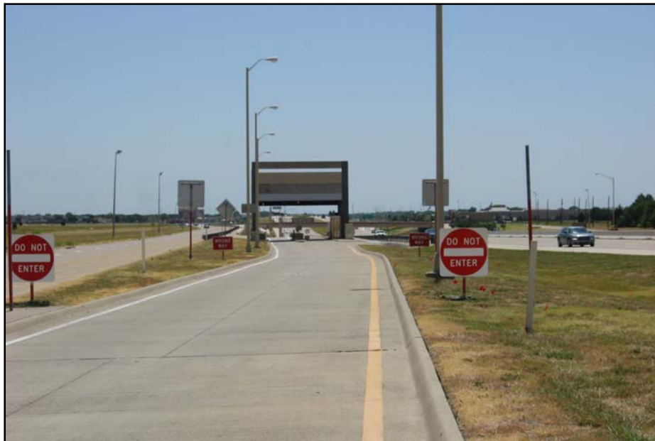
Figure 2-4. Lower-mounted DNE and WW signs along exit ramp (Ouyang 2013).
