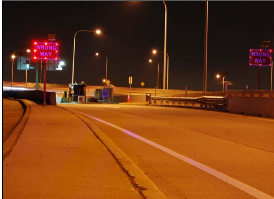
Figure 2-7. LED-enhanced WW signs (Ouyang 2013).
