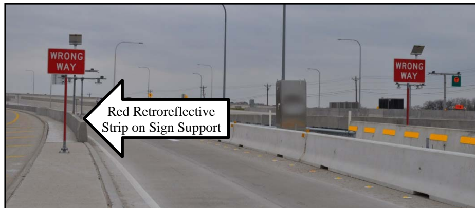
Figure 2-6. Red retroreflective strips on WW sign supports (Image: Yang Ouyang).
