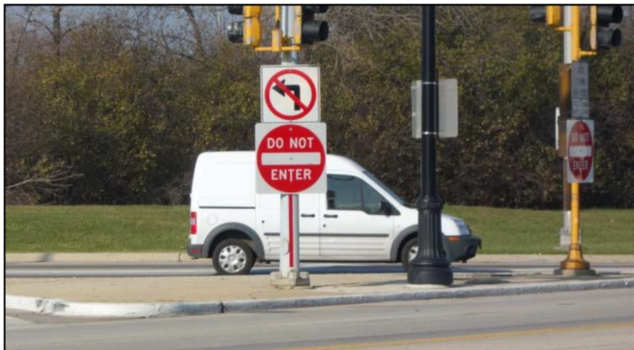
Figure 2-11. Additional No Left Turn sign facing to potential wrong-way drivers (Image: Huaguo Zhou).
