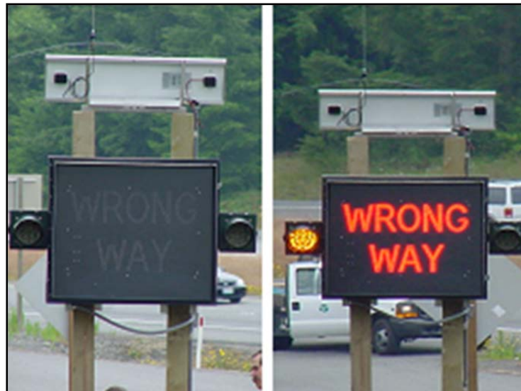
Figure 4-8. LED wrong-way sign to alert wrong-way drivers (Cooner et al. 2004).
