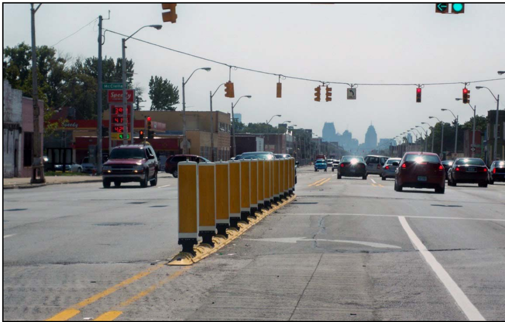
Figure 3-12. Application of longitudinal channelization in restriction of left-turn access (Morena and Ault 2013).
