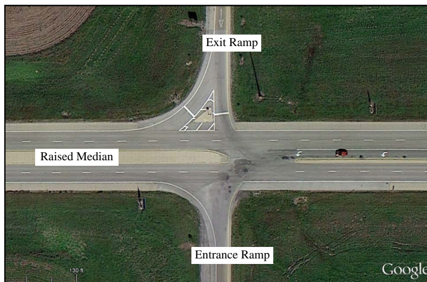
Figure 3-10. A non-traversable raised median at the ramp-crossroad intersection of a diamond interchange (Image: Google Earth).
