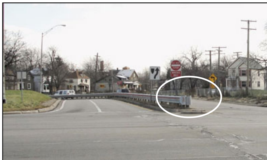
Figure 3-21. Median barrier (guardrail) blocking view of throat of entrance ramp (Morena and Leix 2012).
