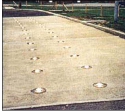
Figure 4-11. In-pavement Warning lights (Cooner et al. 2004).
