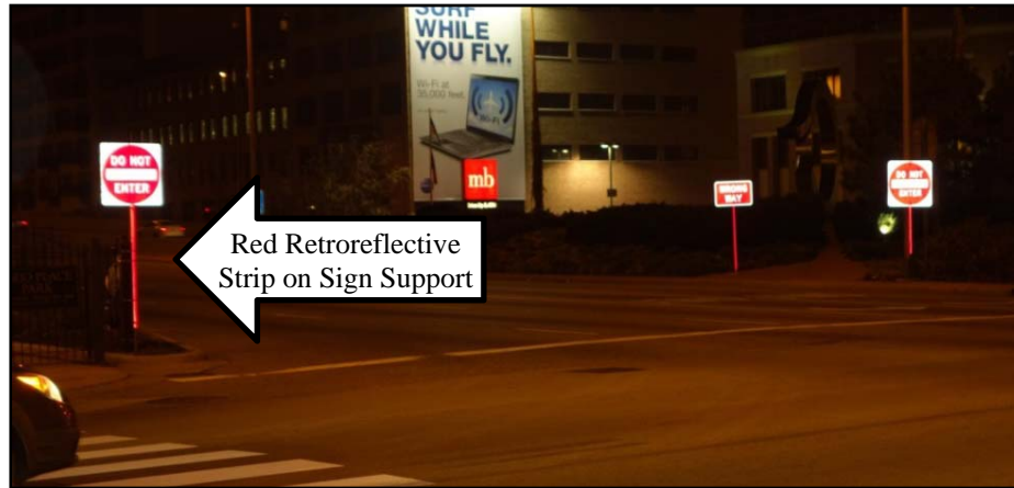
Figure 2-5. Red retroreflective strips on DNE sign supports (Image: Huaguo Zhou).
