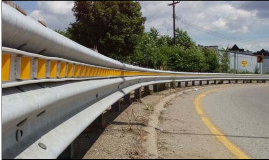
Figure 2-15. Barrier delineators visible while traveling in the correct direction (Morena and Ault 2013).
