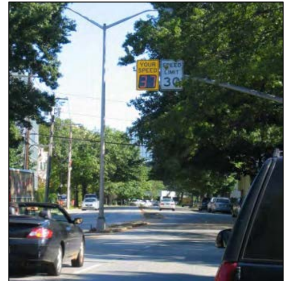
Speed awareness device installed at same time as roundabout
