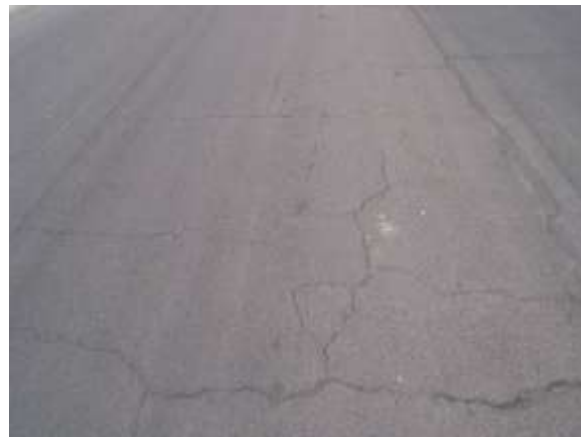
Light Block Cracking – Tight cracks or sealed cracks with the filler in good condition.
