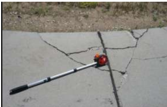
Severe Corner Breaks - Crack is heavily spalled; corner is broken into two or more pieces, is faulted, or moves under load.
