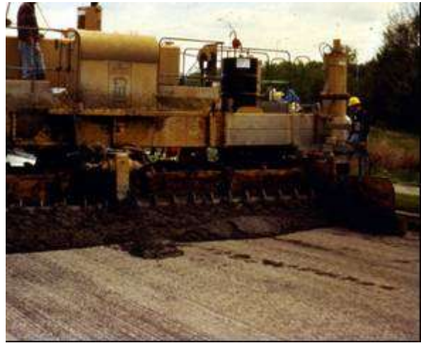
Step 3. PCC placement. PCC is placed using conventional methods.
