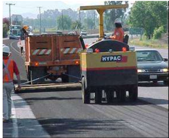
Steps 4 & 5. Drag-brooming of sand and rolling. After the application of sand, the surface is drag-broomed again and rolled with pneumatic-tired rollers.
