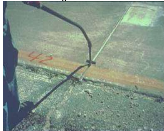
Steps 7 & 8. Curing & joint sealing. The final steps include texturing and providing adequate curing.
