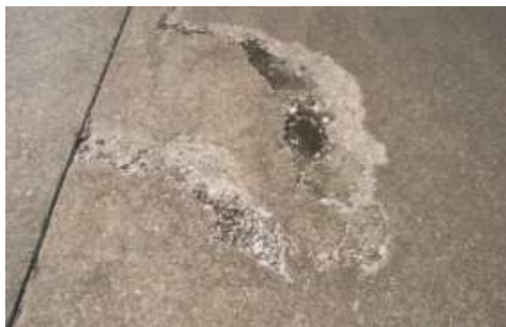
Moderate Surface Distress - Cracks have opened up and/or there is some material loss (scaling) on the pavement surface.
