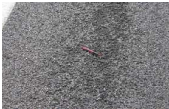
Moderate Weathering/Raveling - Some aggregate loss resulting in an overall rough pavement surface with some localized pitting.
