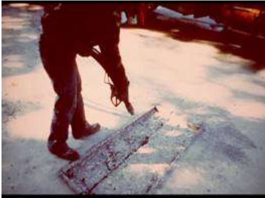
Step 3. Repair area preparation. The repair area should be sandblasted and cleaned to promote good bonding.
