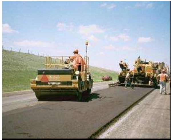
Steps 4. Rolling. Steel-wheeled rollers are used for final compaction.
