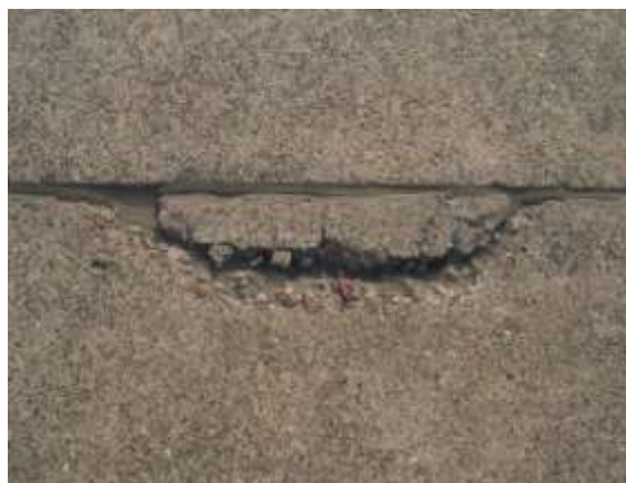
Light Spalling - Slight wear along the joint or crack, with minimal loose or missing pieces.
