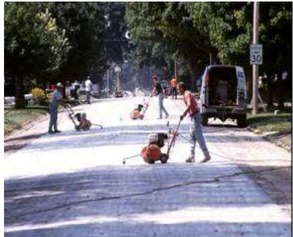
Step 5. Joint sawing & curing. Timely joint sawing is required to establish the contraction joints in the PCC pavement. Curing is important for UTW overlays due to the high surface-area-to-volume ratio.
