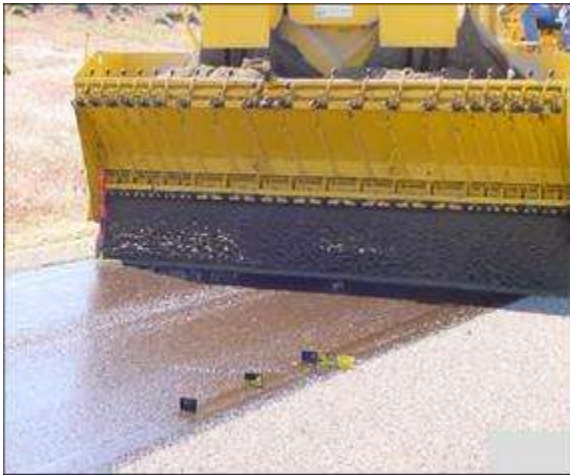
Step 3. Sand application. A thin layer of sand is applied to the broomed emulsion.
