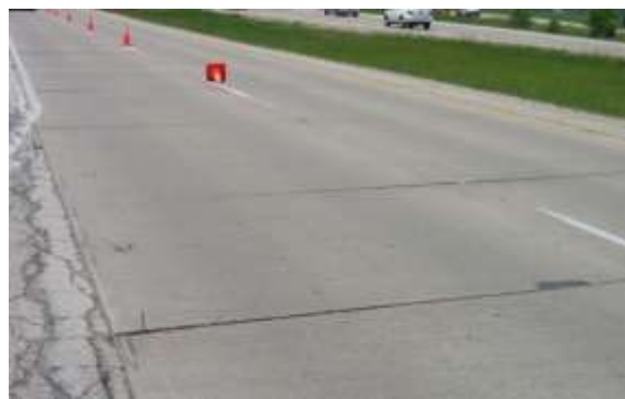
Light Faulting - Faulting is visible and measures approximately less than ¼ inch (6.4 mm) at a given location.
