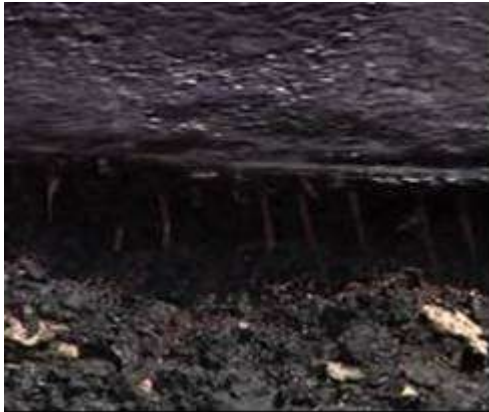
Step 3. Addition of Rejuvenator. A rejuvenating agent is sprayed onto the loosened material and mixed.
