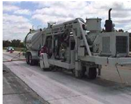
Steps 8 & 9. Diamond grinding & joint sealing. Final steps often consist of diamond grinding and joint sealing.
