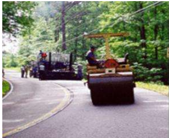
Step 4. Rolling. Steel-wheeled rollers are used to compact the overlay.
