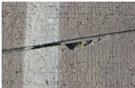
Light Joint Seal Damage - Only localized areas of the sealant are damaged.
