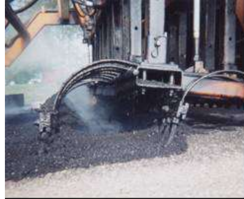
Step 2. Surface scarification. The surface is loosened with scarifying teeth.
