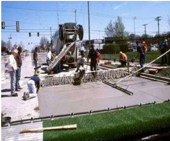
Step 4. Finishing & texturing. The PCC is finished and textured using conventional methods.
