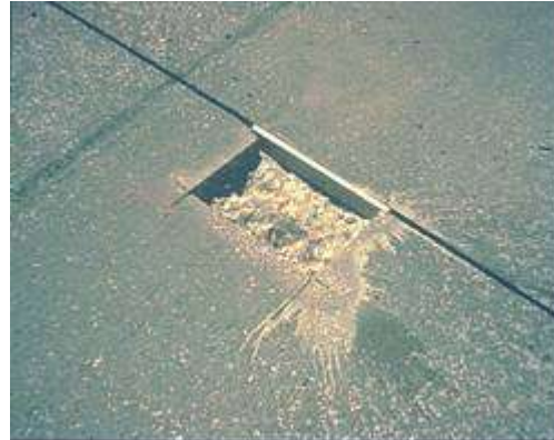
Step 4. Joint preparation. It is important to maintain the existing joint reservoir during construction.
