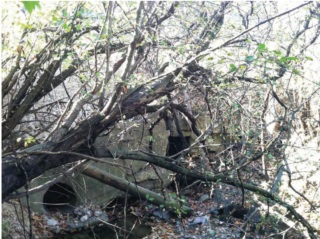
6. Southeast of Culvert Looking Northwest
