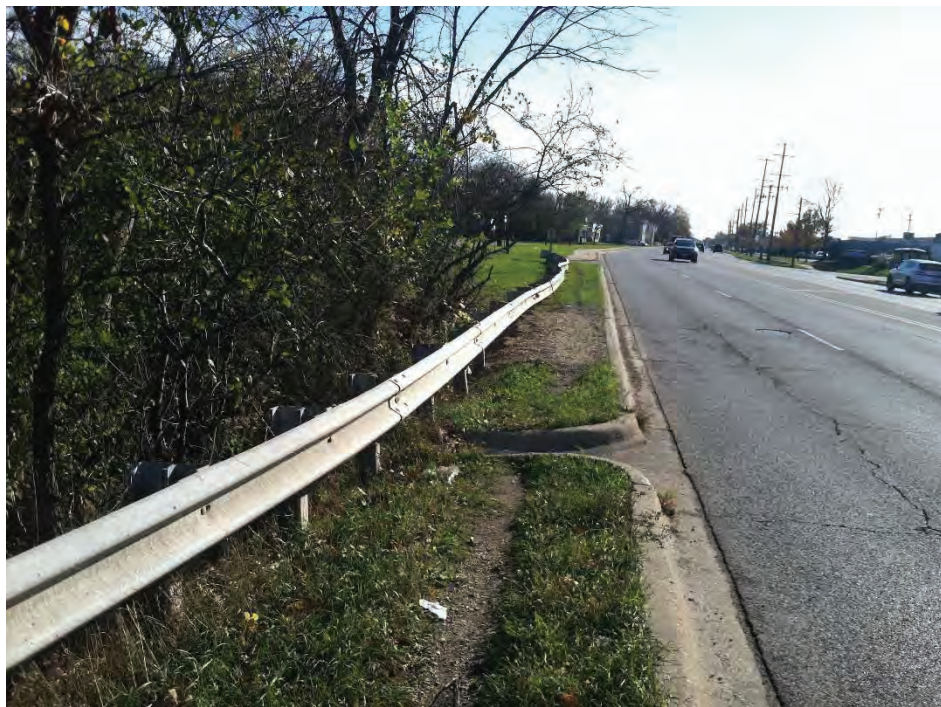
2. Des Plaines River Road (Looking south, north of culvert) (11/2016)
