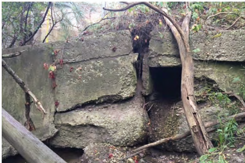
3b. 2x2 box culvert under Des Plaines River Road (looking west) (11/2016)
