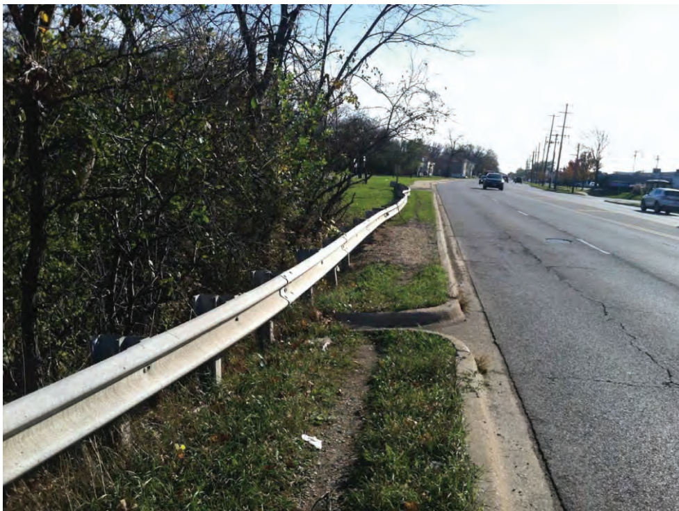
4. Looking South on River Road (Aggregate Fill Added by IDOT)
