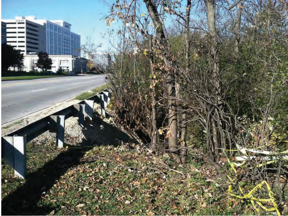
1. Des Plaines River Road (Looking north, south of culvert) (11/2016)
