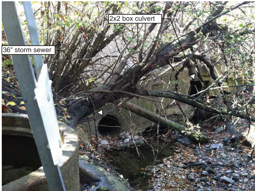
3a. Culverts under Des Plaines River Road (looking west) (11/2016)
