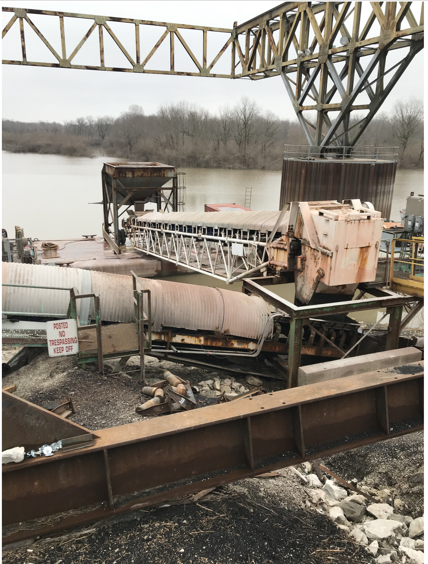
EXHIBIT 4-3: KASKASKIA REGIONAL PORT DISTRICT Conveyor Setup at Overhead Bridge Crane
