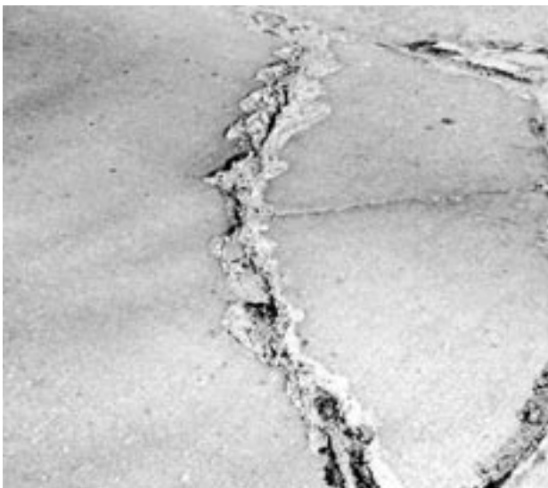
▶ Spalling over shallow reinforcing.
