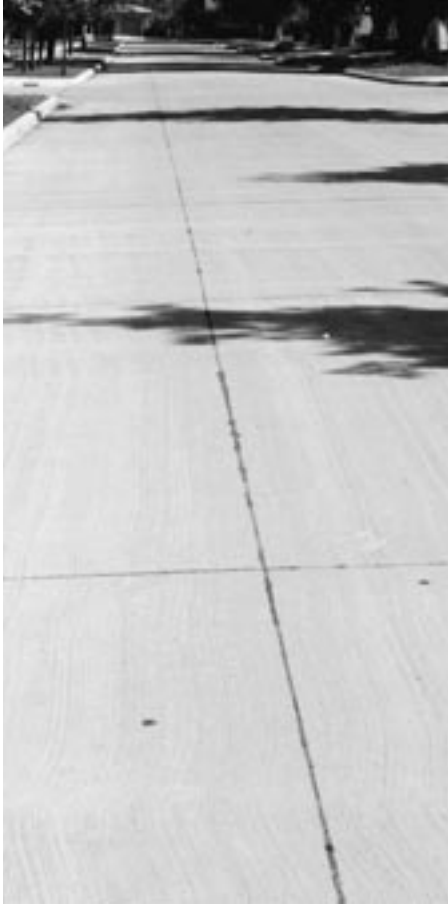
◀ New, well-sealed longitudinal joint.
