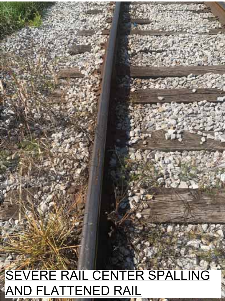
SEVERE RAIL CENTER SPALLING WITH EXCESSIVE FLAKING
