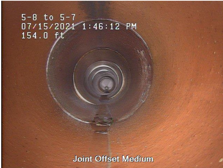
Example: Joint Offset Medium
