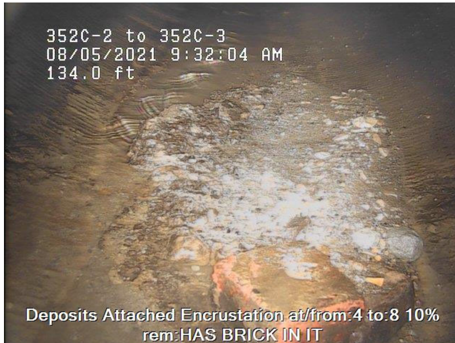
Example: Deposits with Attached Encrustation
