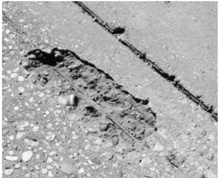
▶ Spalling over shallow reinforcing.
