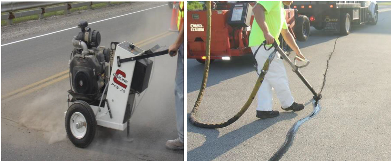
Figure 2- Crack Routing & Sealing
