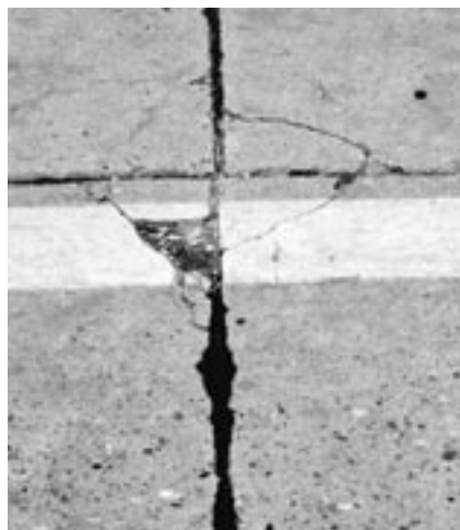
First signs of corner cracking.
