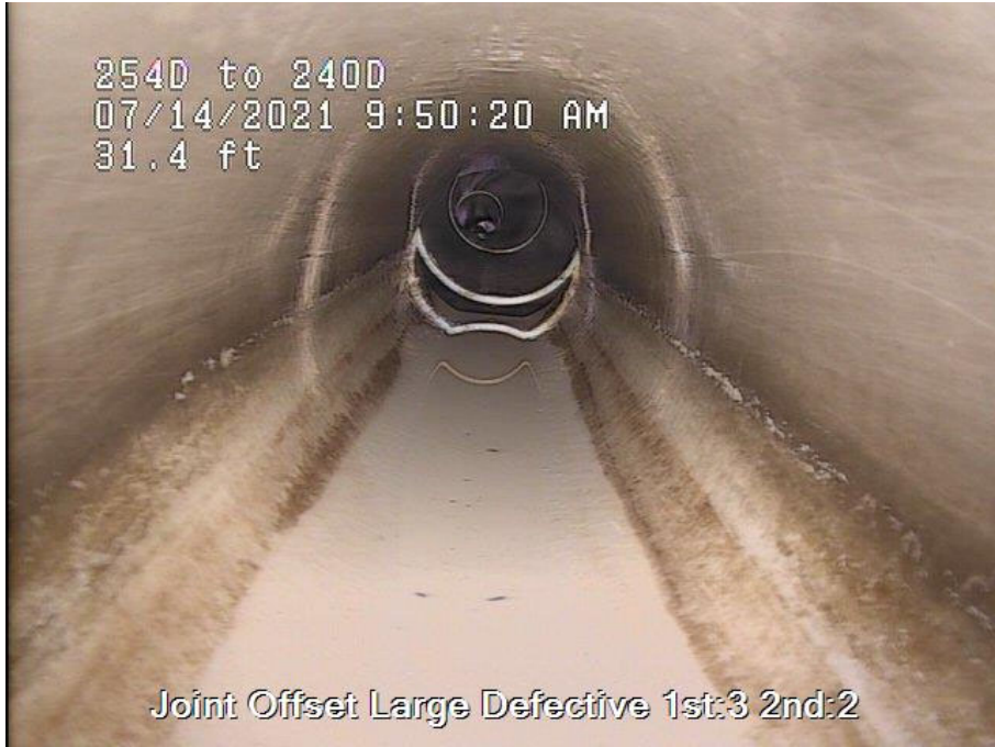
Example: Joint Offset – Large
