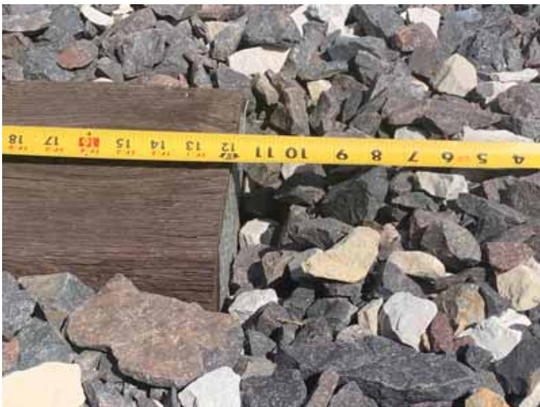
LATERAL TRACK MOVEMENT IN BALLAST SHOULDERS
