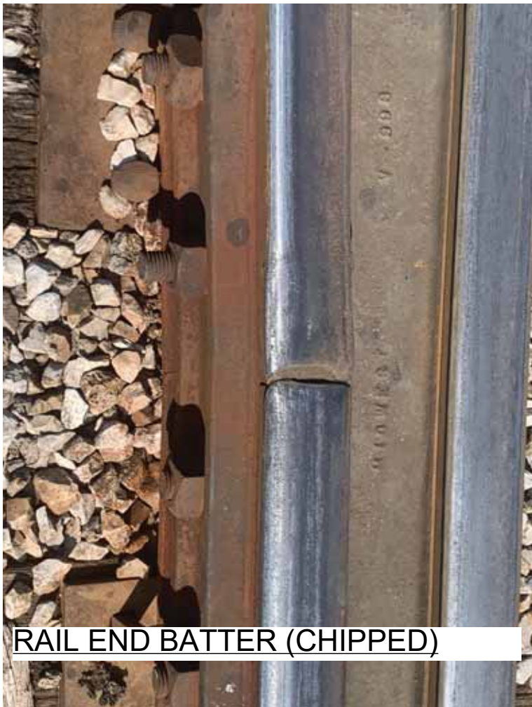
RAIL END BATTER (CHIPPED)
