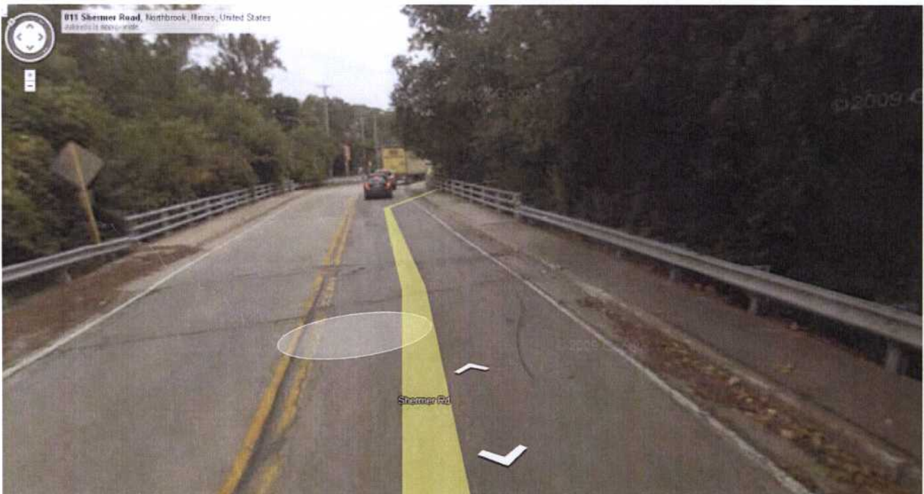
Location: Shermer Road looking north at structure over MF NB Chicago River
