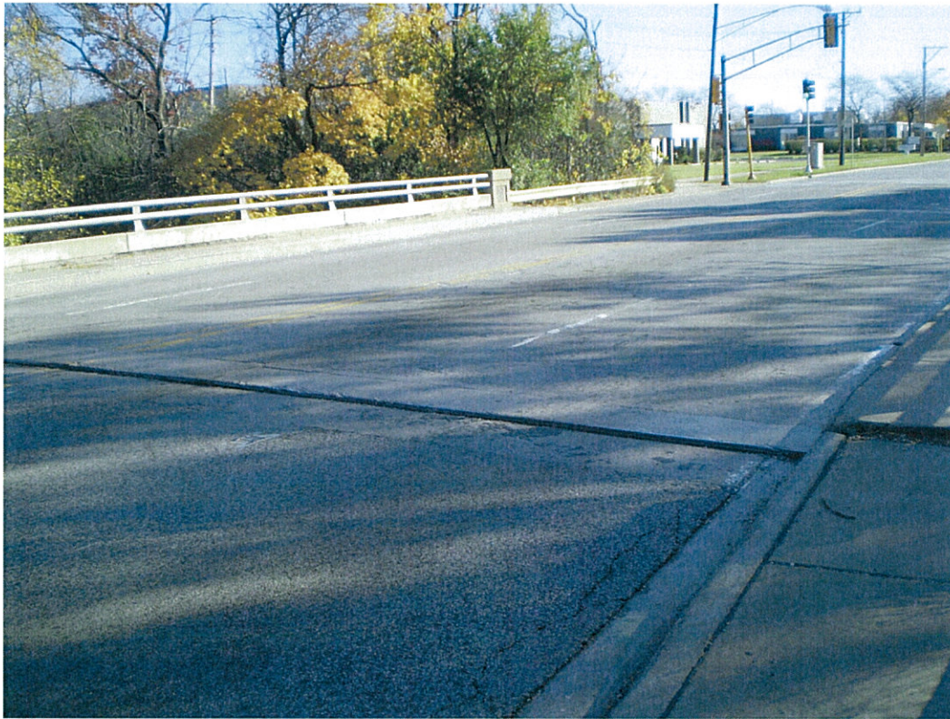
Location: Looking NE from SW corner
