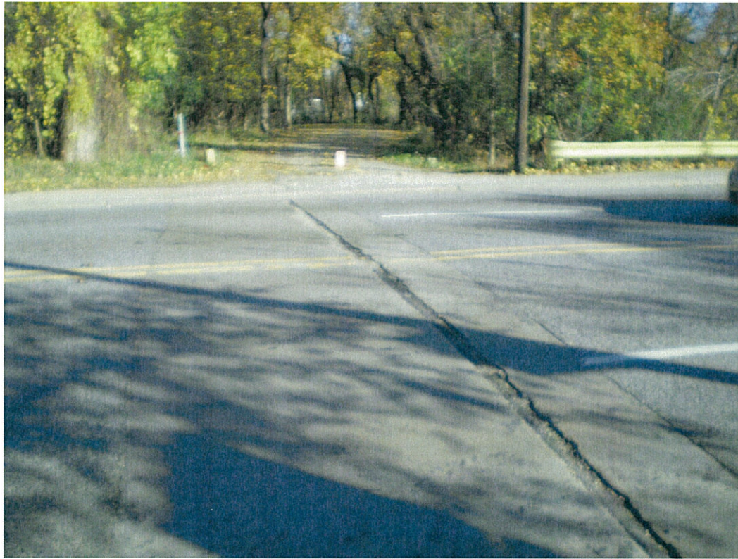
Location: W side of bridge looking N at bike trail
