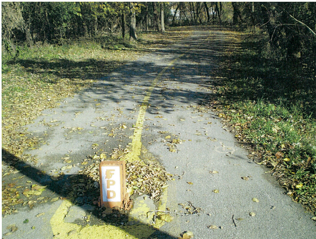
Location Bike path at NW corner
