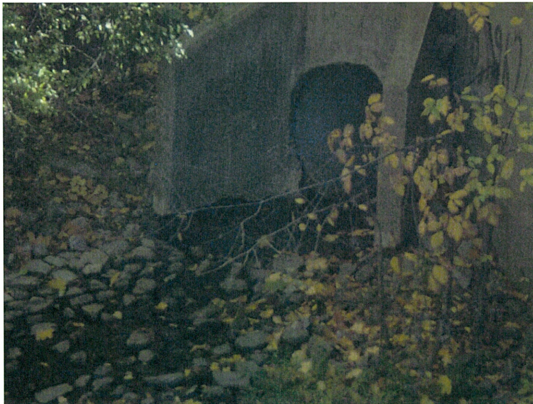
Locatio Culvert on NE side
