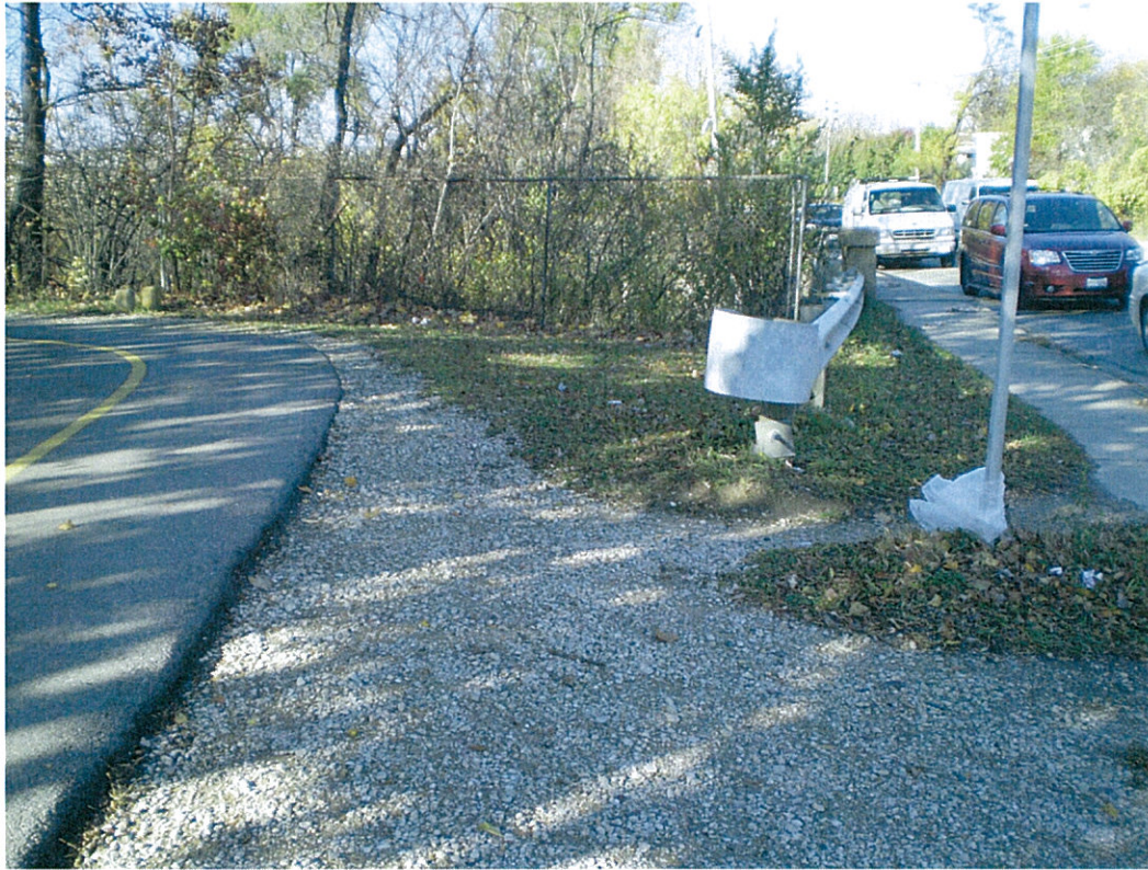
Location: Bike path at SE corner
