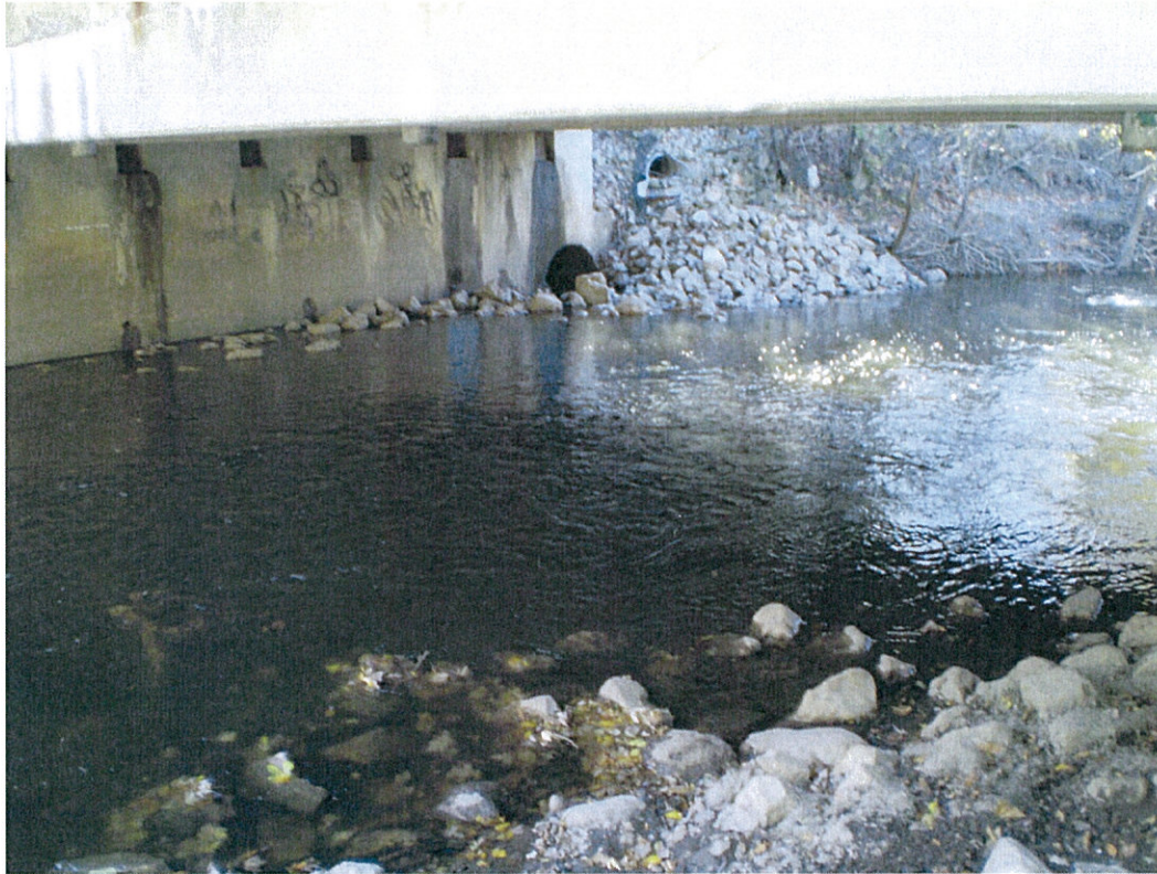
Location: Underneath structure from NW side
