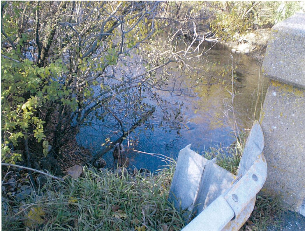
Locatio Guardrail at SE corner of bridge
