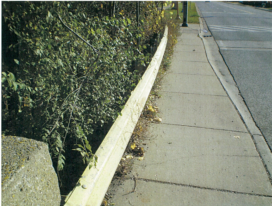
Location: Looking E from NE side
