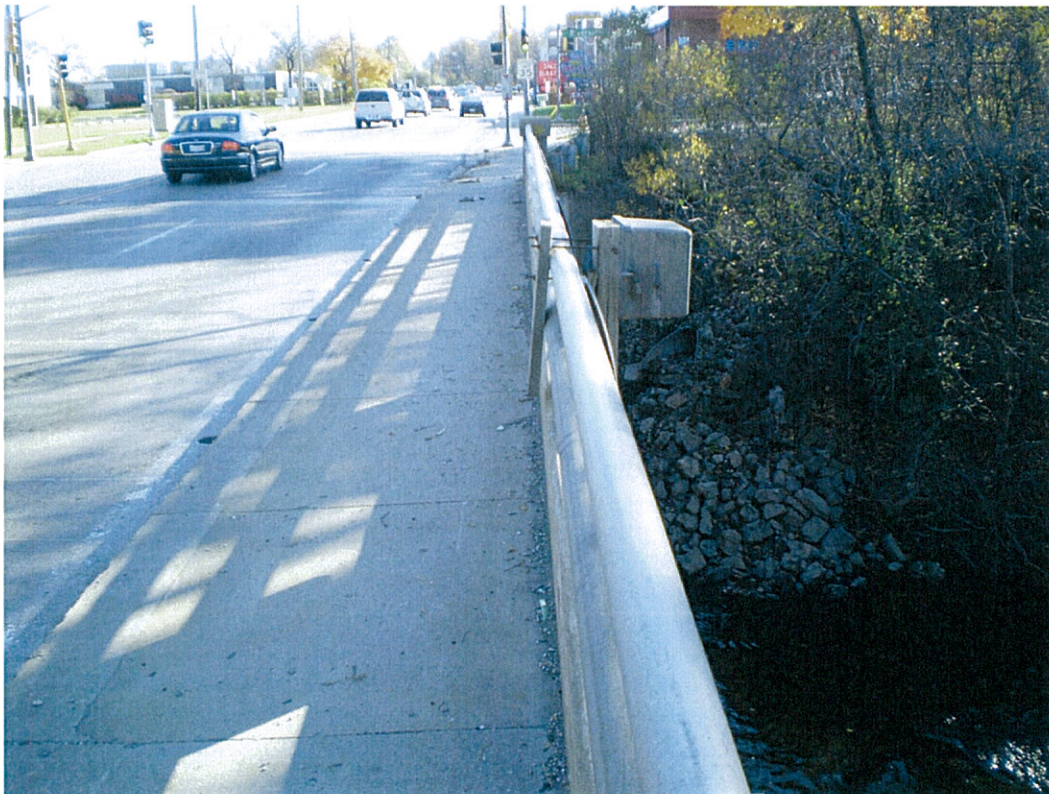
Location: Looking E along S side of bridge
