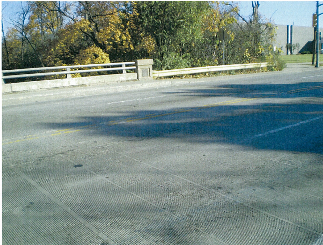
Locatio NE side of bridge from SE
