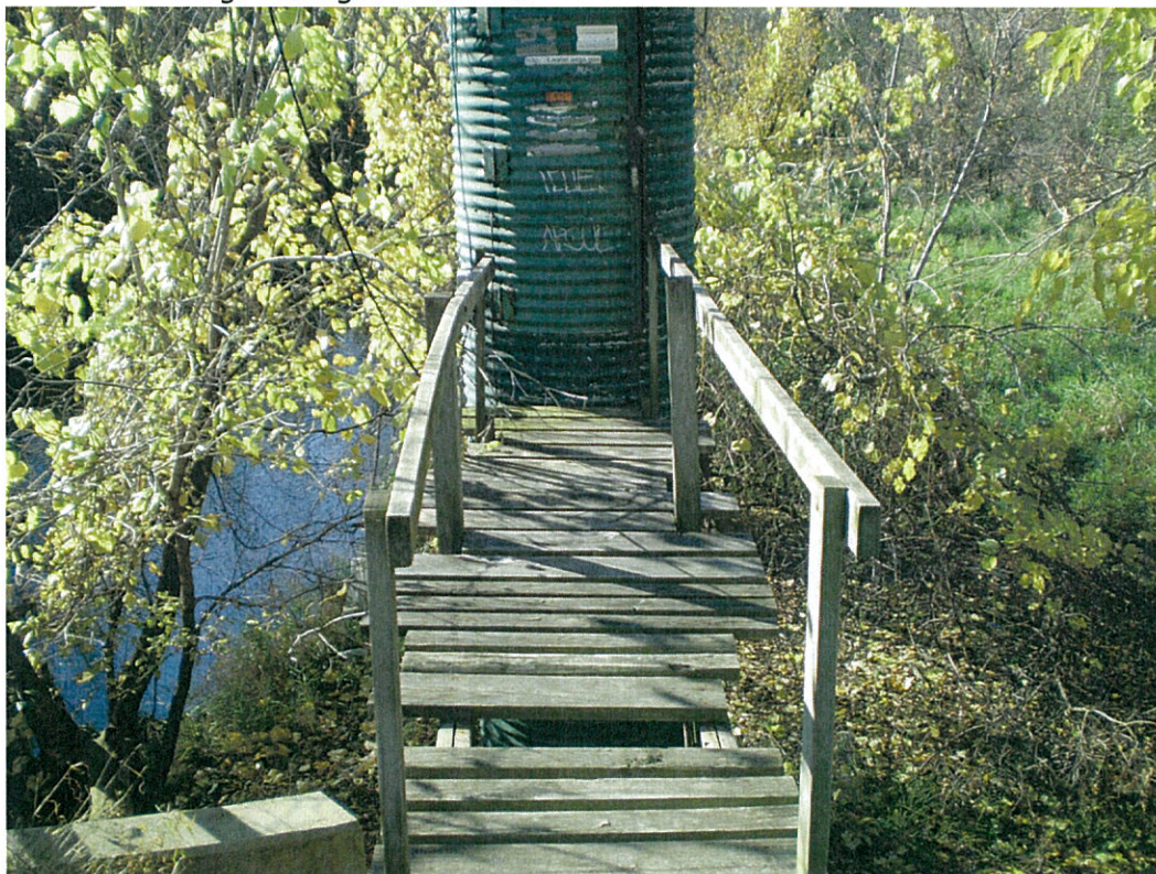
Locatio Structure on SW corner of bridge / Stream Gage House
