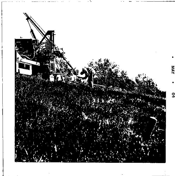
Figure 6. Day Labor's drill 245A was used on all 39-inch depth holes and others to 6-foot depth.
