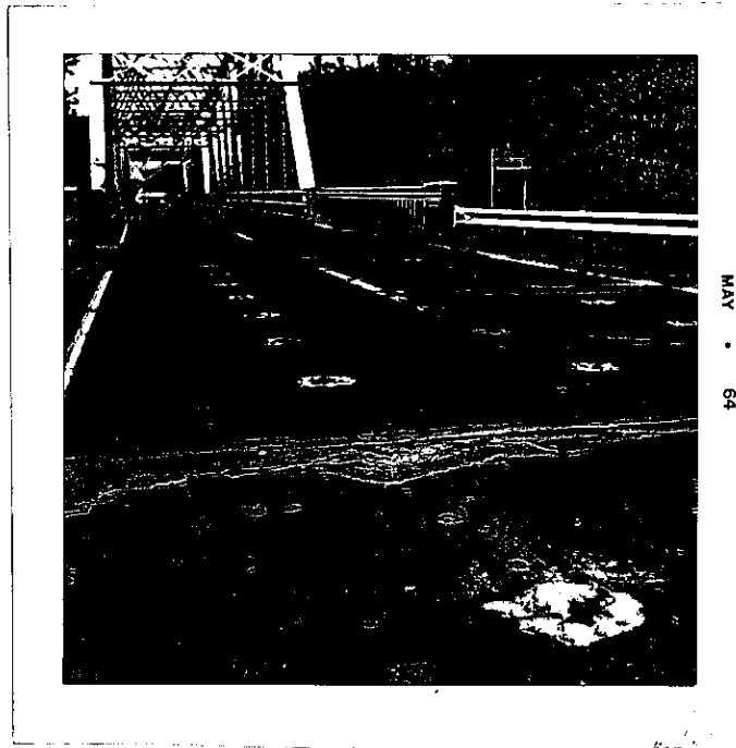
Figure 5. Pattern of holes star-drilled in pavement at bridge approaches preparatory to boring 6-inch diameter holes 39 inches deep for hydrated lime.
