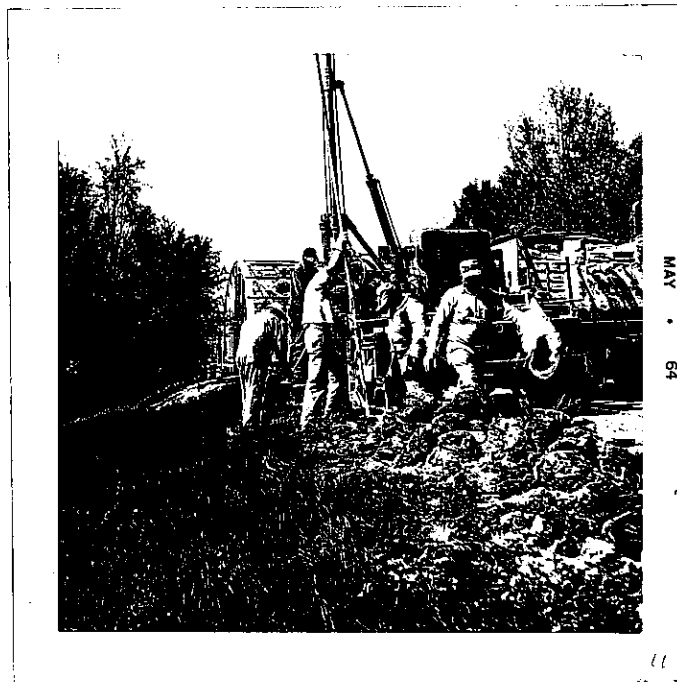
Figure 8. Cone-shaped piles of clayey auger peelings were made over the lime filled holes.
