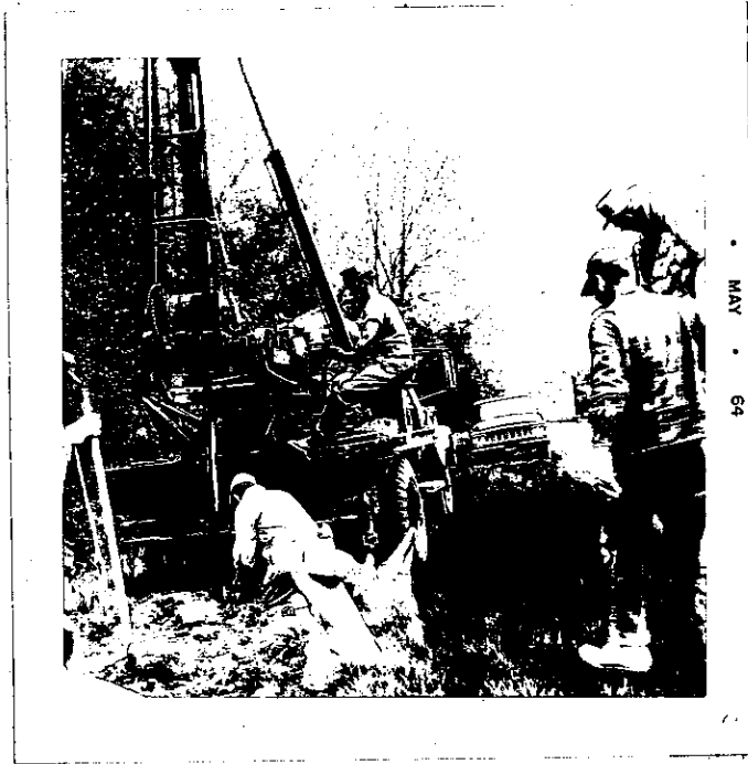
Figure 7. Drilling crew dusted hydrated lime into hole and an auger to aid in keeping the clay from sticking to auger. The previous hole is being tamped with lime backfill.
