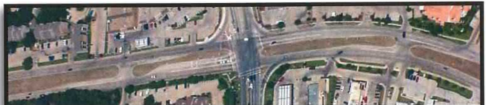
Turn lanes at median openings provide a safe haven for turning vehicles.
