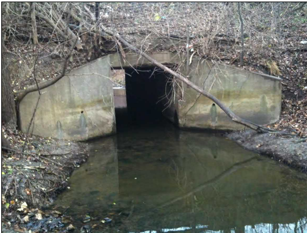
Photo 53 – Looking upstream (east) at the downstream face of IL 47 Culvert
