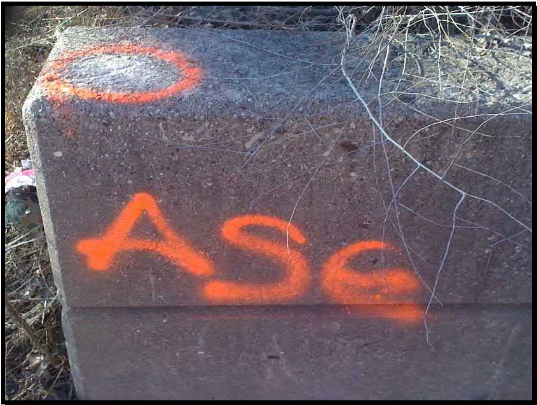
Photo 54. Southwest Wingwall benchmark
