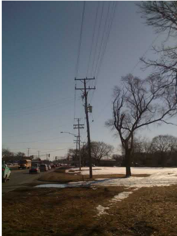
Photograph 7. Aerial utility lines crossing over the railroad behind the west abutment
