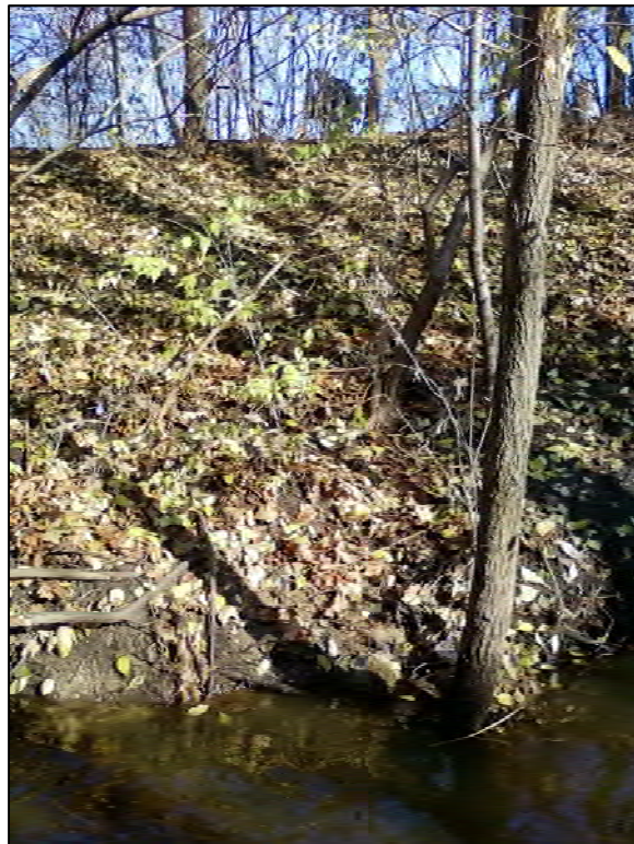
Photo 036 – 300' downstream section looking north
