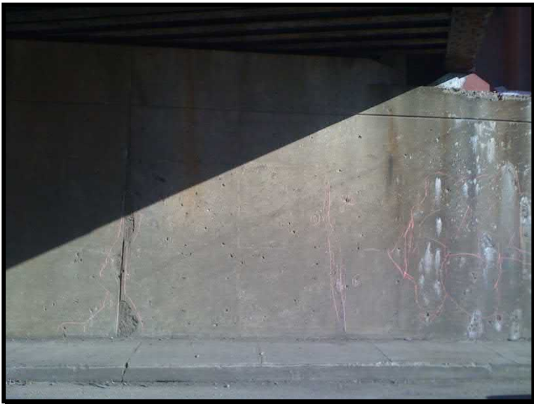
Photo 32. East Abutment Face—South Side
