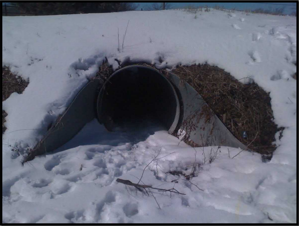
Photograph 5. North pipe at east end
