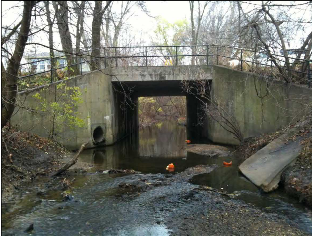
Photo 42 – Looking upstream (south) at downstream face of St. Johns Rd. Culvert
