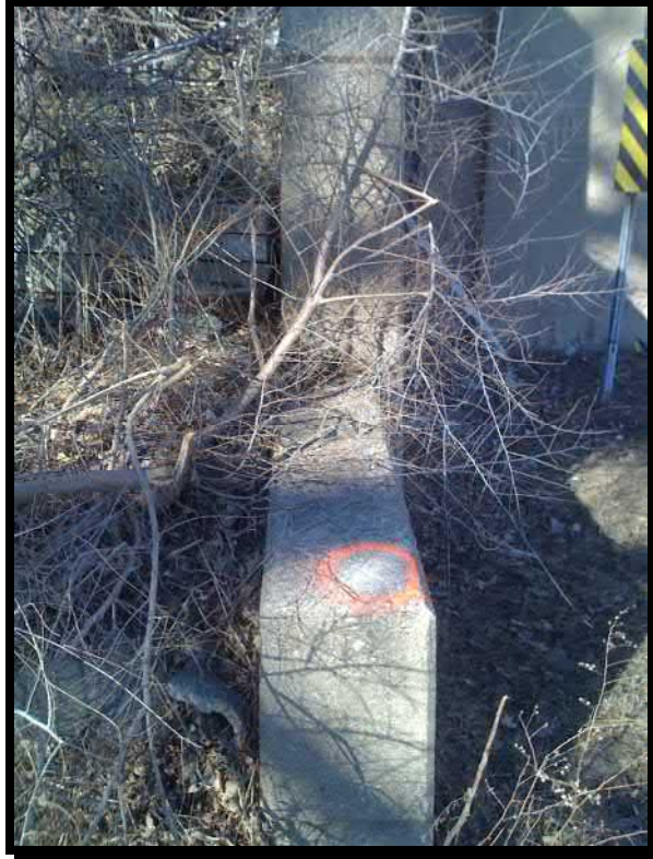
Photograph 11. Benchmark on southwest wingwall
