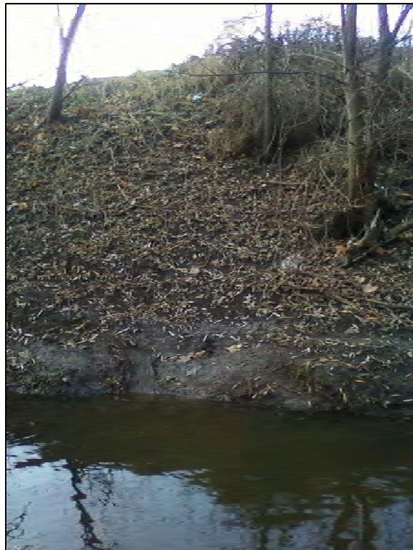
Photo 026 – 600' upstream section looking west
