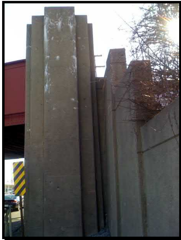
Photo 44. Northwest Wingwall and side of west abutment
