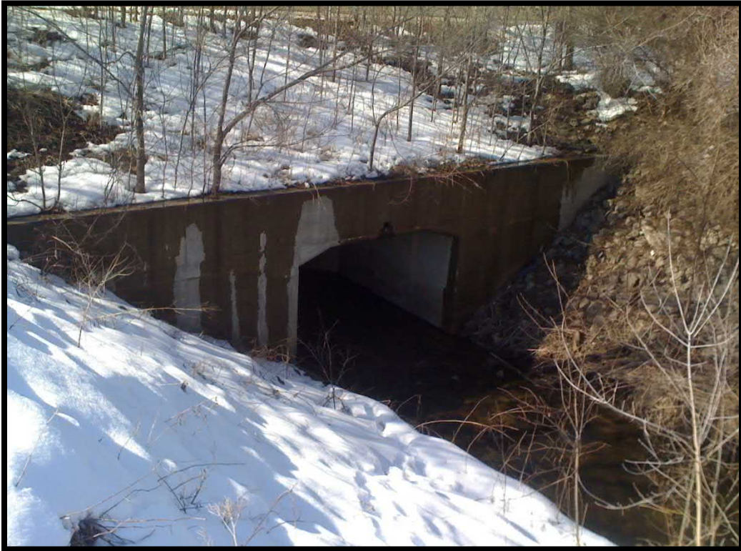
1. East end of culvert with headwalls parallel to IL Route 47
