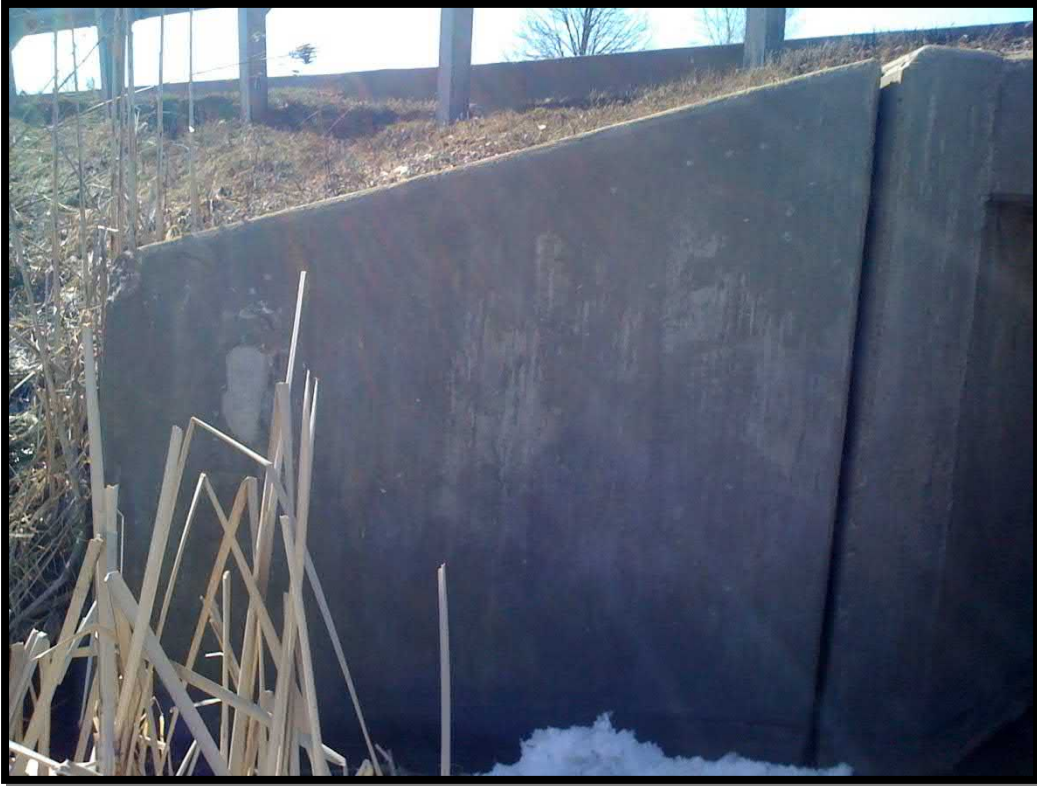
3. East end culvert face south wingwall
