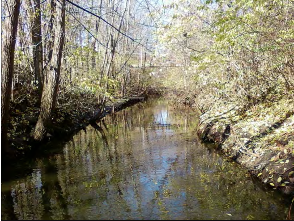
Photo 035 – 300' downstream section looking downstream (west)
