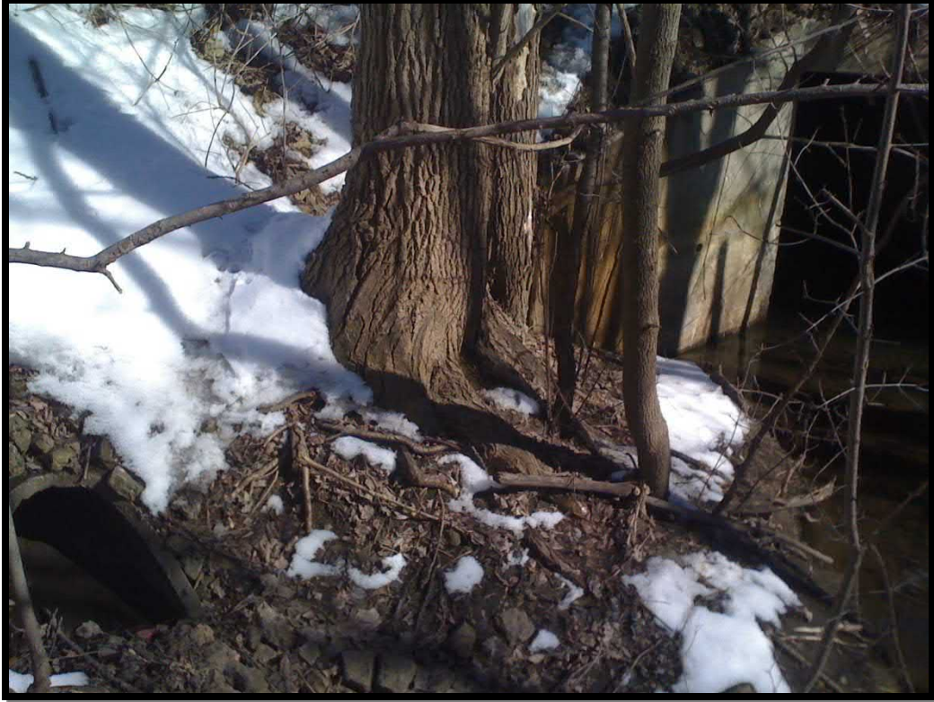
11. Northwest wingwall and nearby drainage culvert
