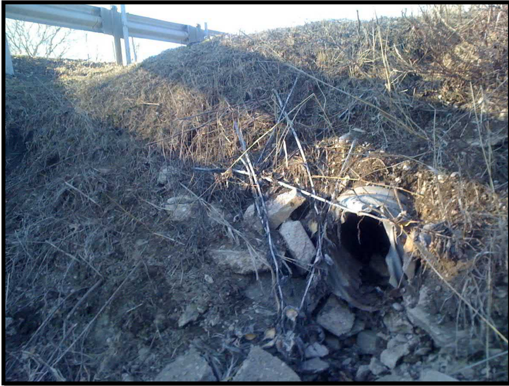
7. 1'-6"-diameter corrugated metal drain pipe outside east end of culvert
