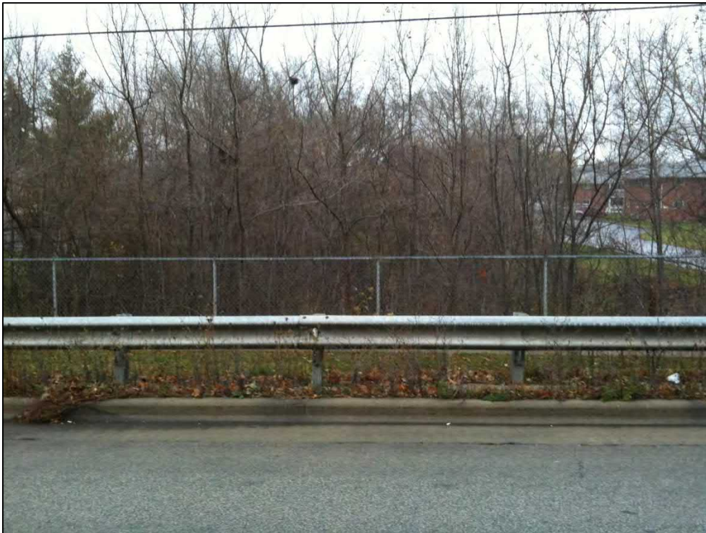
Photo 49 – Standing above culvert on IL 47 looking east (upstream)
