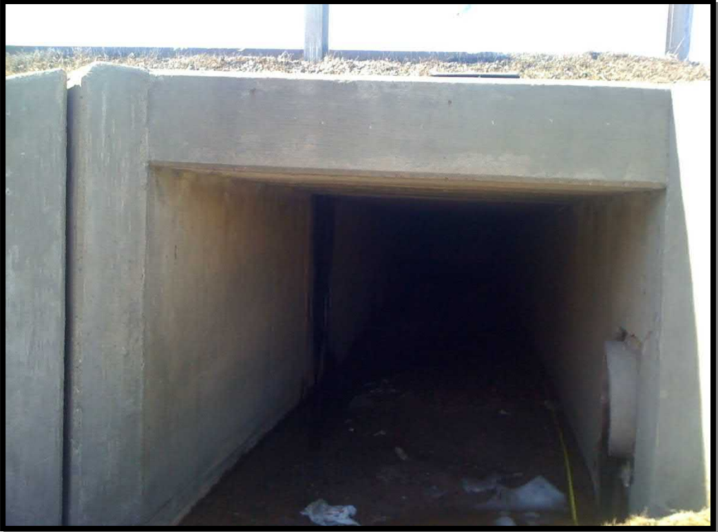
2. East end culvert face
