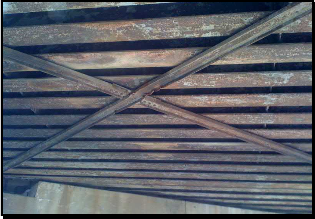
Photograph 3. Cross bracing fixed to bottom of steel floor stringers
