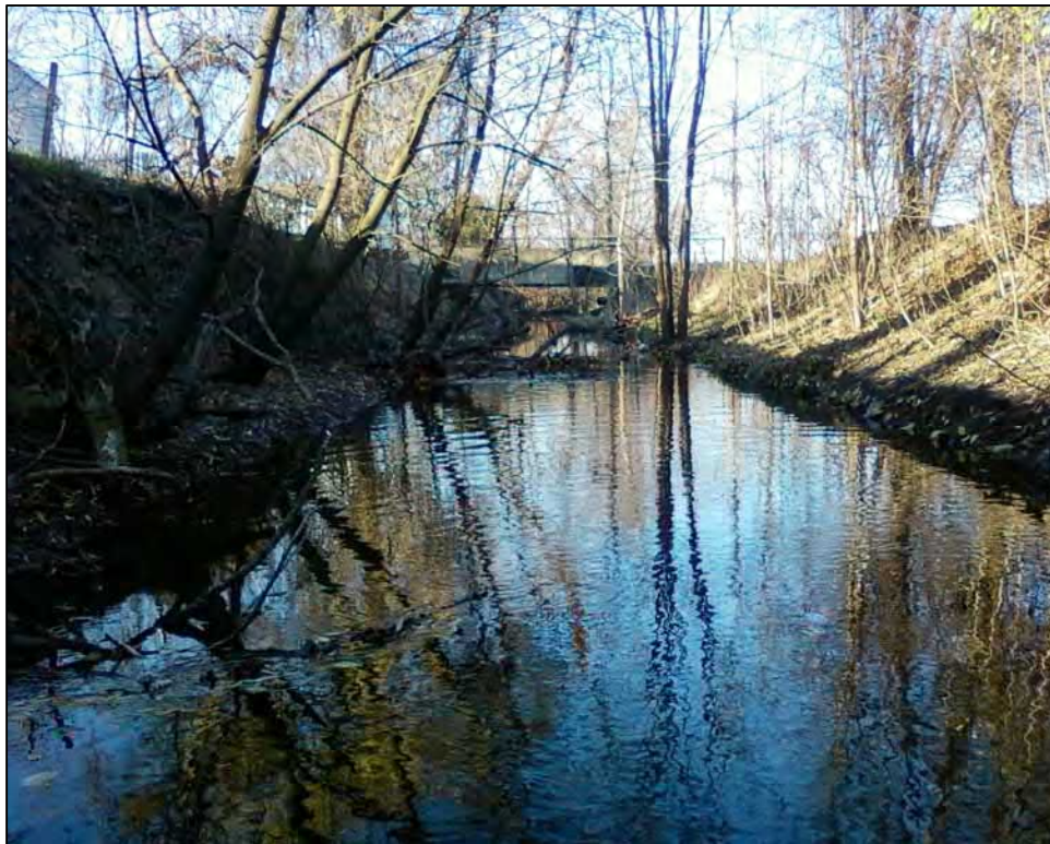
Photo 043 – 1000' downstream section looking downstream (west)
