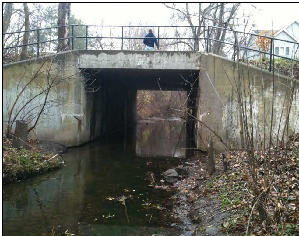
Photo 45 – Looking downstream (north) at upstream face of St. Johns Rd. Culvert
