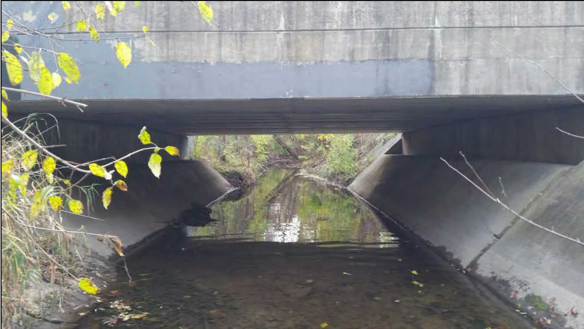
050S – 1210' downstream section looking south (upstream) at Melody Lane Bridge
