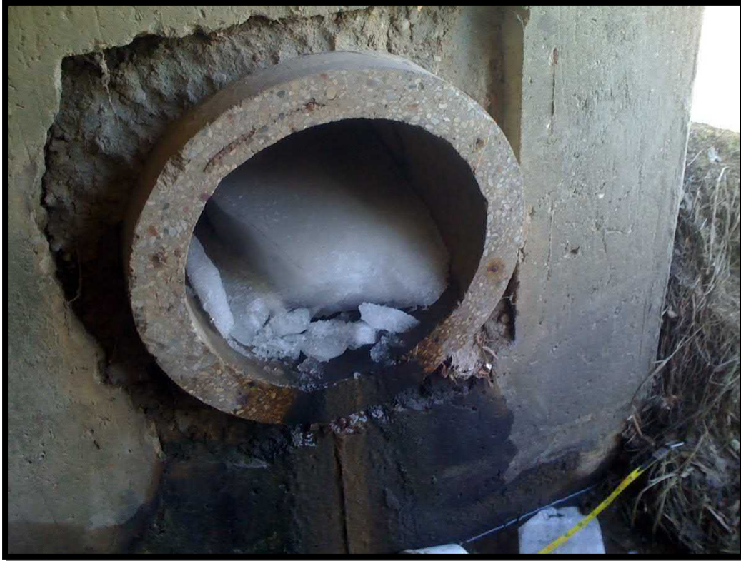
5. Inlet drain 2'-0" into the east side of the culvert
