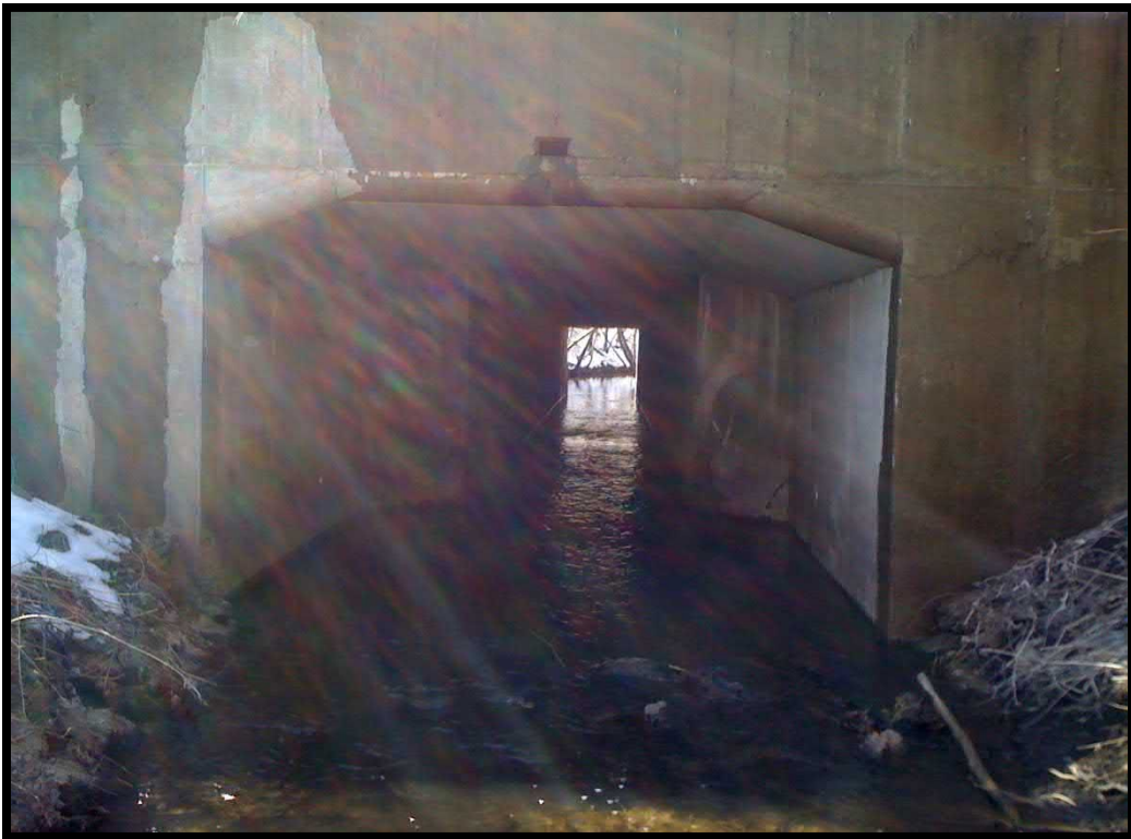
2. East end of culvert looking west into barrel
