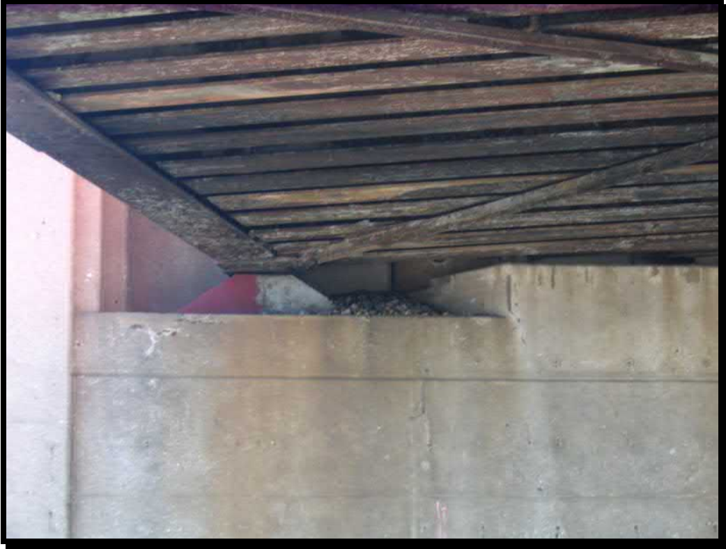
Photo 47. West Abutment-South bearing seat
