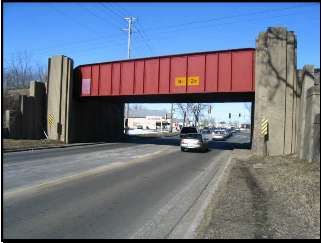
Photograph 1. Union Pacific Railroad Bridge looking north
