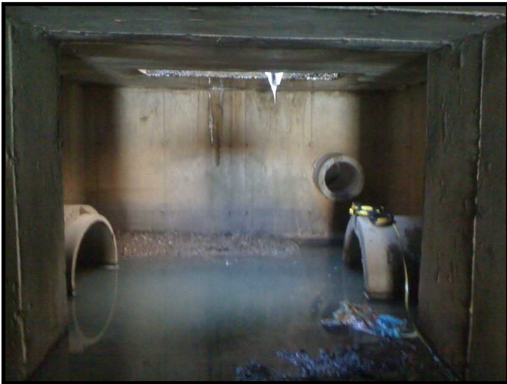
6. Storm sewer and inlet pipe at west end box of culvert
