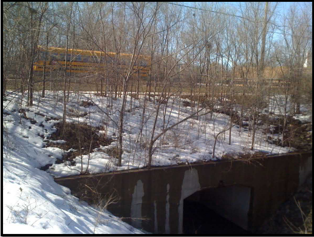
3. East end of culvert looking west at IL Route 47
