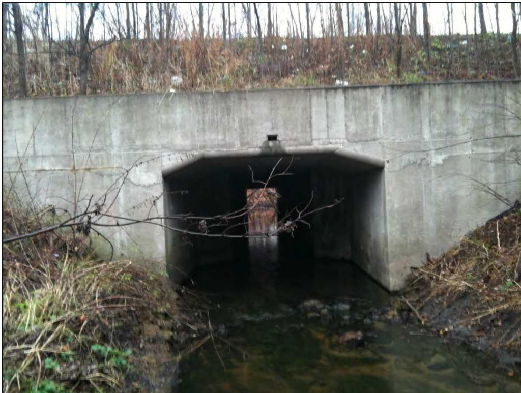
Photo 46 – Looking downstream (west) at the upstream face of IL 47 Culvert
