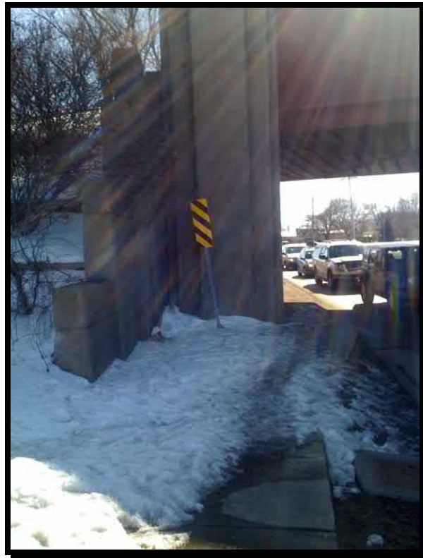
Photograph 4. Stepped wingwall, typical at each corner of the bridge
