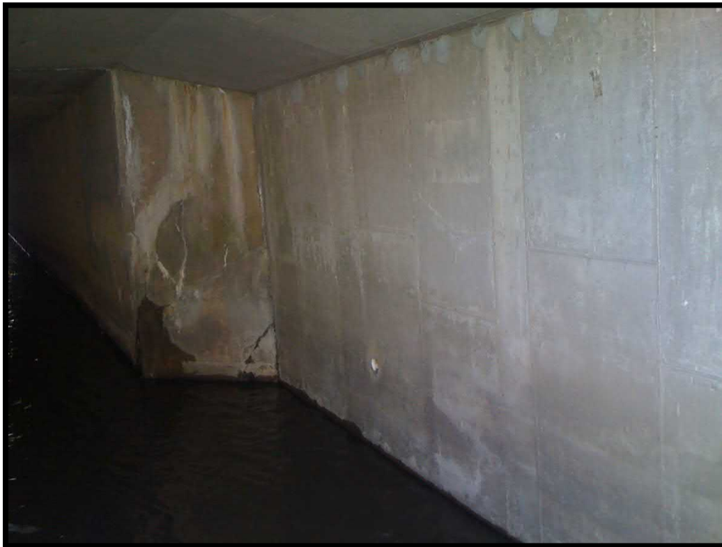
16. East end entrance of culvert looking north
