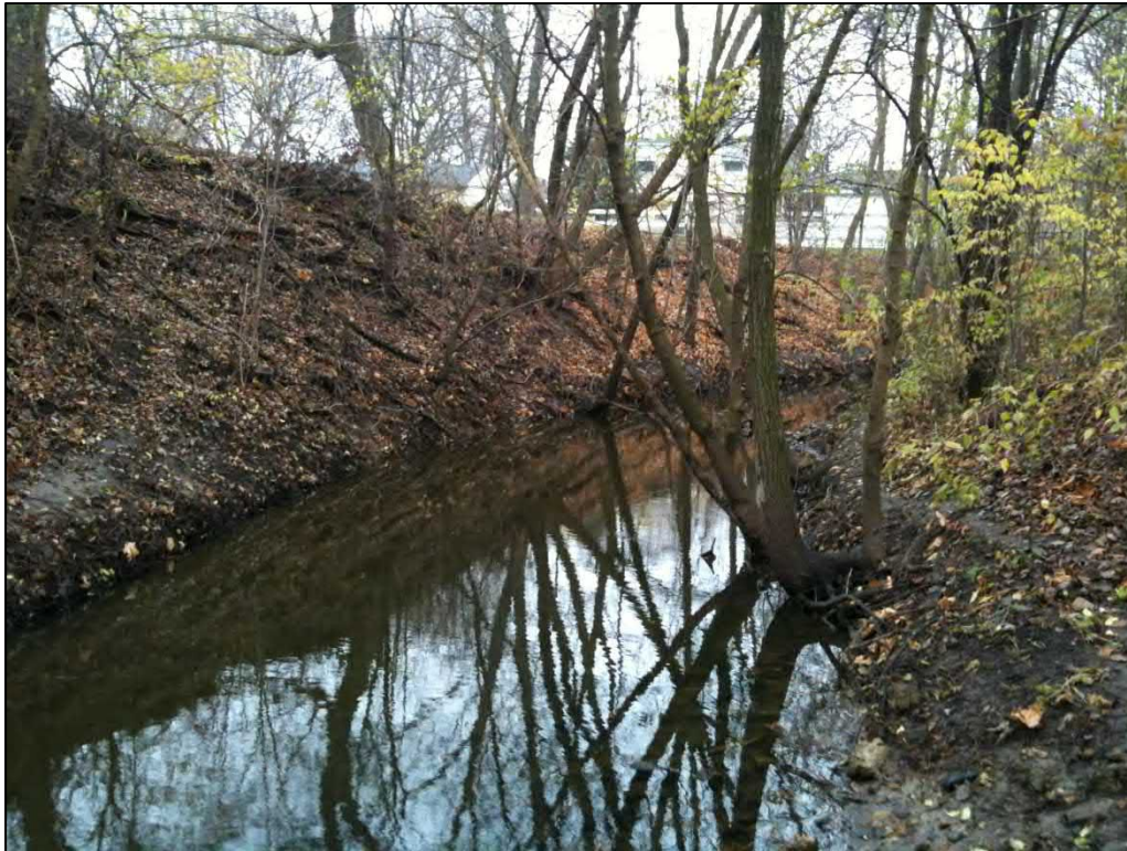
Photo 52 – Standing at downstream face of IL 47 Culvert looking downstream (west)
