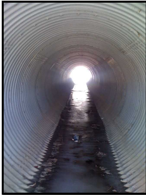
Photograph 7. Interior of south pipe culvert barrel
