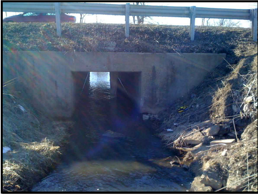
1. East end of culvert looking west
