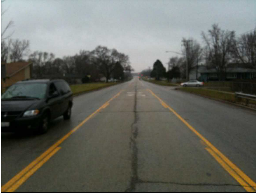
Photo 48 – Standing above culvert on IL 47 looking north
