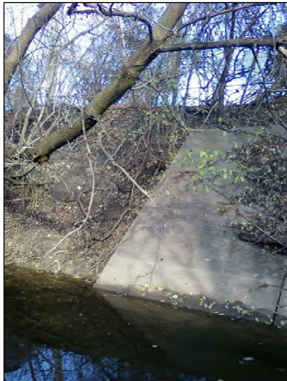
Photo 028 – 500' upstream section looking north
