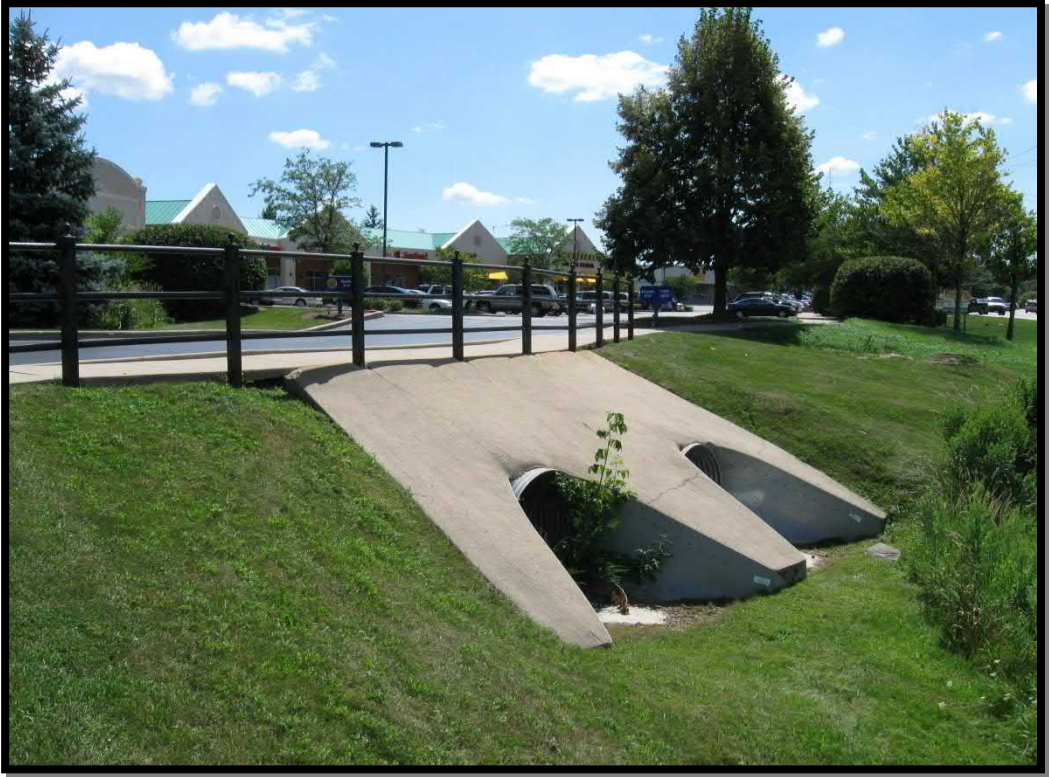
Photograph 1. West end of culvert looking south
