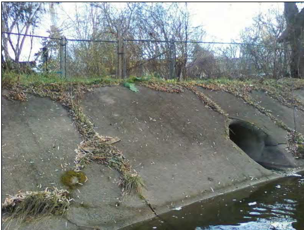
Photo 024 – 600' upstream section looking east
