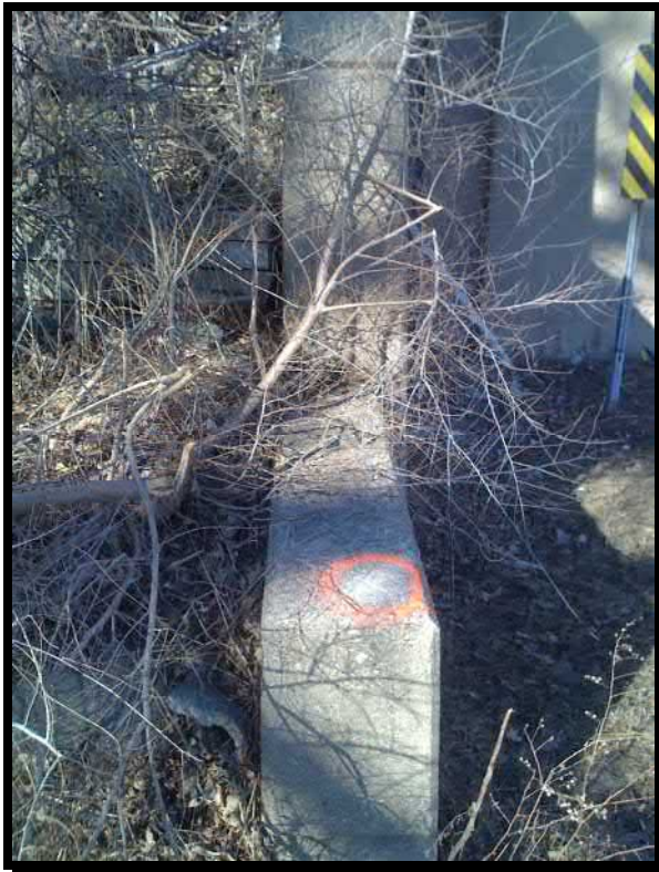
Photograph 42. Benchmark on southwest wingwall
