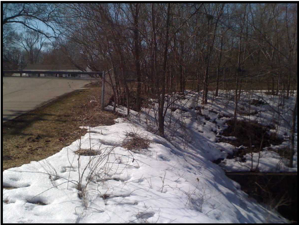
4. East end of culvert looking south
