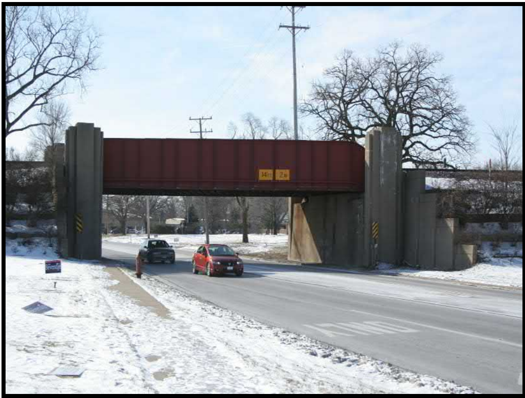
Photograph 2. Union Pacific Railroad Bridge looking south
