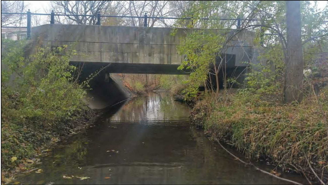
140N – 1120' downstream looking north (downstream) at Melody Lane Bridge
