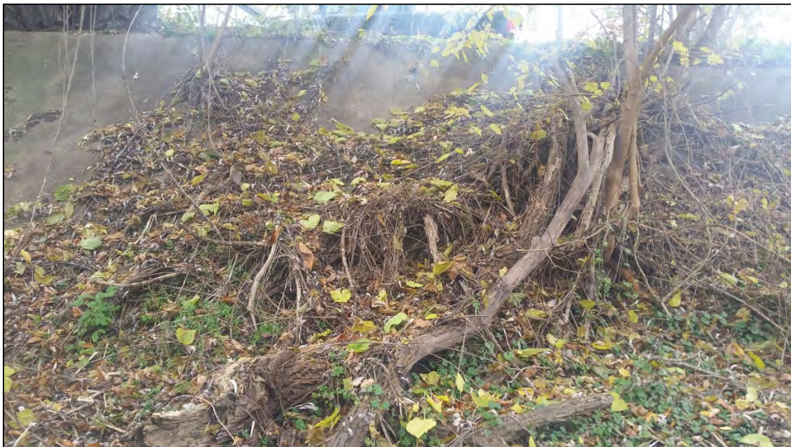
140W – 1120' downstream looking west
