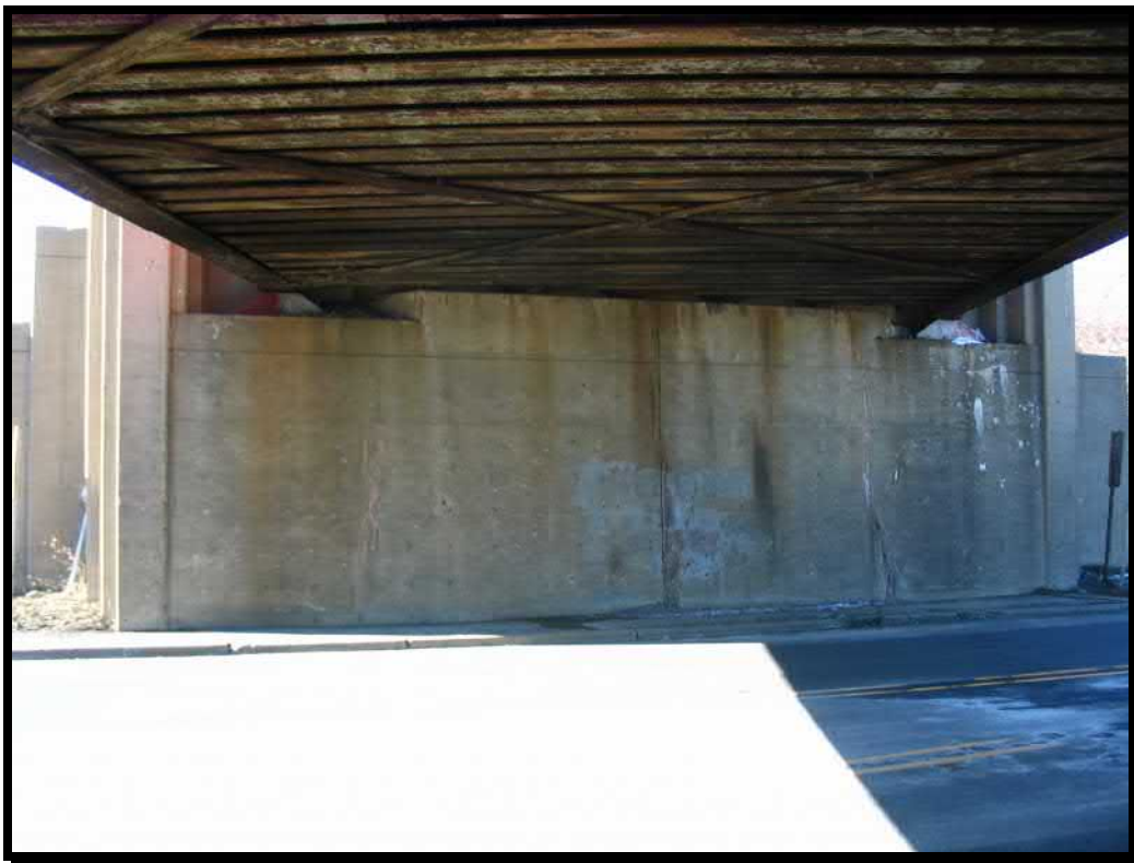
Photo 46. West abutment face
