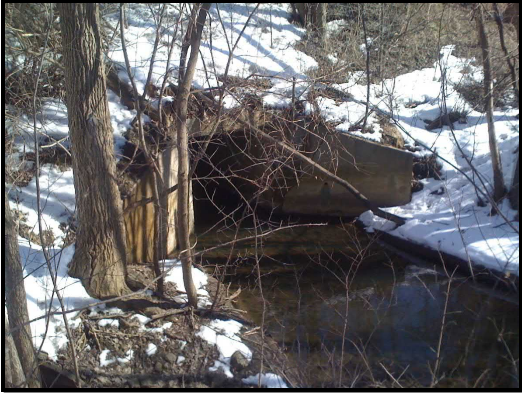
9. West end of culvert with wingwalls
