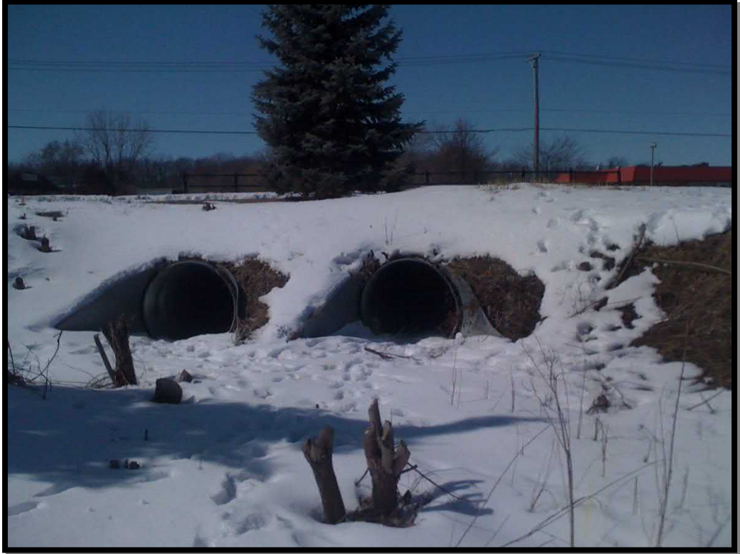
Photograph 4. East end of culvert looking west
