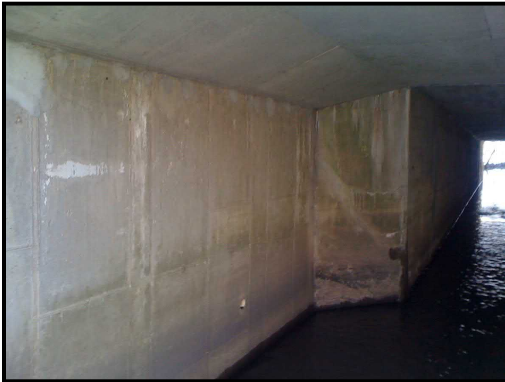
14. East end entrance of culvert looking south
