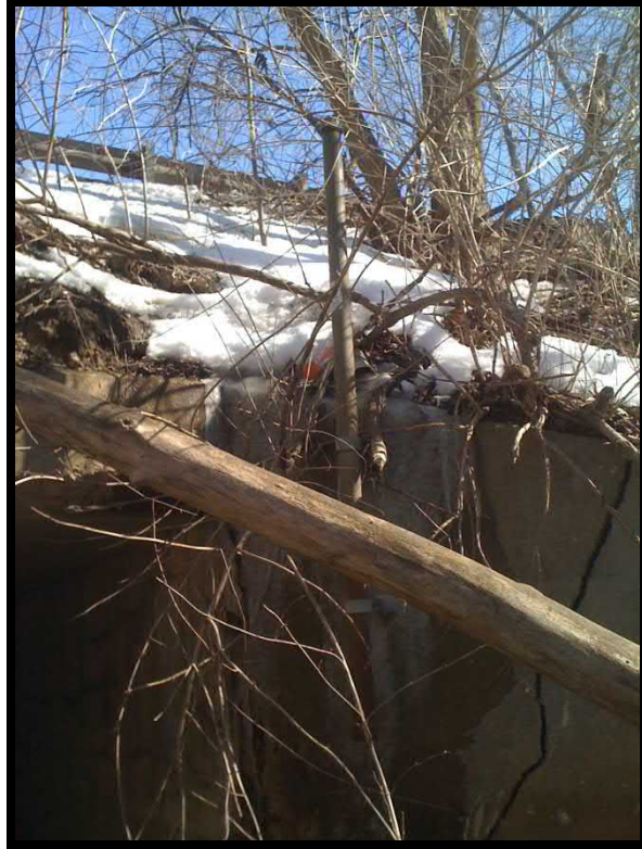
13. Water level gauge on structure's southwest wingwall
