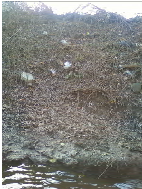
Photo 030 – 500' upstream section looking south
