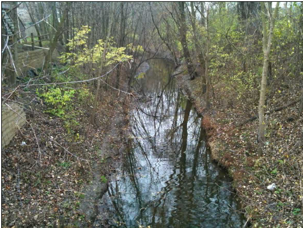
Photo 44 – Standing at upstream face of St. Johns Rd. Culvert looking upstream (south)
