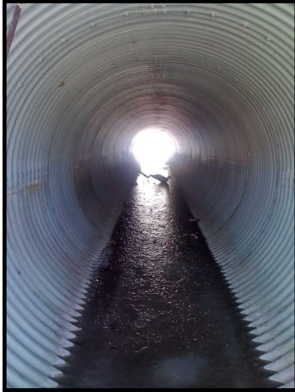
Photograph 6. Interior of north pipe culvert barrel
