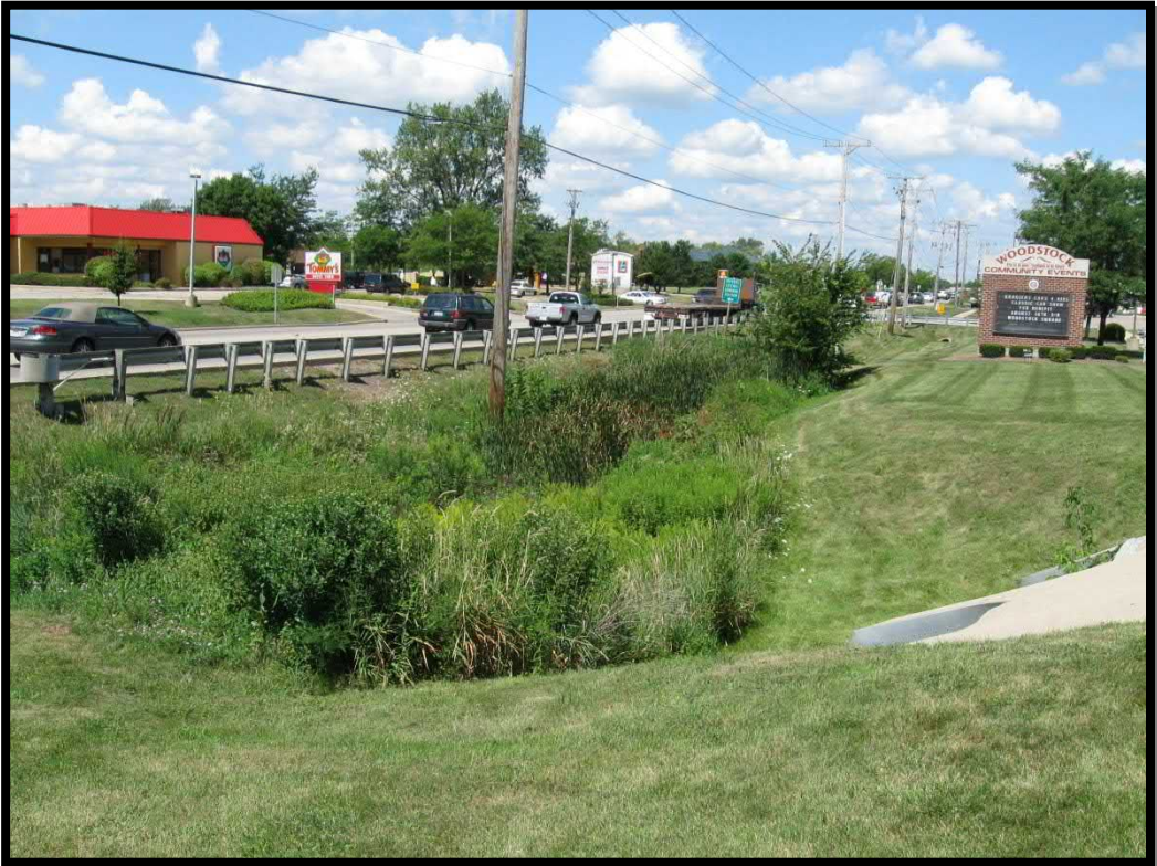
Photograph 3. West end of culvert looking north
