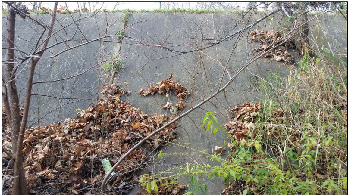
050W – 1210' downstream section looking west
