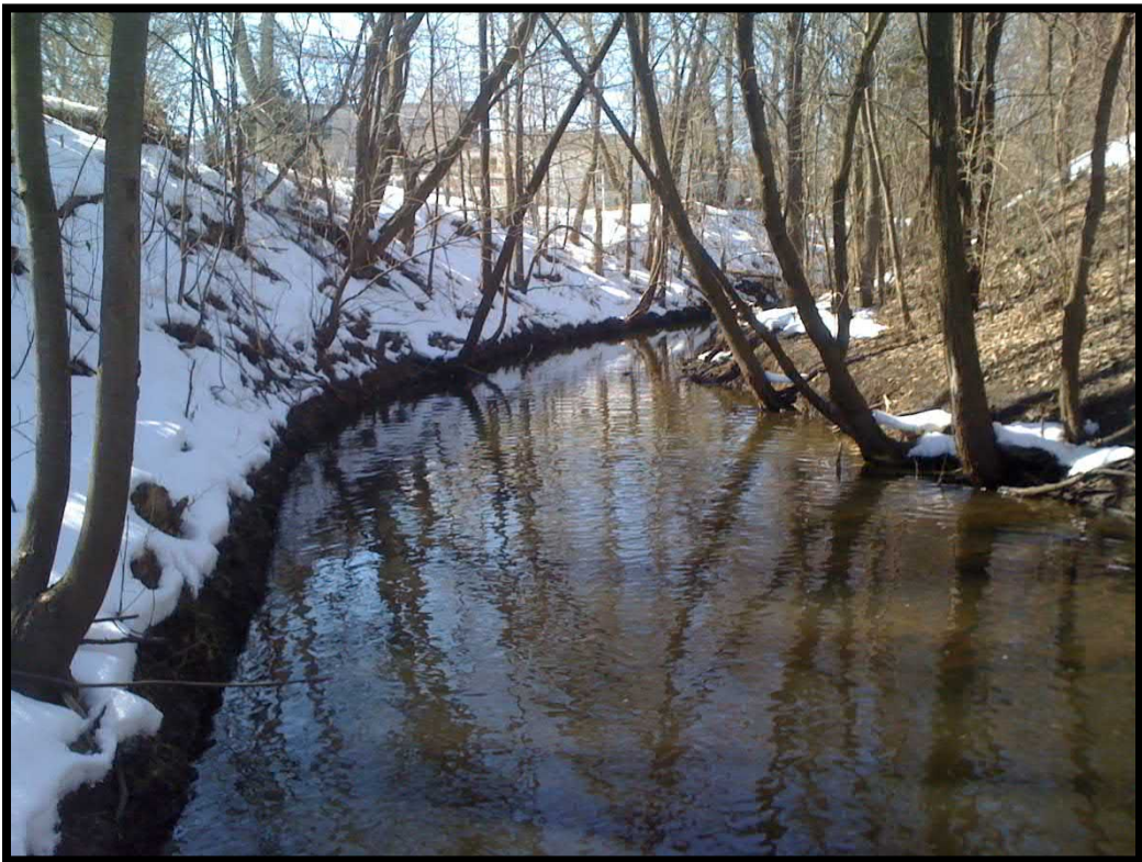
10. West end of culvert looking west (upstream)
