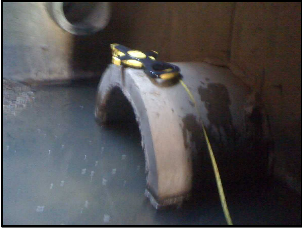
7. North facing outlet pipe in west end of culvert
