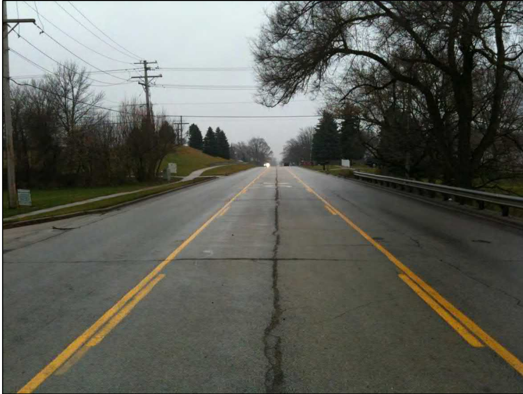
Photo 50 – Standing above culvert on IL 47 looking south
