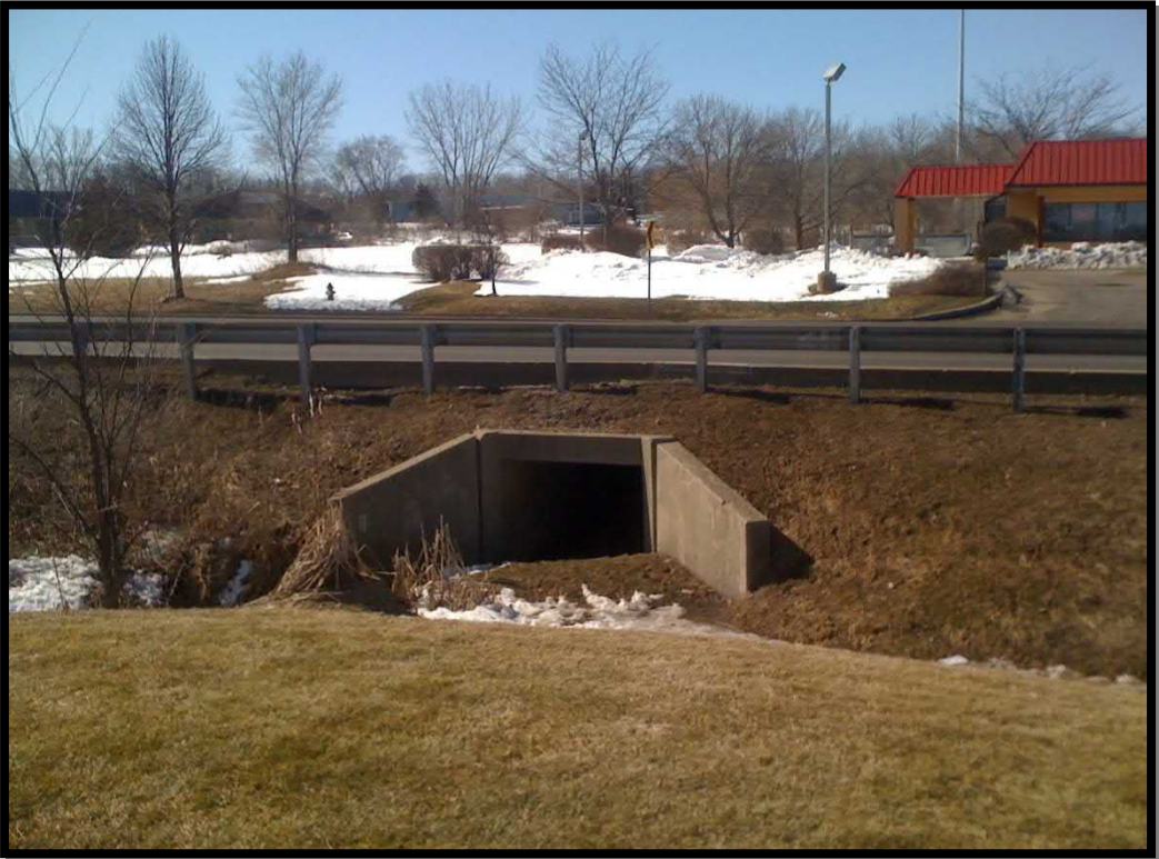
1. Culvert location on east side of IL Route 47
