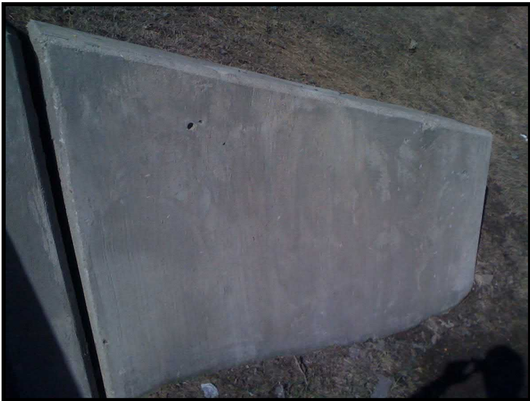
4. East end culvert face north wingwall
