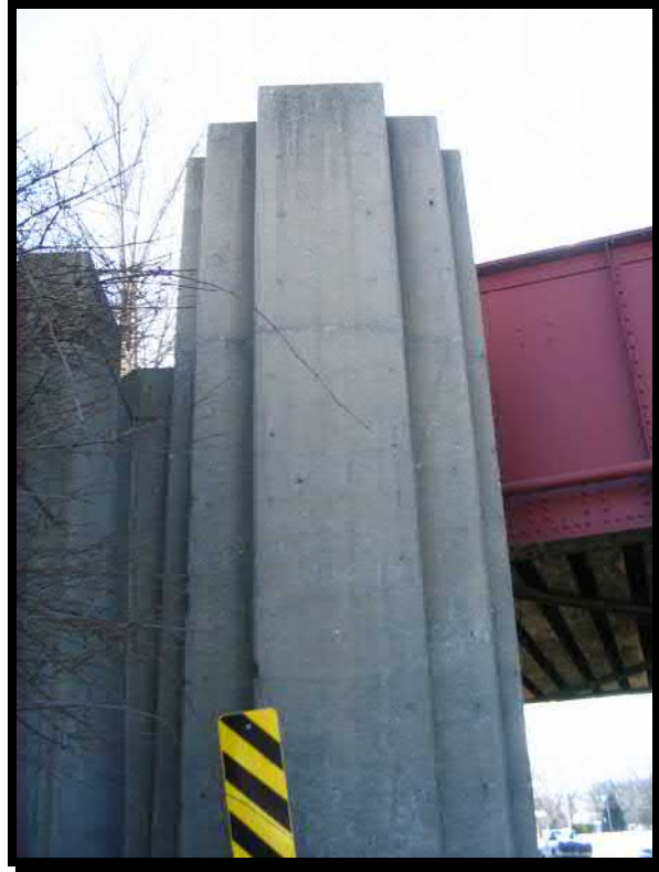
Photograph 5. Decorative column, typical at the ends of both abutments
