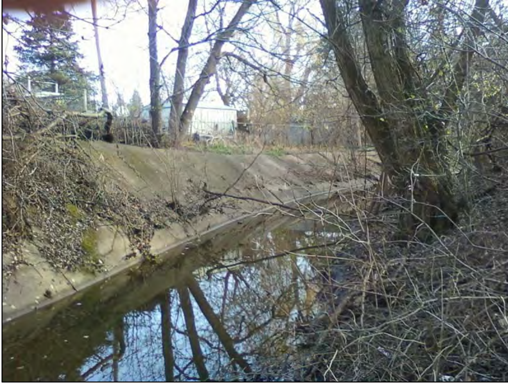
Photo 029 – 500' upstream section looking upstream (east)
