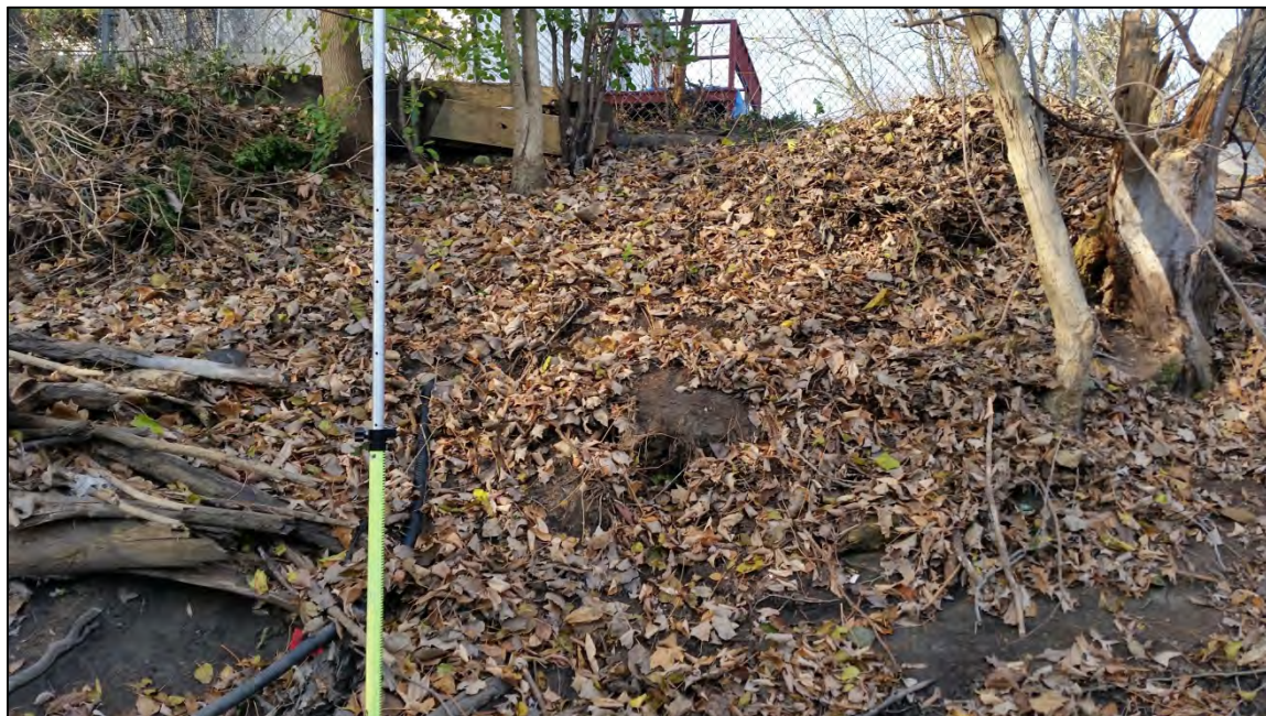
000W – 1260' downstream section looking west
