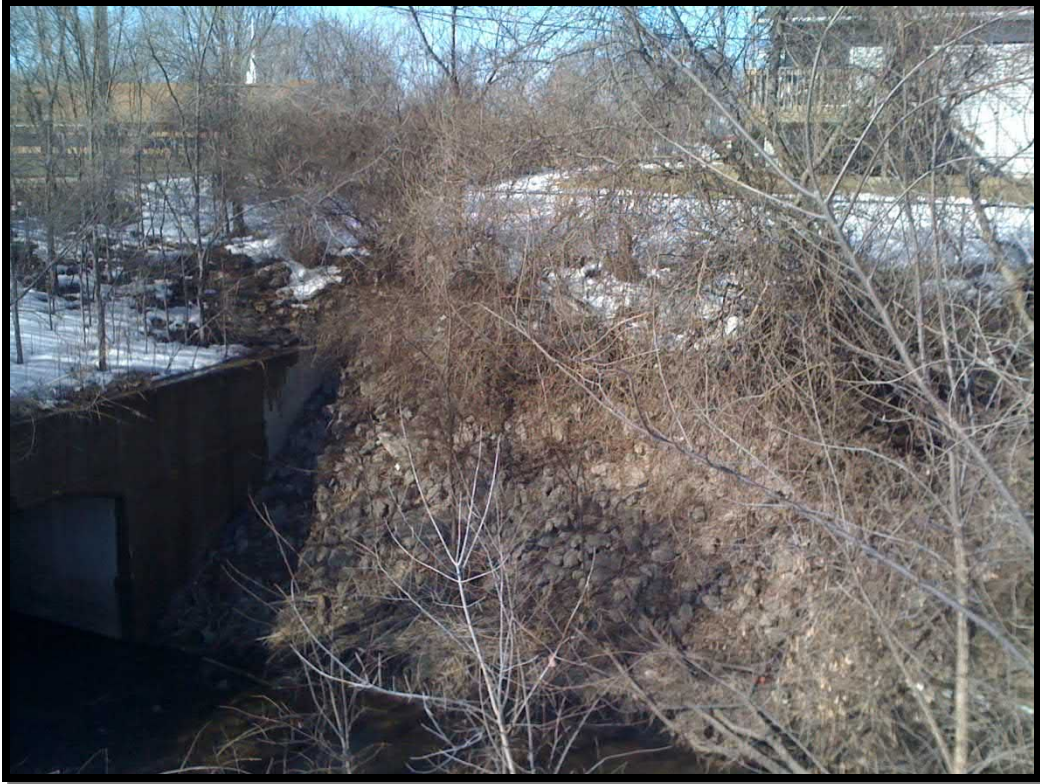
5. East end of culvert looking north
