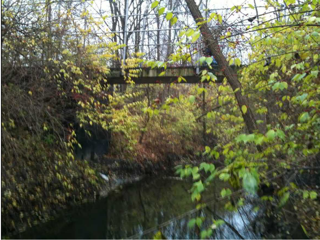
Photo 56 – Looking upstream (south) at downstream face of Pedestrian Bridge
