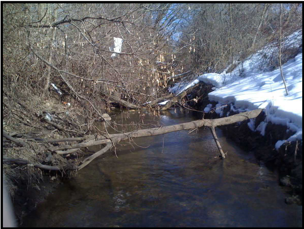
6. East end of culvert looking east (downstream)
