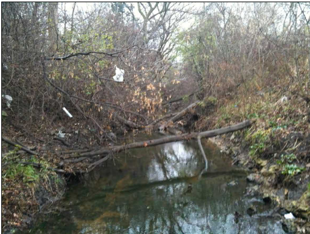
Photo 47 – Standing at the upstream face of IL 47 Culvert looking upstream (east)
