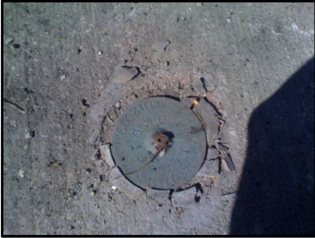
13. Benchmark on southeast wingwall
