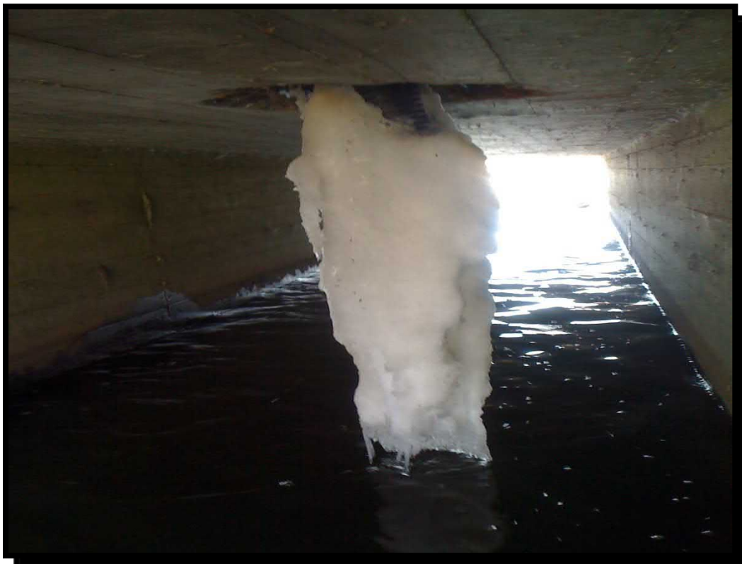
8. Hole in the top slab with exposed reinforcement and protruding drain pipe
