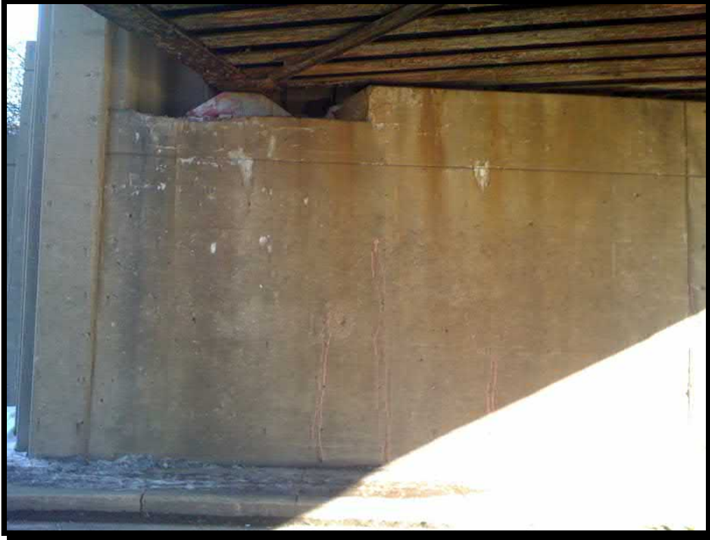
Photo 33. East Abutment Face—North Side
