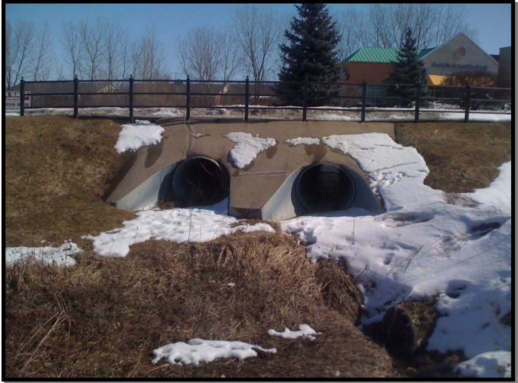
Photograph 2. West end of culvert looking east
