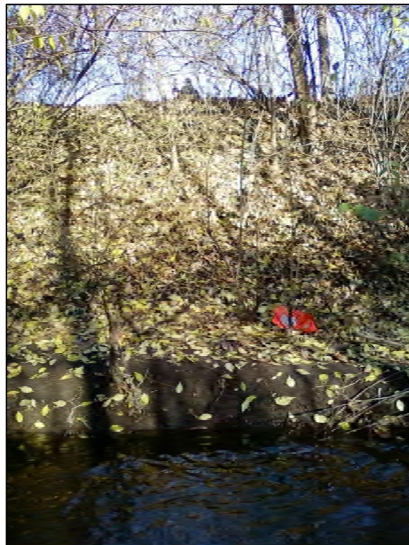
Photo 040 – 500' downstream section looking north
