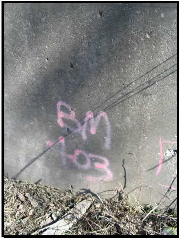
Photograph 10. Benchmark on southeast wingwall
