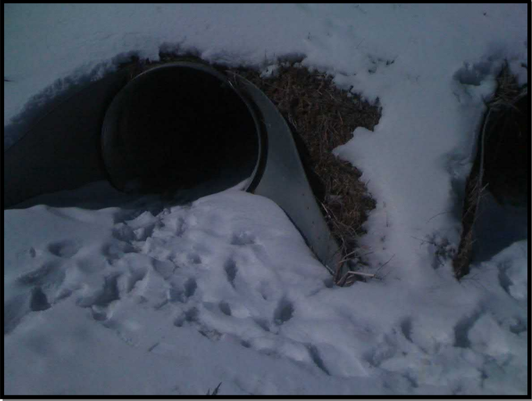
Photograph 6. South pipe at east end
