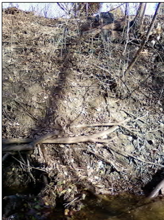
Photo 032 – 300' upstream section looking north
