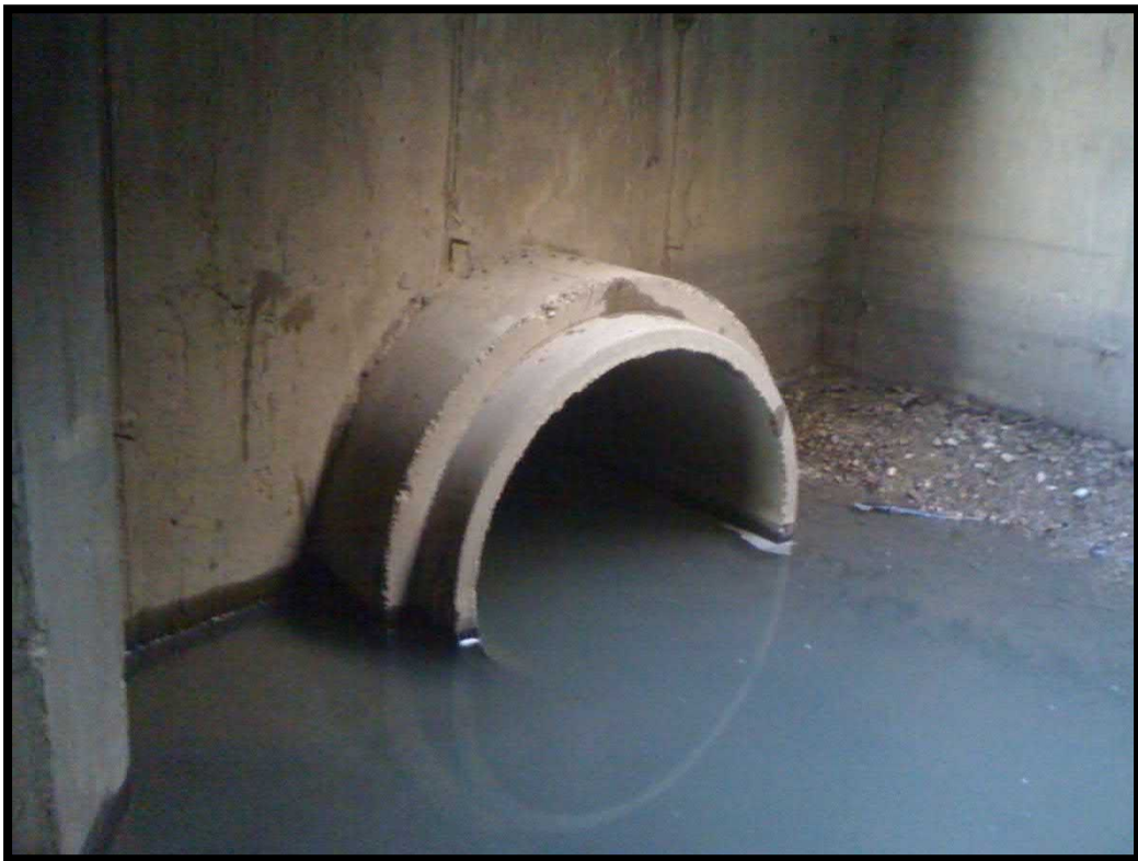
8. South facing outlet pipe in west end of culvert
