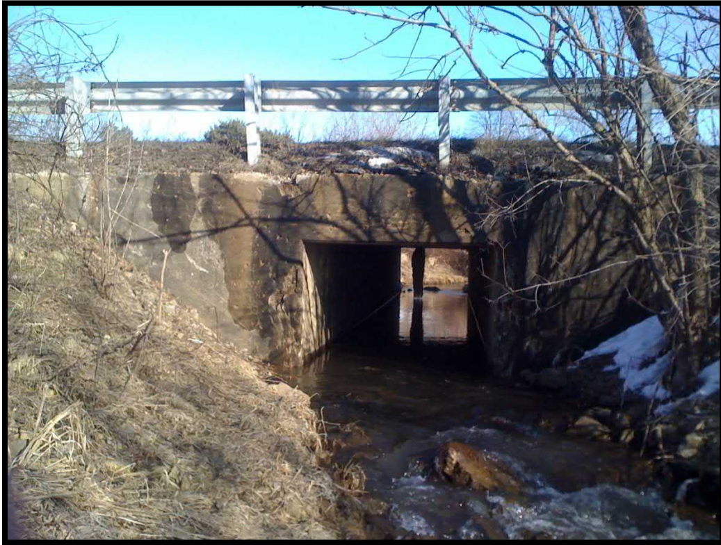
3. West end of culvert looking east
