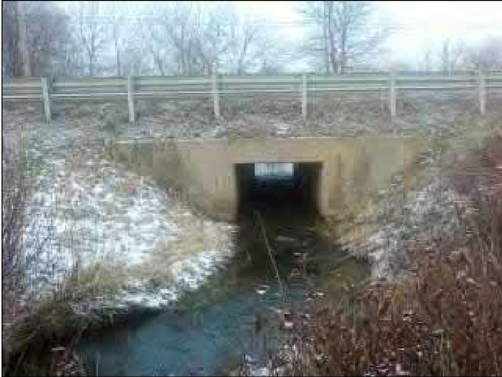
Photo 3 – Upstream face of 6' x 5' RCBC looking west
