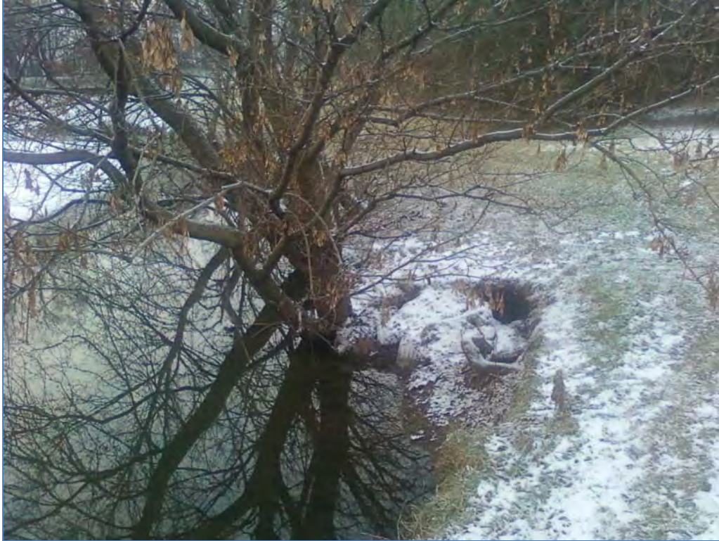
Photo 1 – Standing at northwest side of pond looking south at 2-24” CMPs
