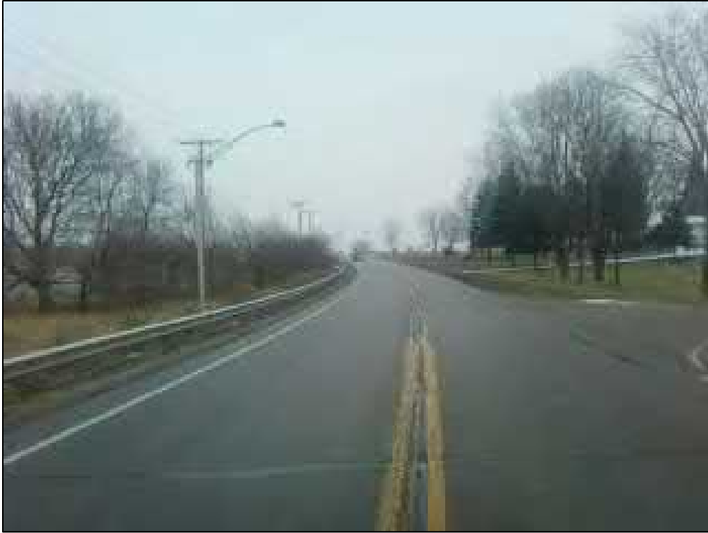
Photo 7 – Standing above culvert on IL-47 looking north
