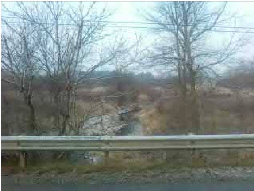
Photo 10 – Standing above culvert on IL-47 looking downstream (west)
