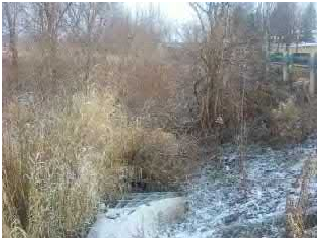
Photo 12 – Standing south of the downstream face of culvert looking north
