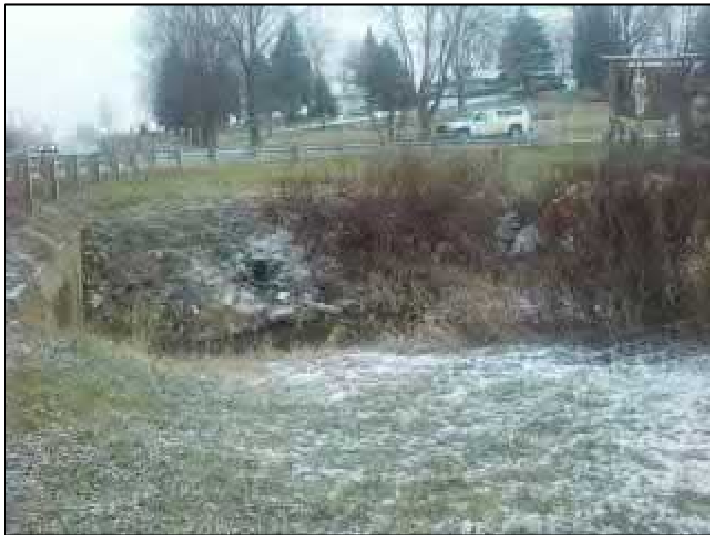
Photo 6 – Standing at upstream face of culvert looking north
