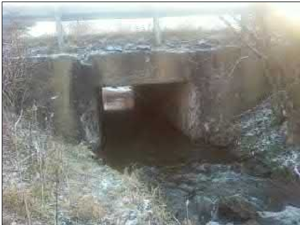
Photo 14 – Downstream face of 6' x 5' Culvert looking upstream (east)
