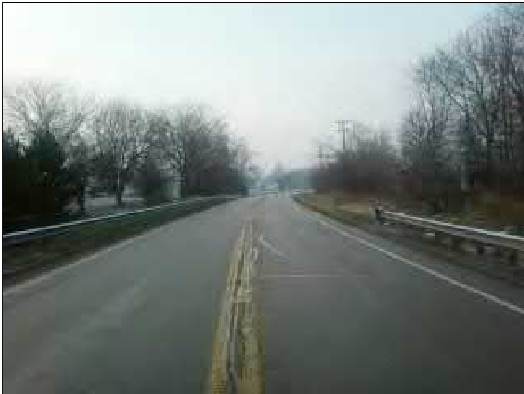
Photo 8 – Standing above culvert on IL-47 looking south
