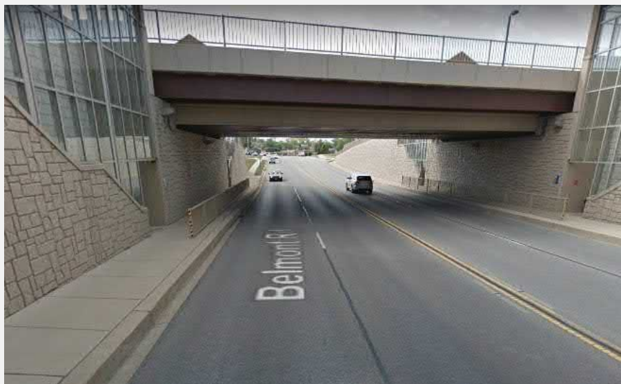
Exhibit 2 - Belmont Road railroad underpass in Downers Grove
