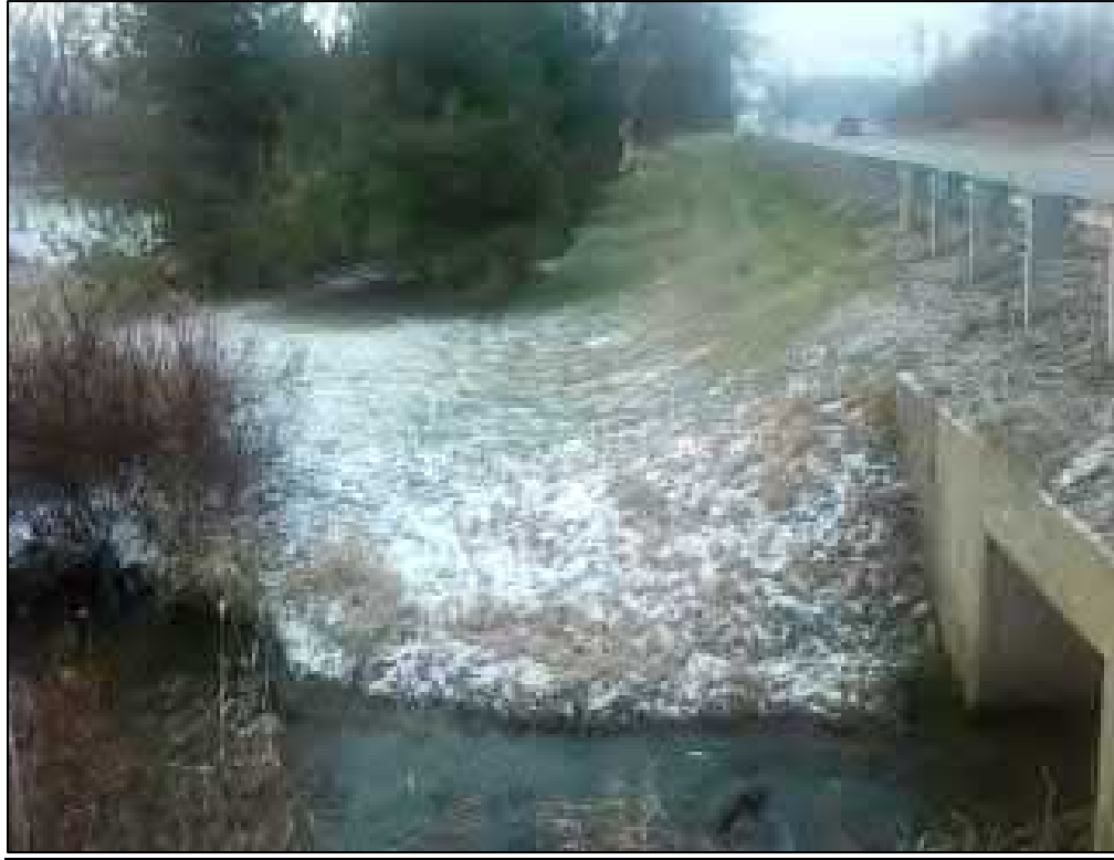
Photo 5 – Standing at upstream face of culvert looking south
