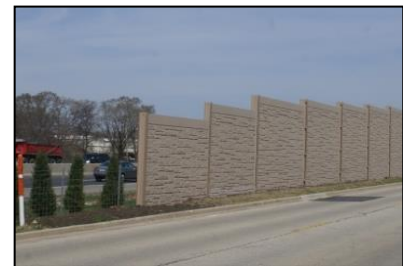
Noise Barrier (photo courtesy of IDOT)
