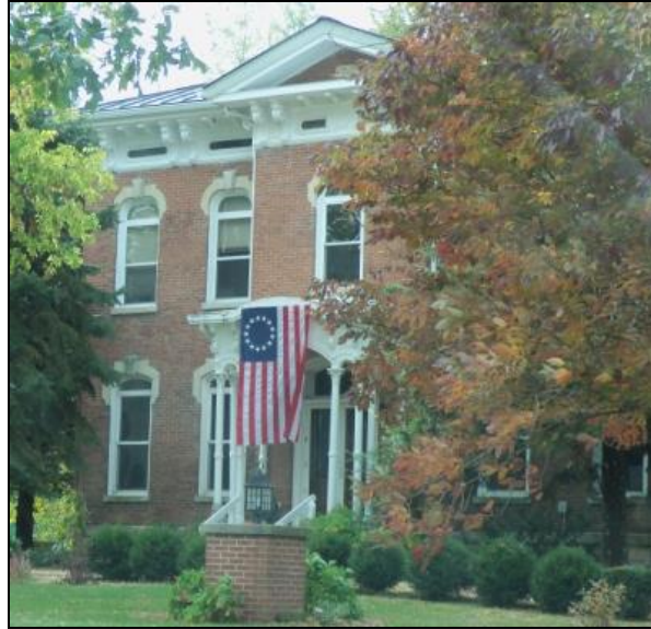
Home on 2100 East Road that may be eligible for the NRHP
