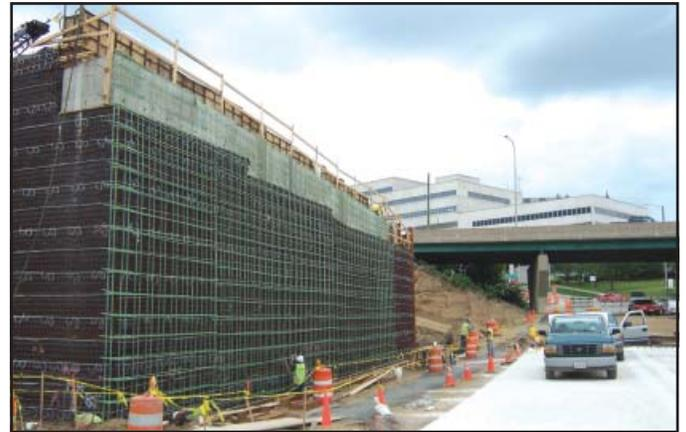
event. Alternatives to using the precast panels are a welded wire mesh material that extends the entire height and length of the wall or a cast-in-place wall facing. Generally, the wire mesh option is used for walls that will not be visible to motorists and do not require an aesthetically pleasing appearance.
