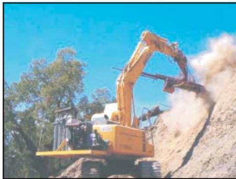
then collapses onto the bar, creating a powerful bond. Tests show this bond to be much greater than with percussion-driven nails. Pull-out tests indicate bond strength can be
