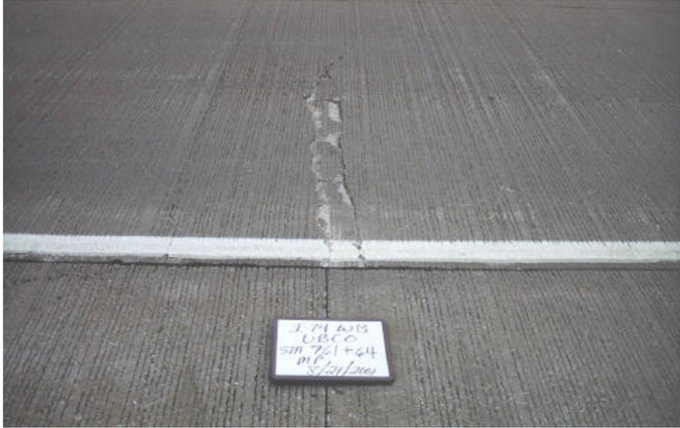
Figure 1. Early Stage of Punchout in Unbonded Concrete Overlay in 2001.
