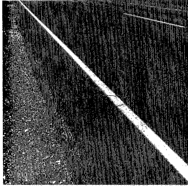
Photo 1. A typical longitudinal crack along the pavement-shoulder joint. The present resurfacing is the first resurfacing over the old PCC pavement.
