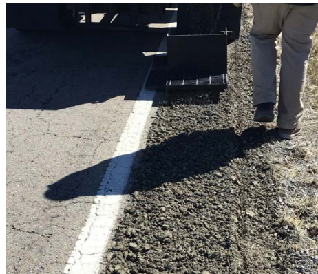
The spreader efficiently and consistently places aggregate with minimal waste.
