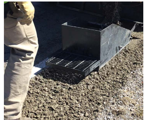
Quality aggregate shoulders eliminate dangerous drop-offs and improve motorist safety.
