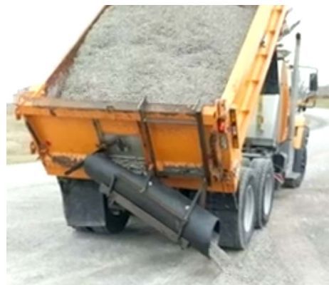
The chute releases gravel approximately 6-12 inches from the pavement edge.
