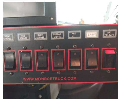
A switch inside the cab allows the operator to divert the brine to spray the white line without exiting the vehicle.
