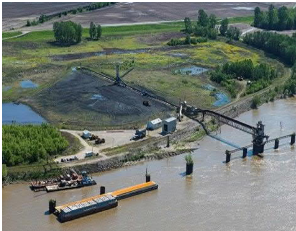
FIGURE 4-10: KELLOGG DOCK COAL TRANSLOAD
