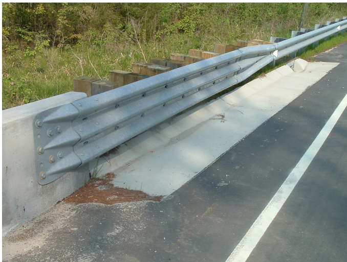
A single-faced Thrie-beam guardrail (left) joined with a W-beam guardrail.
