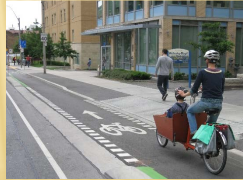
raised bike lane
